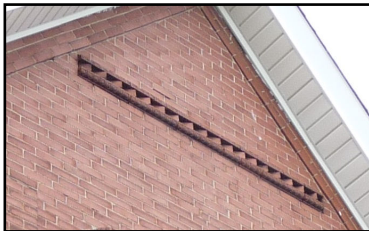
Figure 21: projecting dog-tooth course detail, September 2016
