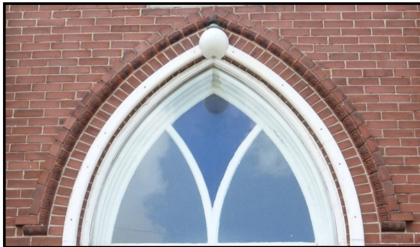
Figure 19: Hood mould detail, September 2016
