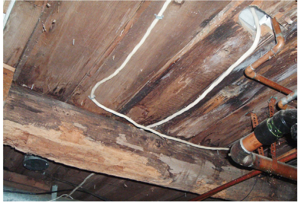
The basement appears to have had some issues with moisture and plumbing leaks.
