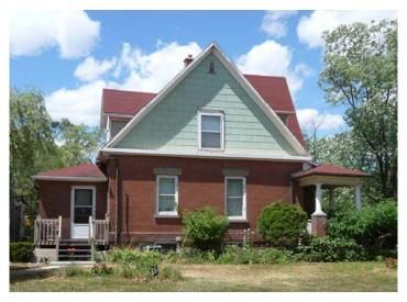
Windows are a mixture of historic wood sash, fixed and modern replacements; most have had aluminum storms placed on the exterior. All main floor windows have a cast lintel and sill and the basement windows have brick voussoirs.
