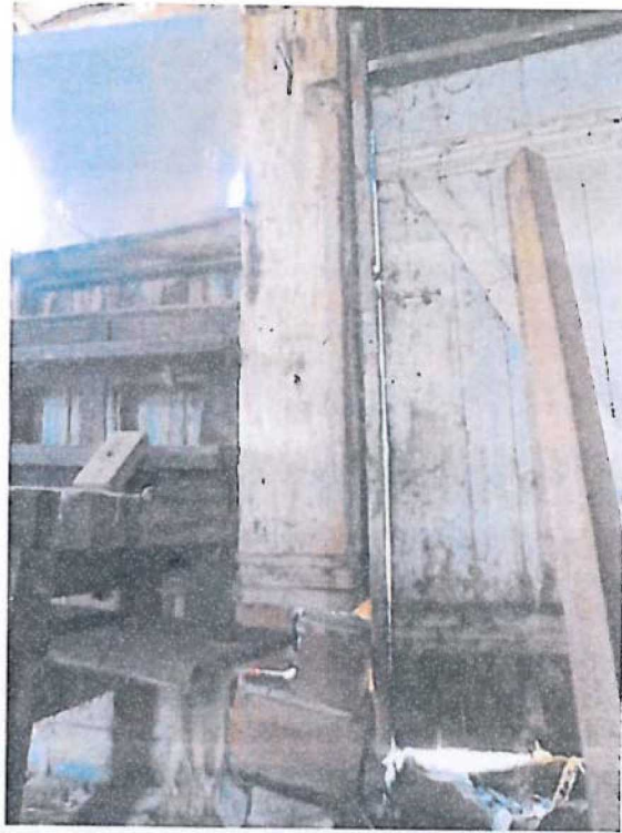
Picture 11: Damaged Foundation Wall at Column
