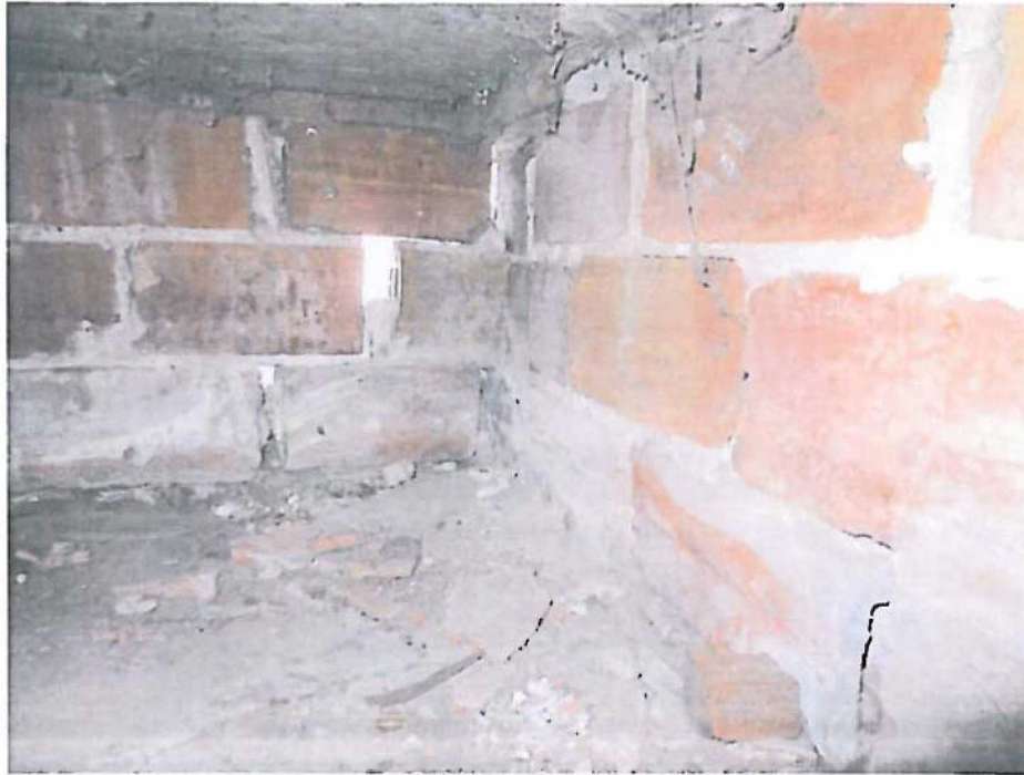
Picture 12: Damaged Foundation Wall at Corner Column
