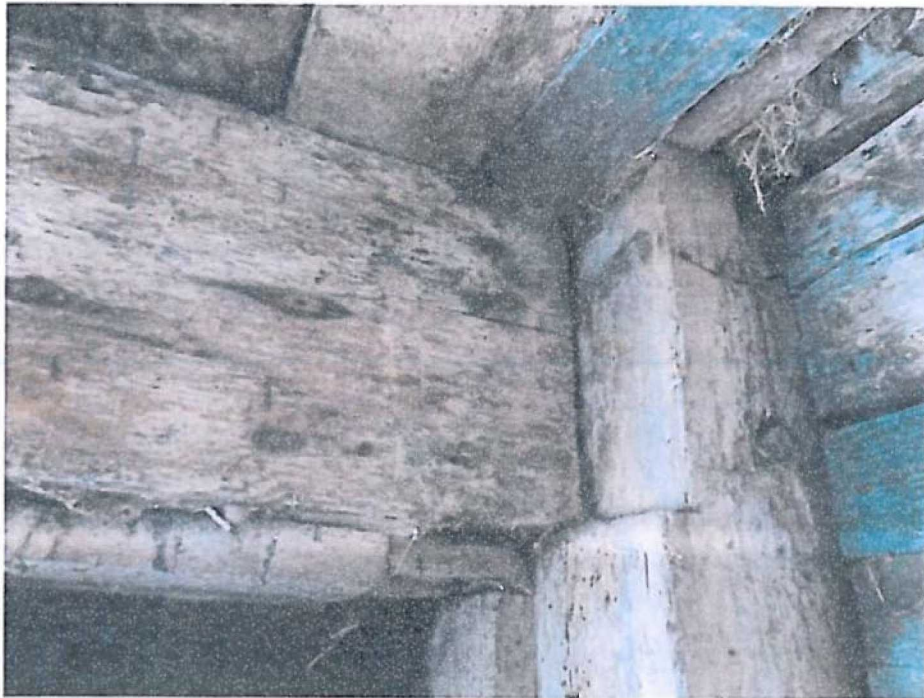
Picture 8: Improper Beam Bearing
