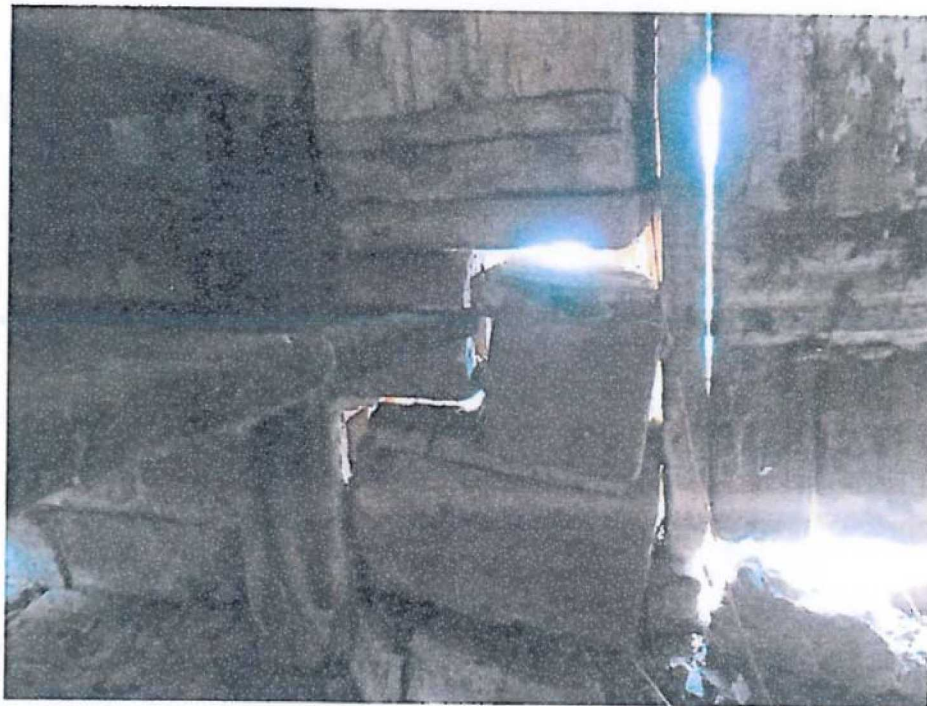
Picture 12: Damaged Foundation Wall at Column
