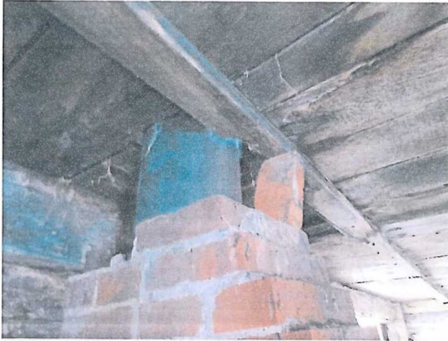
Picture 7: Floor Opening Improperly Re-Supported
