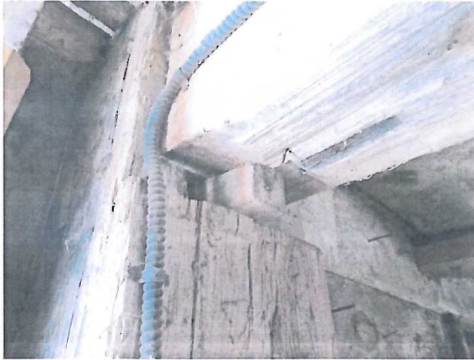
Picture 9: Improper Beam Bearing
