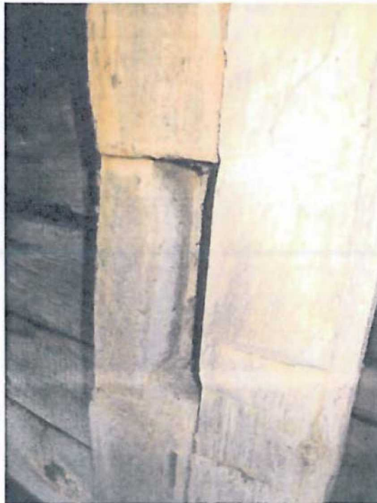
Picture 10: Hole in Column
