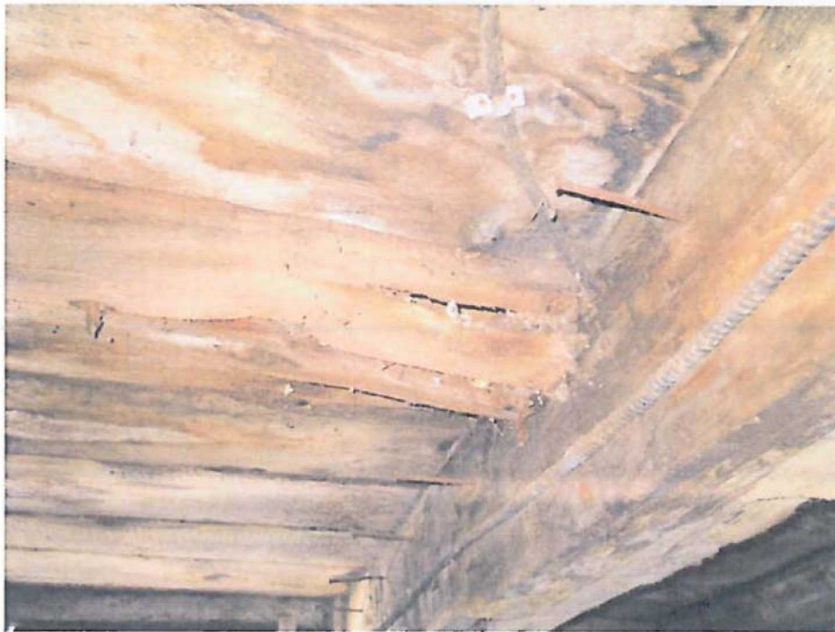
Picture 6: Damaged Floor Planks
