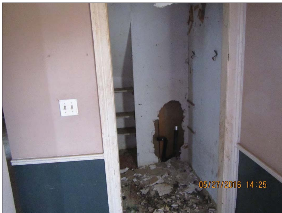
Figure 24: Plaster damage where services were removed.
