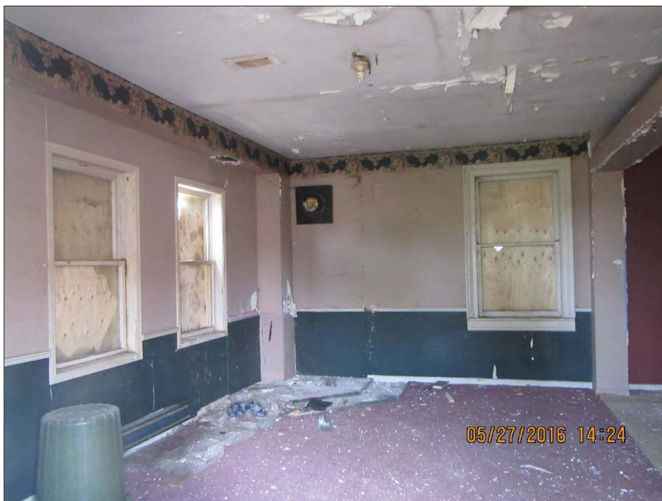
Figure 23: Interior view showing peeling paint and broken window glass.
