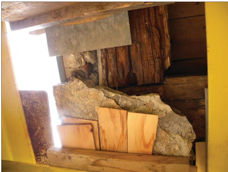
Figure 21: Rot in the end section of the sill plate
