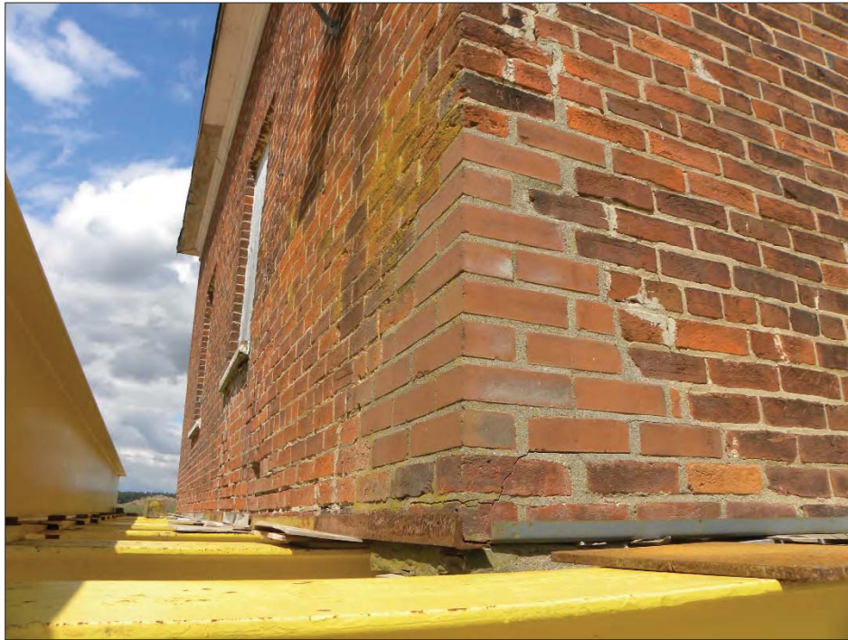
Figure 20: Masonry repair in new brick and Portland cement at the northeast corner. Missing brick and cracks can also be seen.
