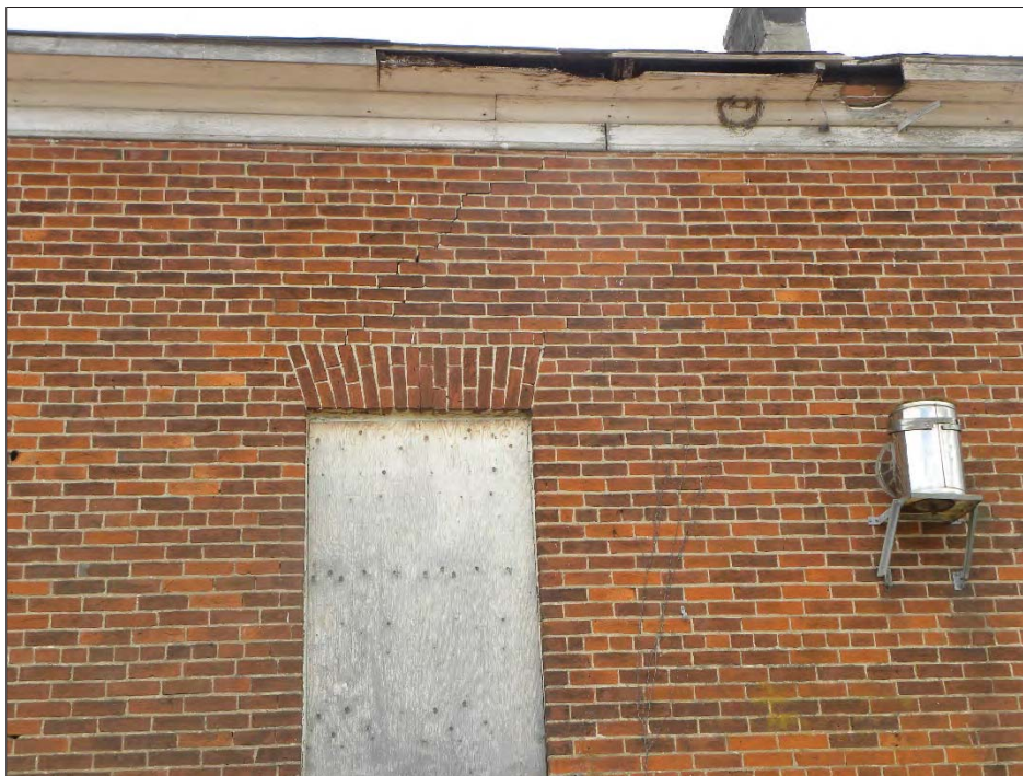
Figure 18: Section of missing fascia, soffit, and bedmould near the northeast corner. A crack in the masonry can also be seen.
