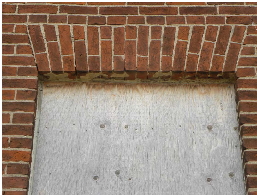
Figure 8: Details of the voussoir over the ground floor windows.
