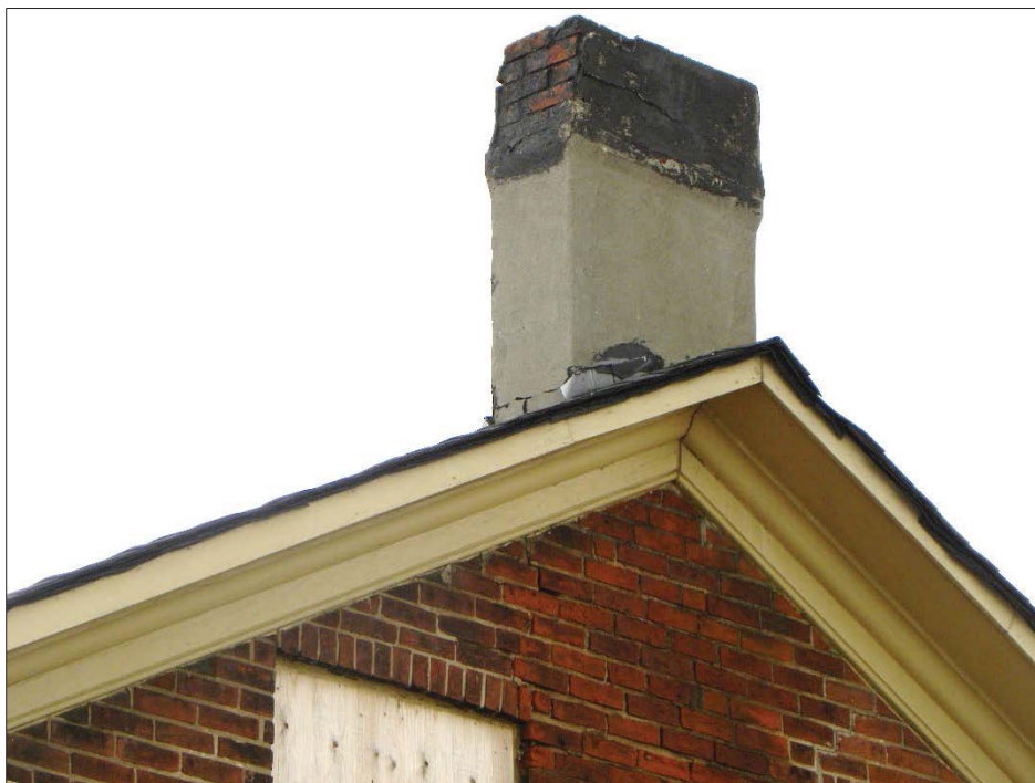
Figure 19: Lifted or missing flashing and mortar loss on the south chimney.
