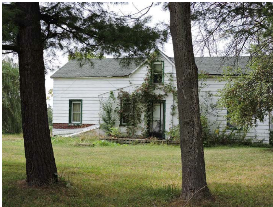
Figure 7: Façade of Ford-Slacer farmhouse with exposed red brick, showing treeline (AB, 2015)
