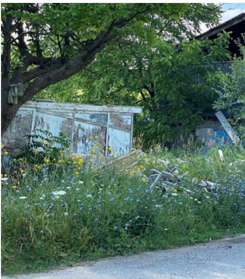
Wood shed structure.
