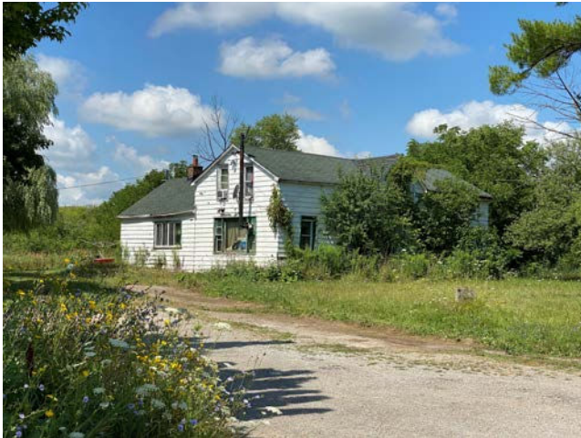
Front and side (northeast) elevations of house.
