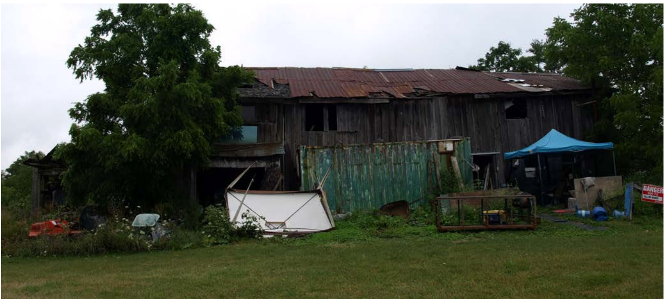
Side (southeast) elevation of the barn.
