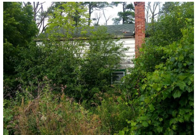
Partial rear (southwest) elevation of house.
