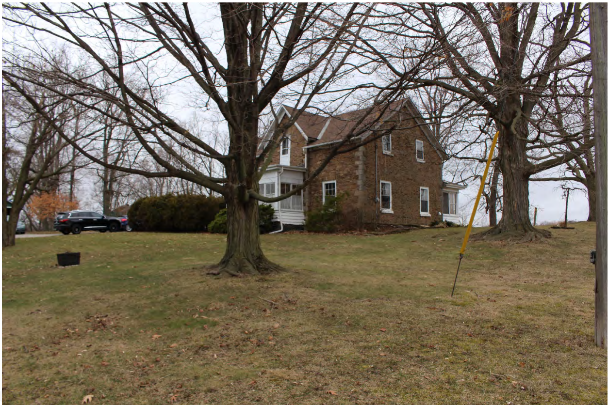
Figure 1: View of 2031 North Service Road West from near North Service Road, looking west (ML 2020).
