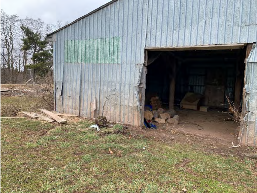
Figure 11: 1980s outbuilding (CU 2020).
