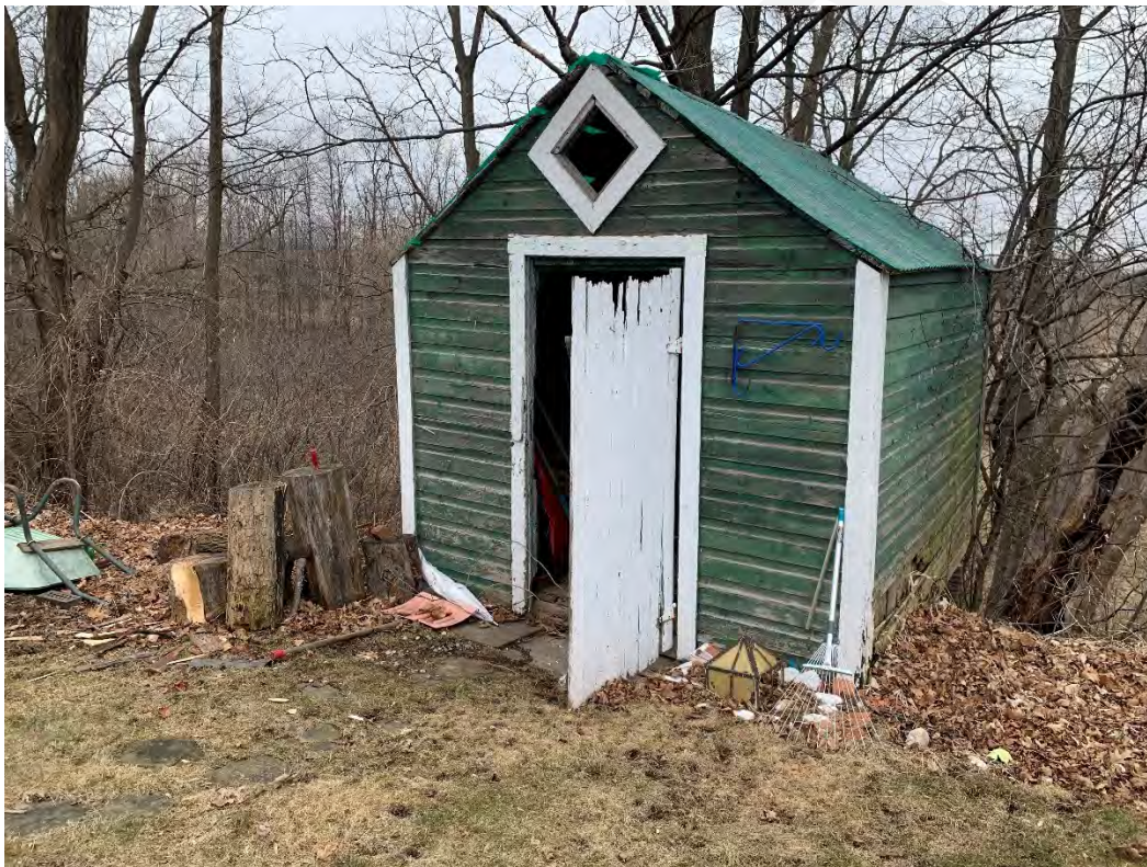
Figure 15: View of shed along valley (CU 2020).
