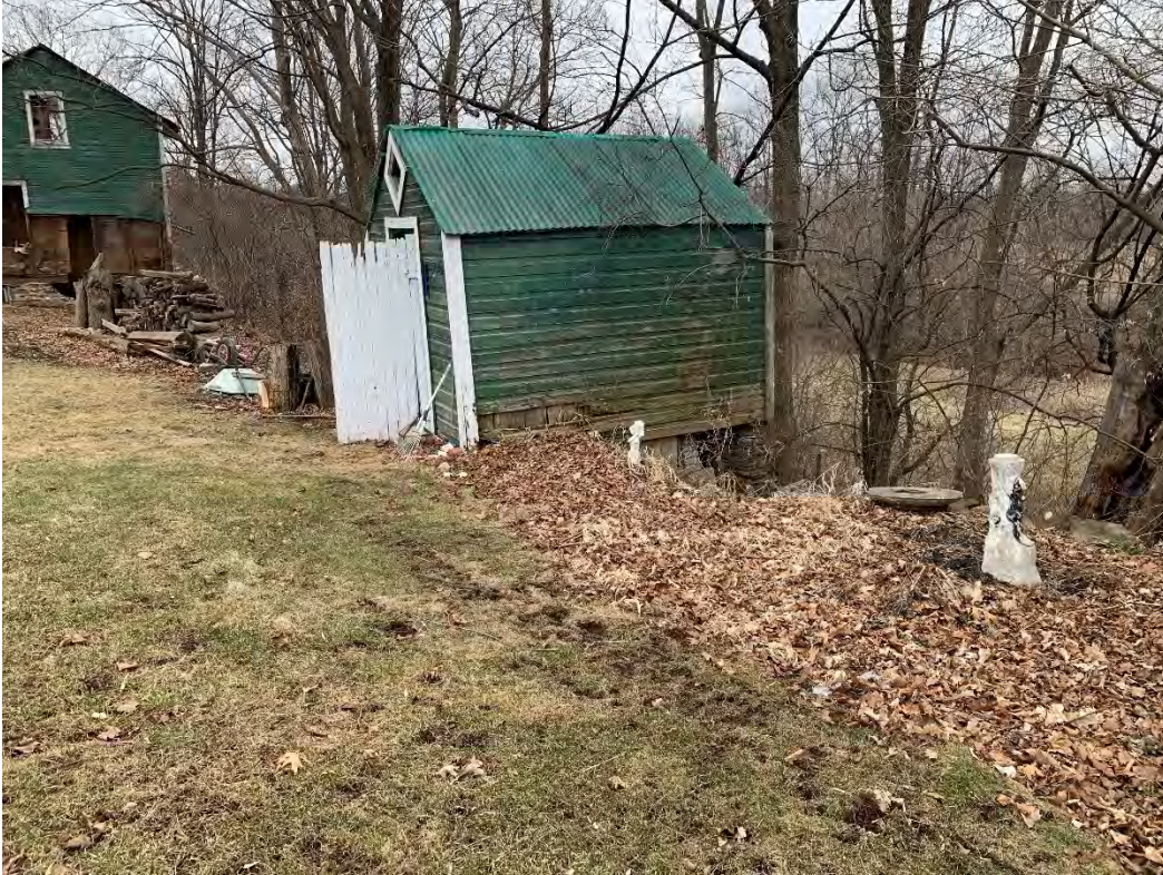
Figure 16: View of shed along valley, looking west (CU 2020).
