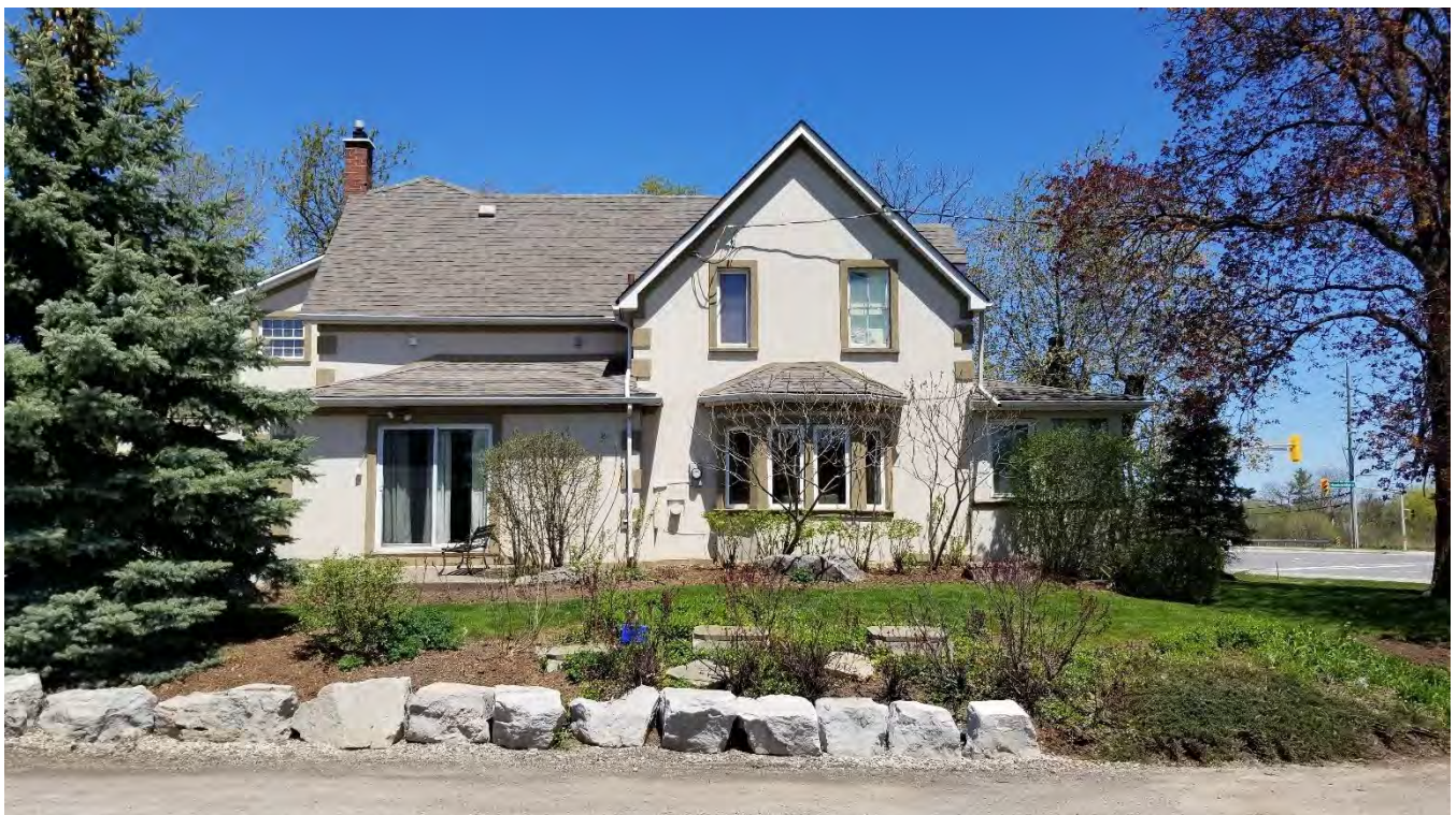
Figure 12 Southwest façade of Turner House.
