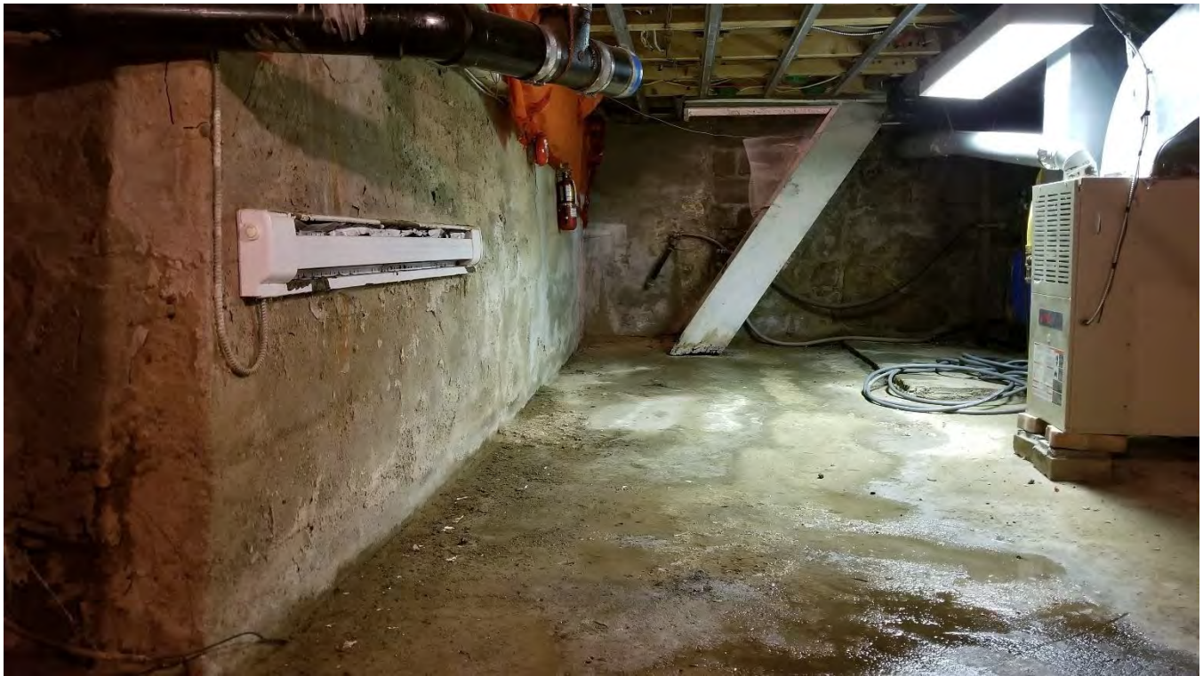
Figure 51 Basement, looking northwest.
