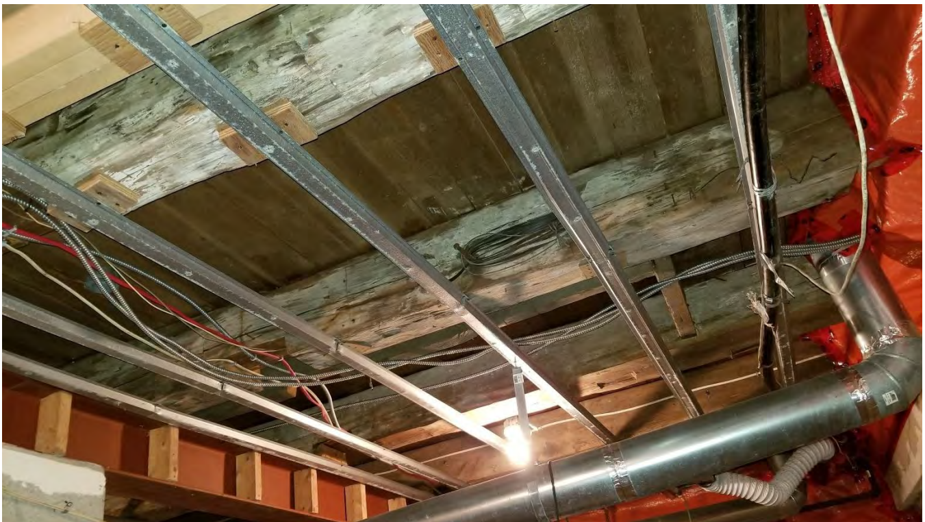
Figure 40 Hand hewn joists and steel I-beam reinforcement.
