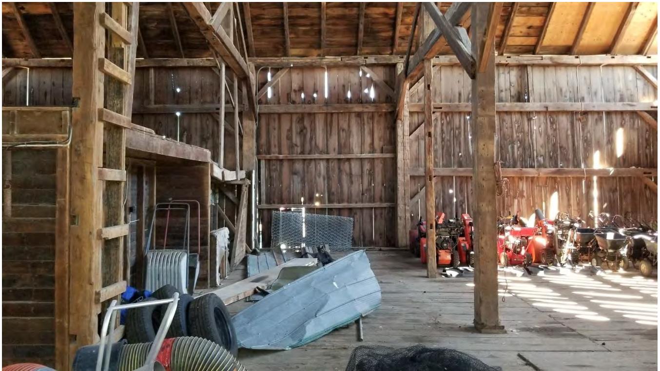
Figure 88 Second floor of the barn, looking southeast.
