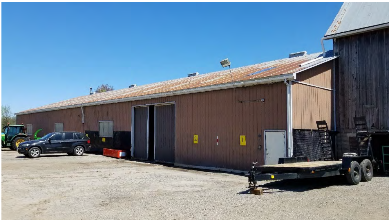
Figure 76 Northwest elevation of extension.
