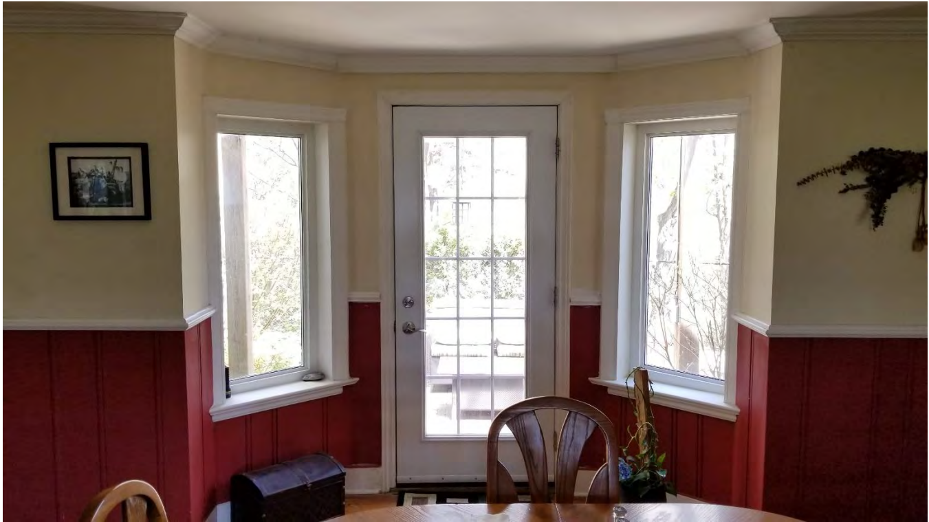
Figure 30 Bay window on the northeast wall of the main block. The central opening has been converted to a door.
