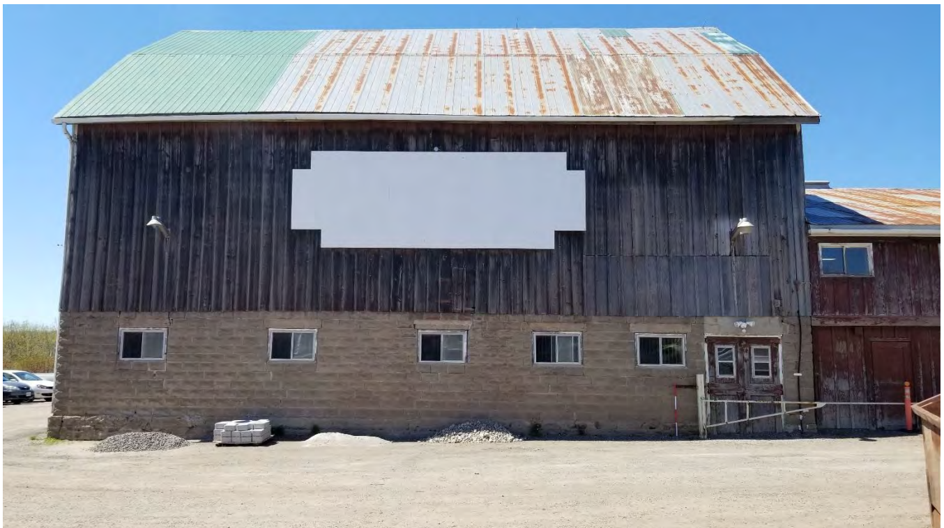
Figure 72 Southeast elevation of the barn and board and batten extension.
