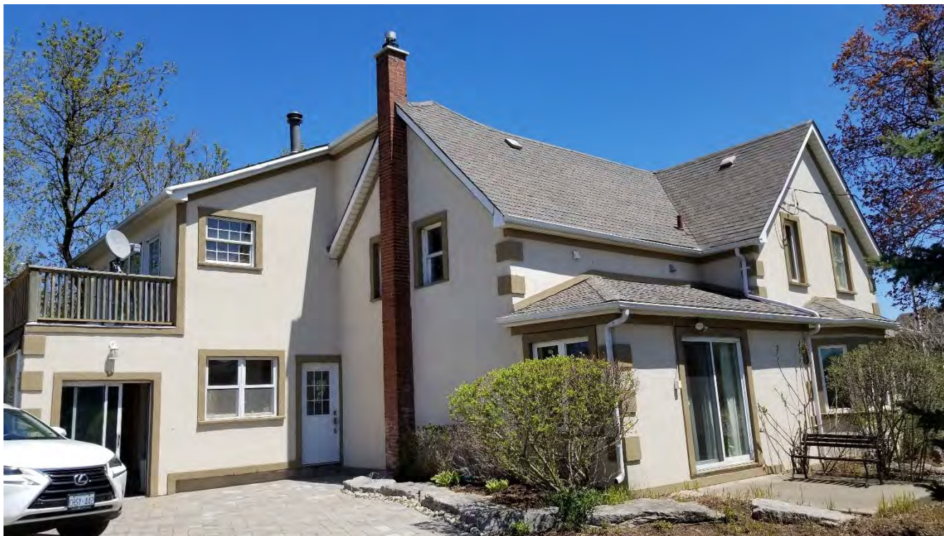
Figure 13 Southwest and northwest façades of Turner House.
