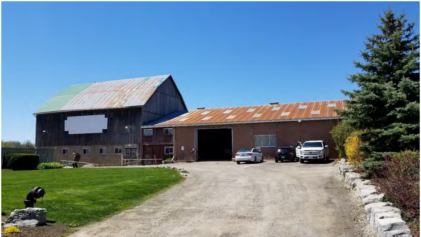
Figure 69 Southeast elevation of the barn and extension.
