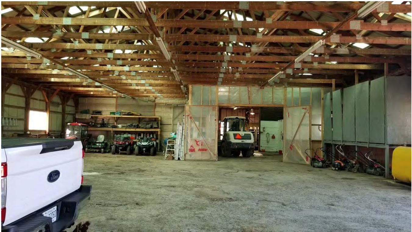
Figure 94 Aluminum extension, looking northeast.
