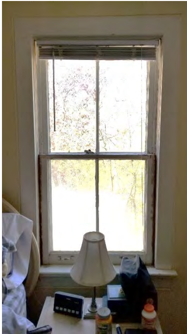
Figure 35 Two-over-two window with wood trim in northeast bedroom.
