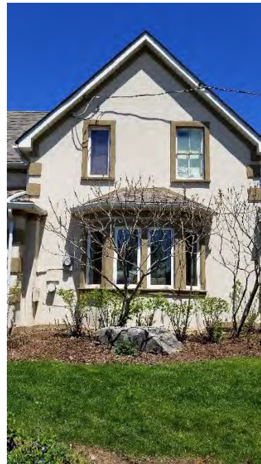
Figure 21 Bay window, two-over-two window, and rectangular flat glazed window on southwest façade of main block.
