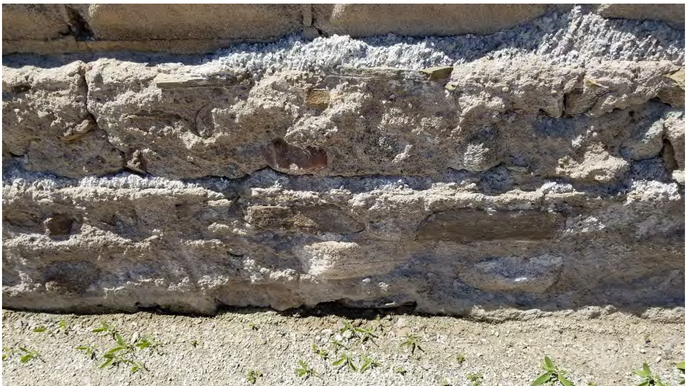
Figure 70 Coursed rubble stone foundation of the barn.
