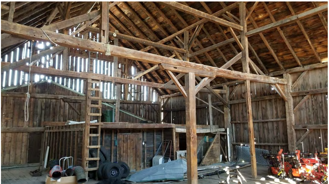
Figure 87 Second floor of the barn, looking east.
