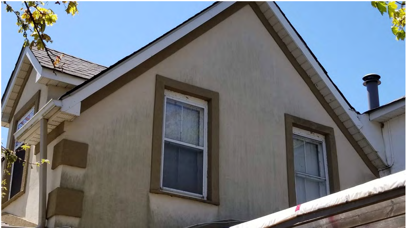
Figure 22 Two-over-two windows on the northeast façade of the main block.
