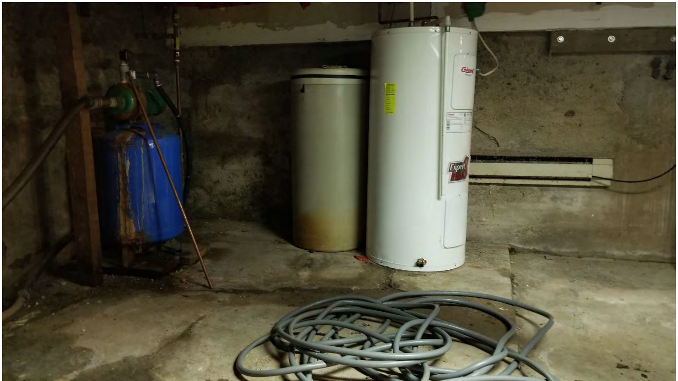
Figure 53 Basement, looking north.
