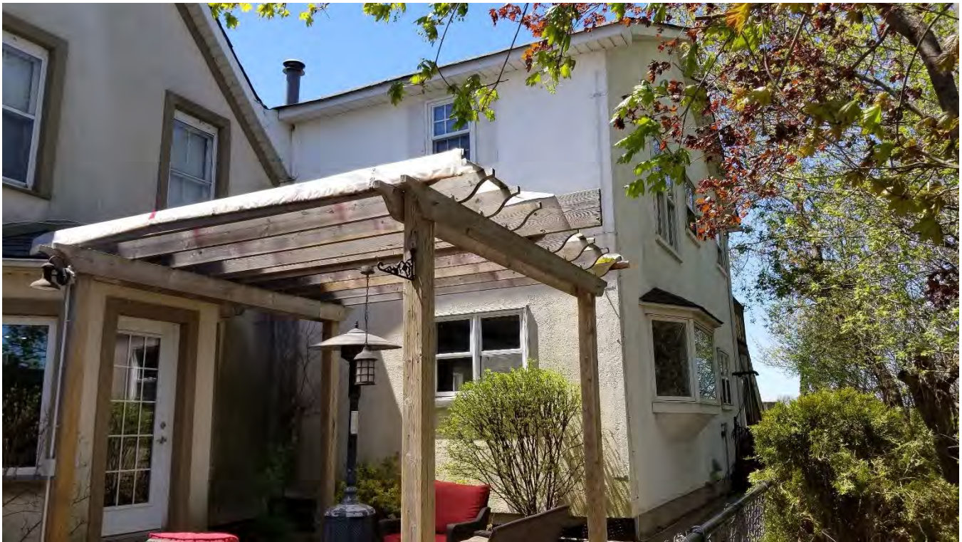
Figure 15 Northeast and southeast façade of Turner House.
