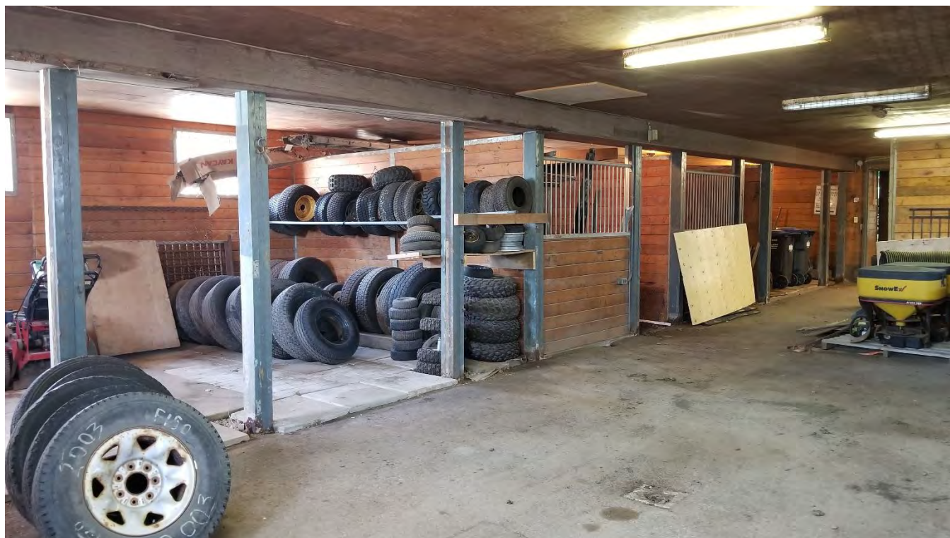
Figure 82 Ground floor of the barn, looking north.
