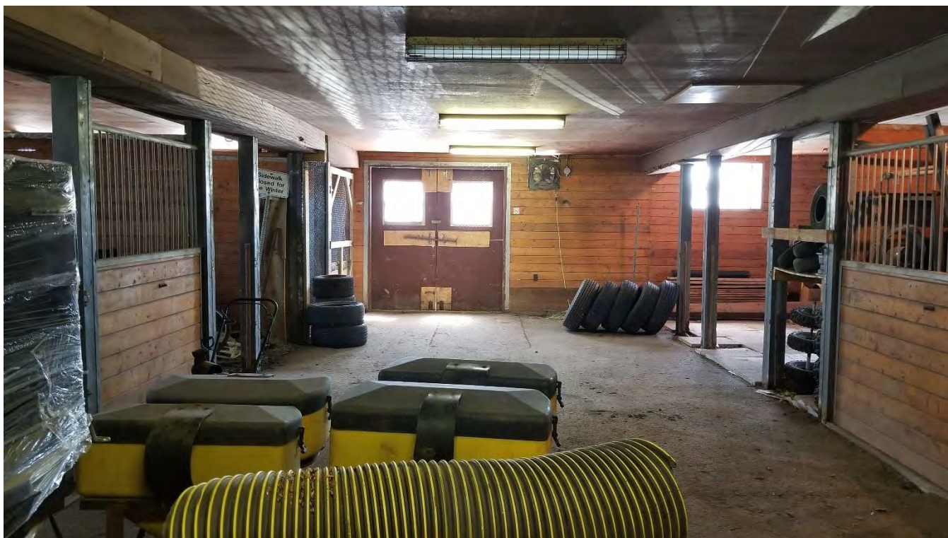
Figure 80 Central passage of the barn with stalls on either sides, looking southwest.
