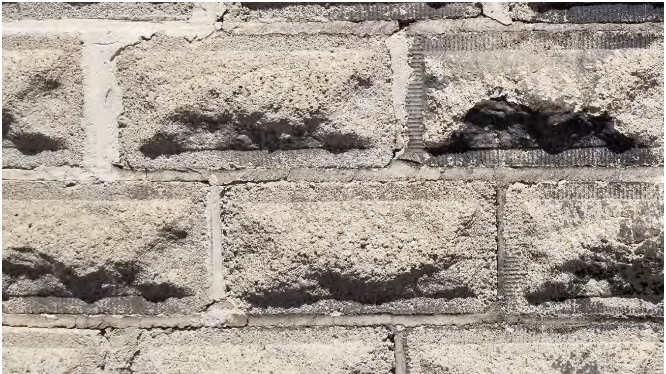
Figure 71 Rock-face CMUs with tooled edge
