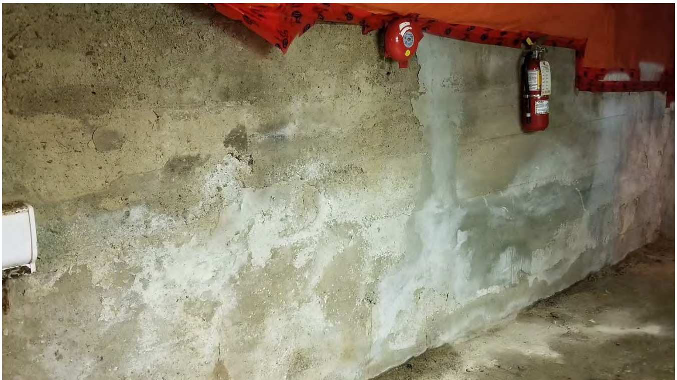
Figure 52 Southwest basement wall showing evidence of form boards.
