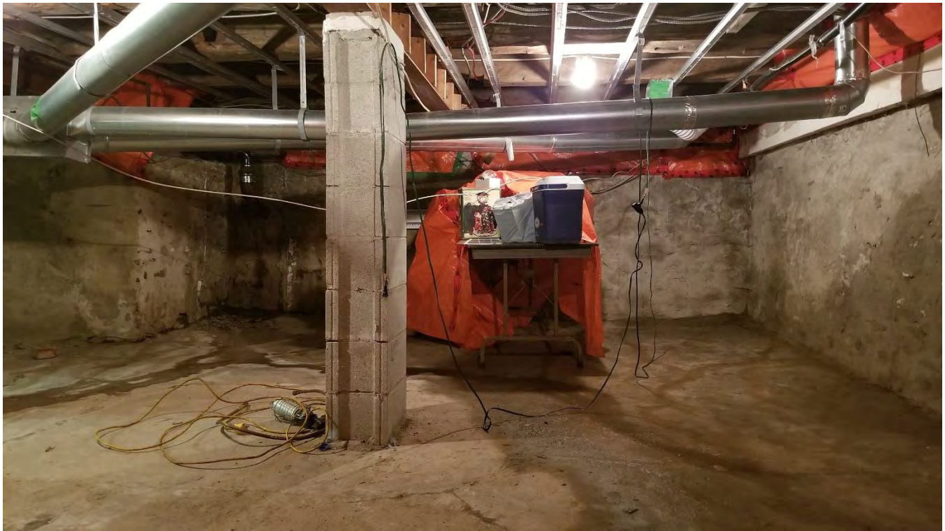
Figure 37 Basement, looking northeast.
