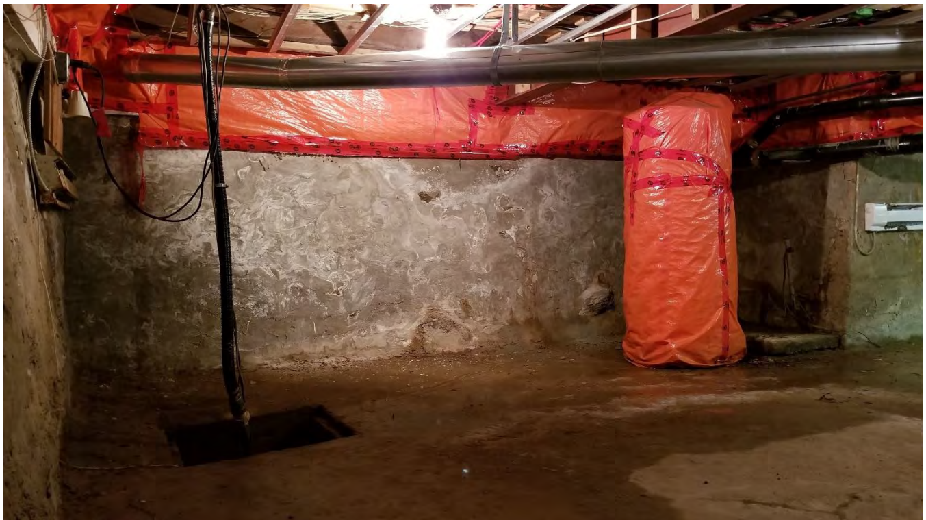
Figure 38 Basement, looking southwest.
