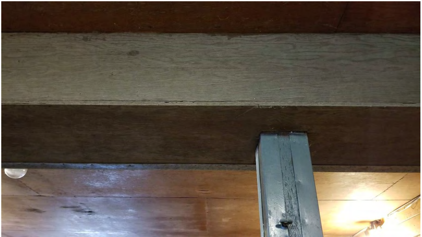
Figure 84 Milled dimensional post supporting the second floor and plywood covered beam.
