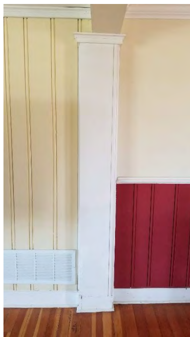
Figure 28 View of pilaster, baseboards, crown moulding and beadboard.
