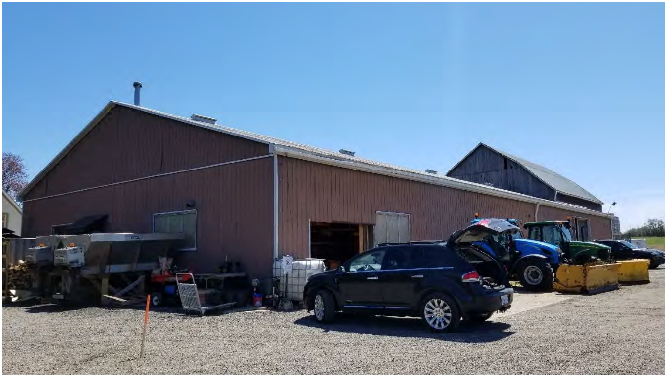
Figure 77 Northwest and northeast elevation of aluminum extension.
