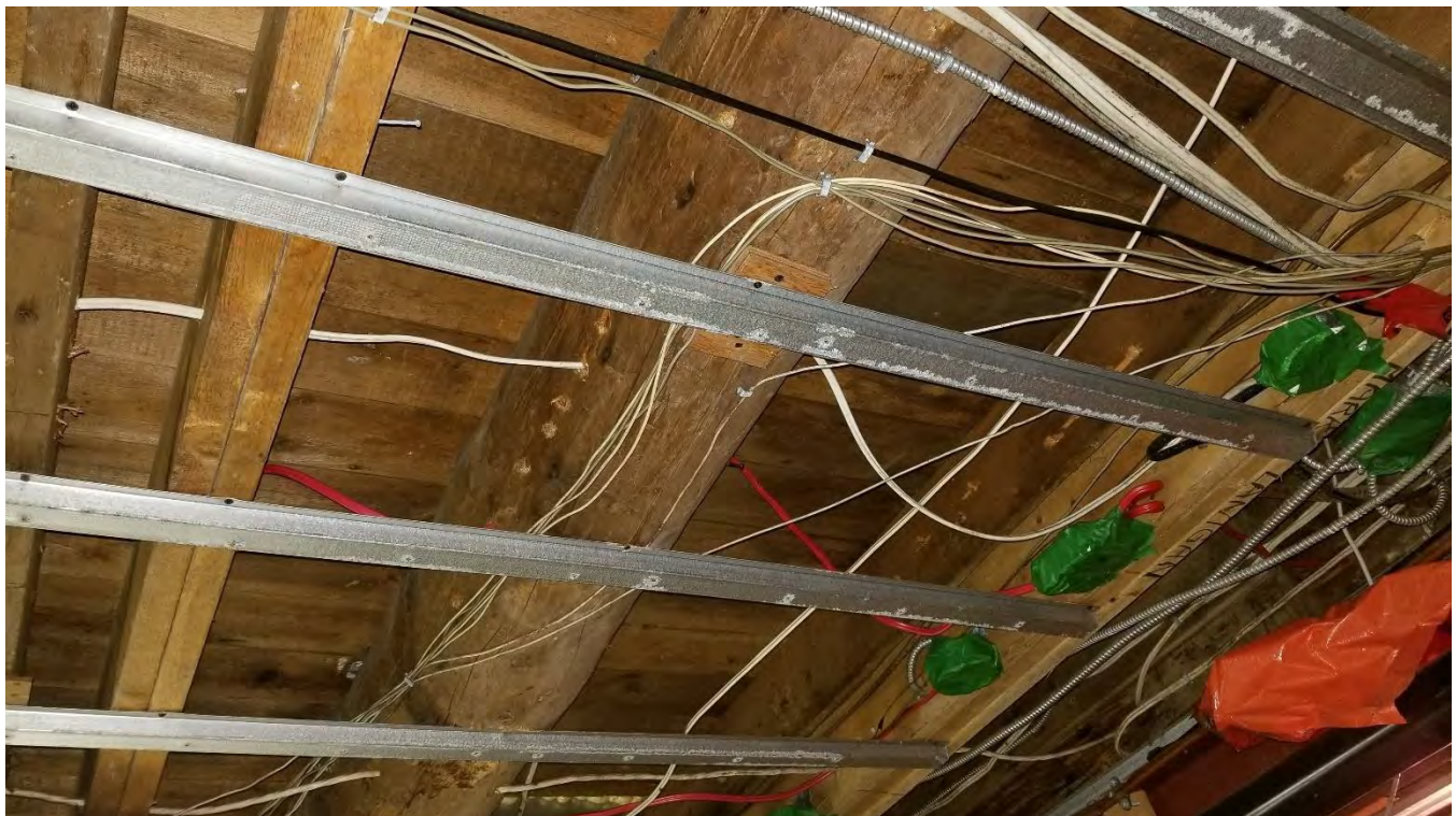
Figure 54 Basement, round timber and dimensional joists.
