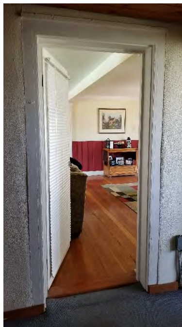
Figure 23 Original main entrance of the main block; now enclosed by the front extension.
