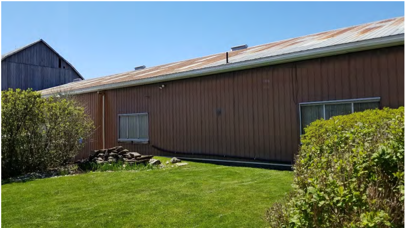
Figure 79 Southeast elevation of aluminum extension.
