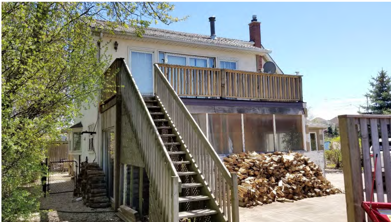
Figure 14 Northwest and northeast façades of Turner House.
