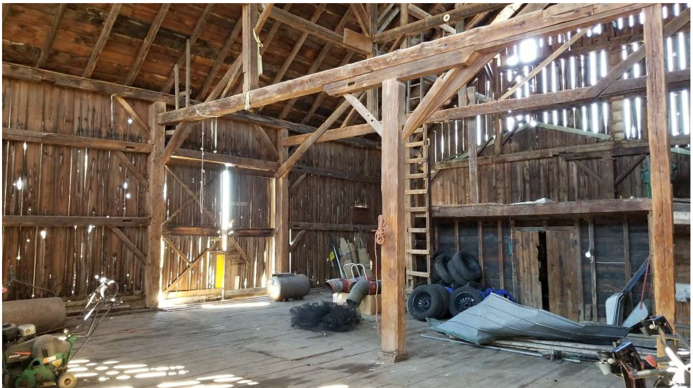
Figure 85 Second floor of the barn, looking north.
