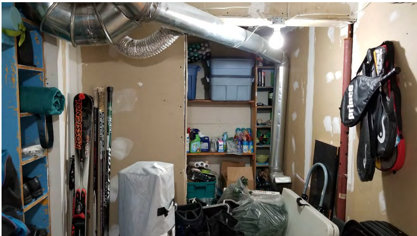
Figure 45 Storage room, looking northeast.
