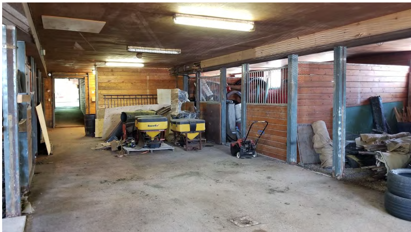
Figure 83 Ground floor of the barn, looking northeast.
