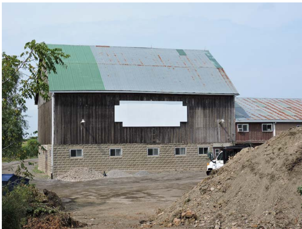
Figure 7: Bank barn, south elevation (AB, 2015)
