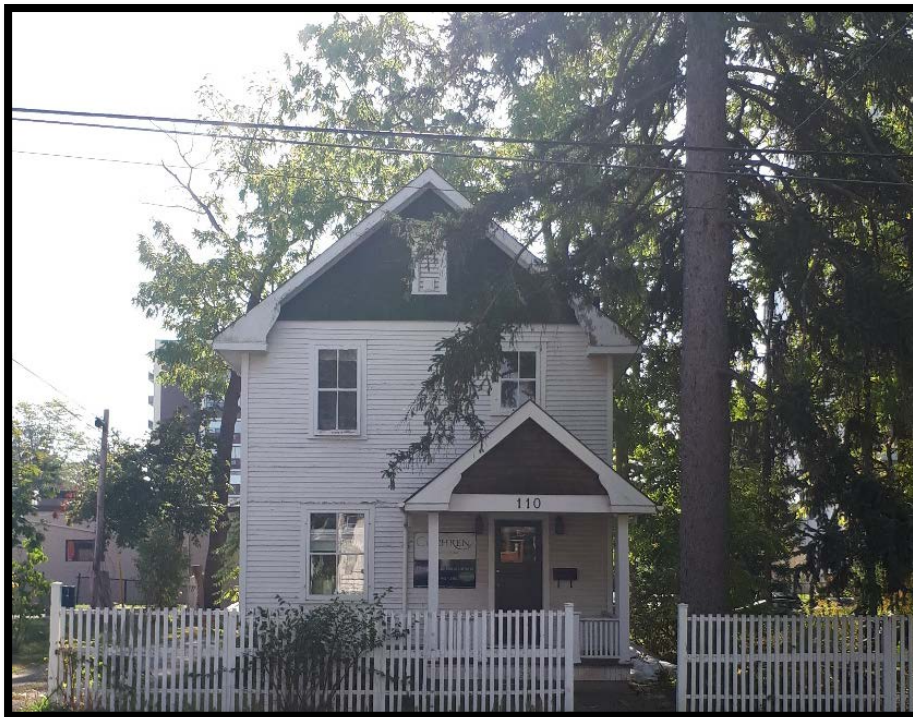
Figure 22: Front façade of house located at 110 Deane Avenue (MHBC, 2019)
