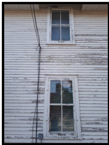
Figures 25, 26 & 27: (Above) View of east façade showing condition of clapboard cladding and location of original windows; (Below left) View of original windows to the left of the façade showing deteriorating condition; (Below right) View of original windows to the right of the façade showing break between the original soffit and newer soffit (MHBC, 2019)
