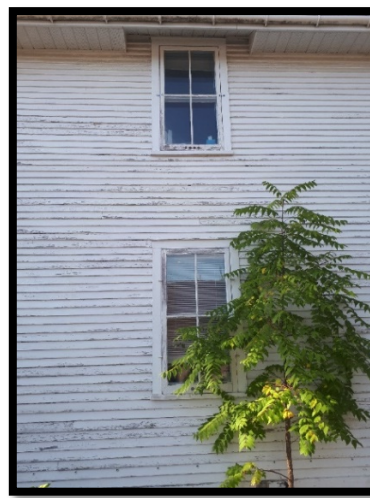
Figures 25, 26 & 27: (Above) View of east façade showing condition of clapboard cladding and location of original windows; (Below left) View of original windows to the left of the façade showing deteriorating condition; (Below right) View of original windows to the right of the façade showing break between the original soffit and newer soffit (MHBC, 2019)
