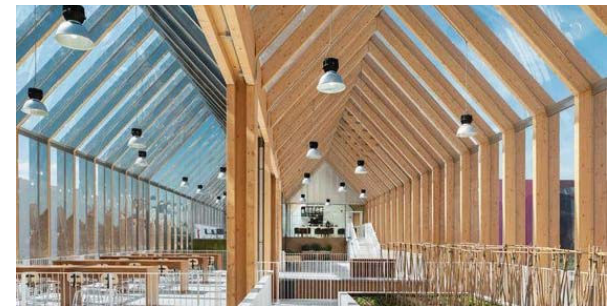
WOOD STRUCTURE WITH GLAZED ROOF
