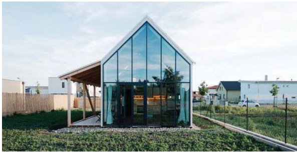
SYMMETRICAL CENTRAL PITCH WITH LOW SLOPE SIDE ROOF
