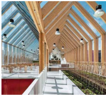
GLASS ROOF WITH EXPOSED WOOD STRUCTURE
