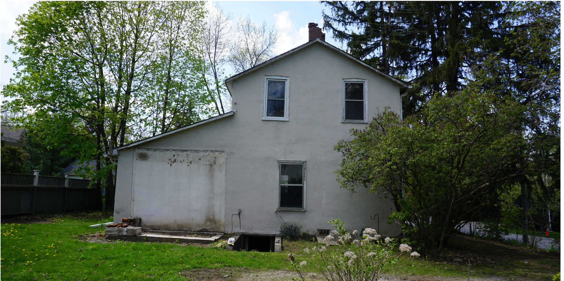
Rear view from South East - Access way to the basement, the foundation of a former addition and the additions outline on the rear can all be seen in the above photo
