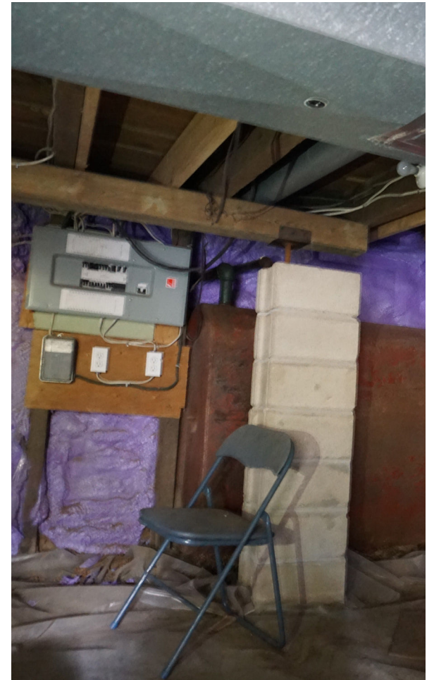
View of a column and post added to support the floor
