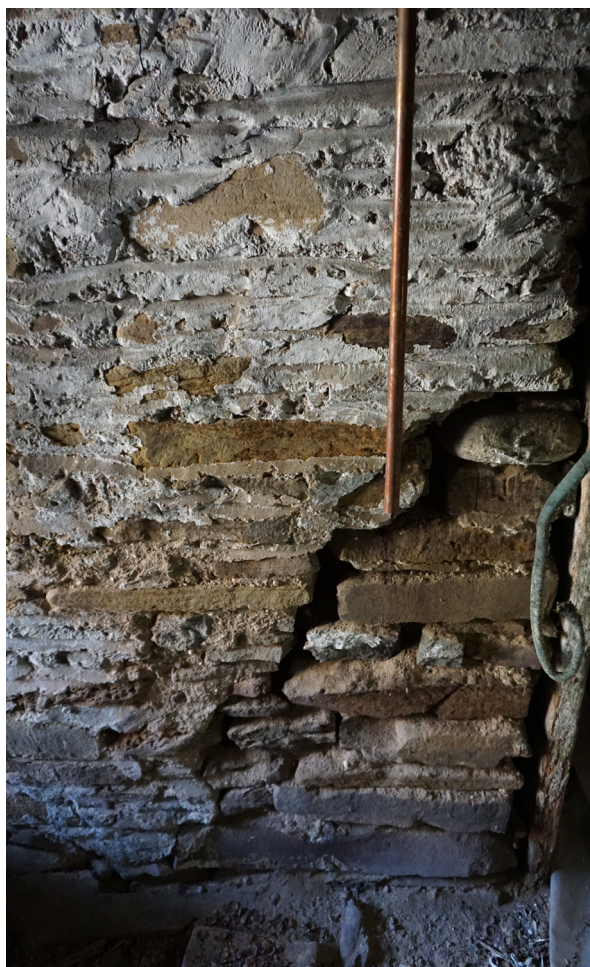
Lake Stone Foundation degradation
