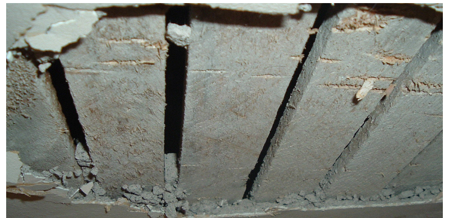
Views of the interior wall construction/wood lath and plaster
