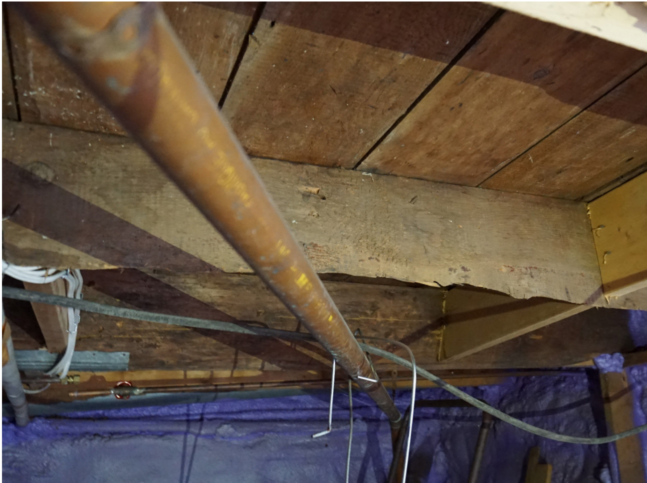
View of rotting joists in the basement
