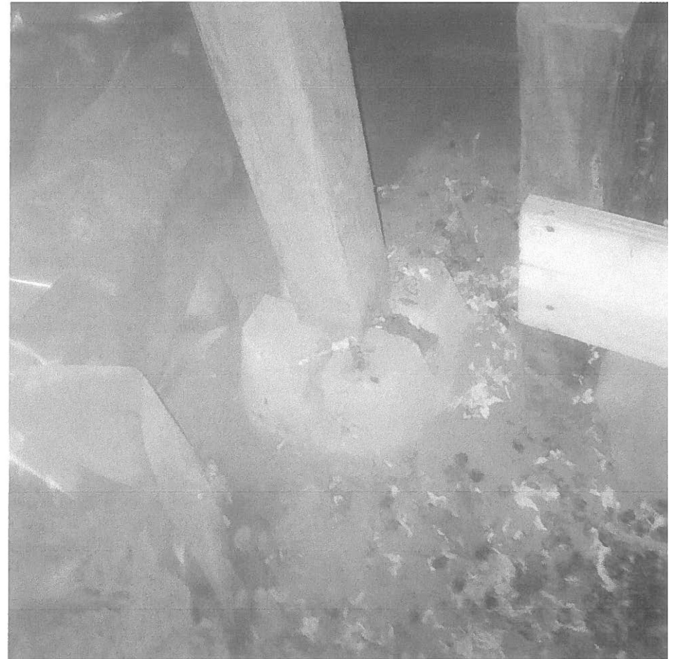
Figure 1.0 Photo of Main Floor Support Structure (Remedial Works) – Inadequate Support Post/Foundation
