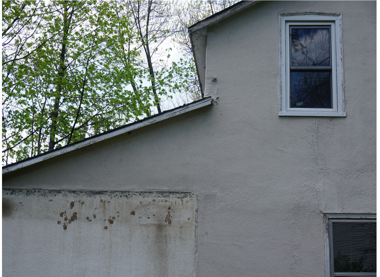
Cracks, deterioration, and outline of a former addition visible on the Exterior wall
