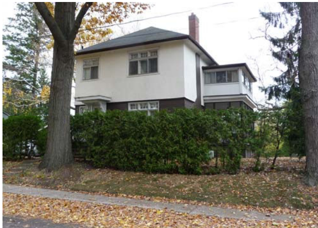
Figure 4 – Southwest corner view
