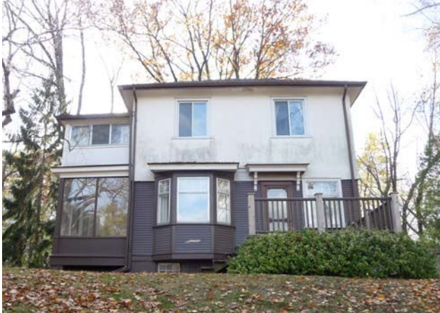
Figure 6 – West/rear elevation view
