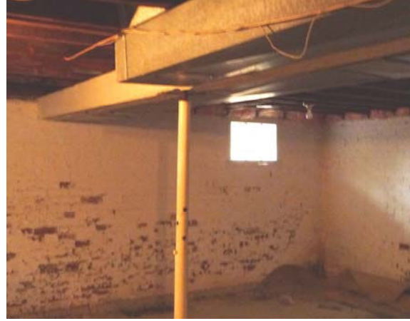
Figure 7 –Interior, brick foundation
