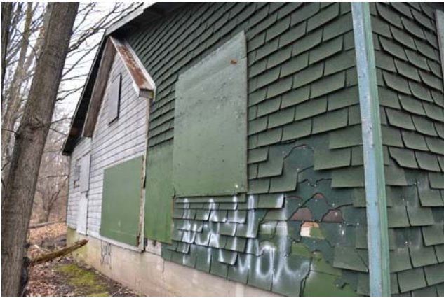
Rear wall of garage. [Staff photo 2020]
