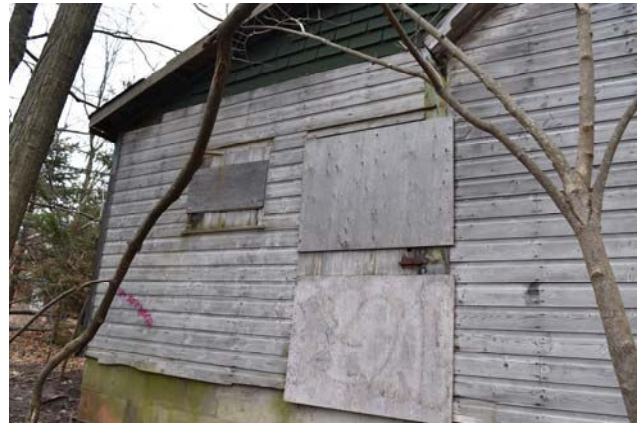
Rear wall of garage. [Staff photo 2020]
