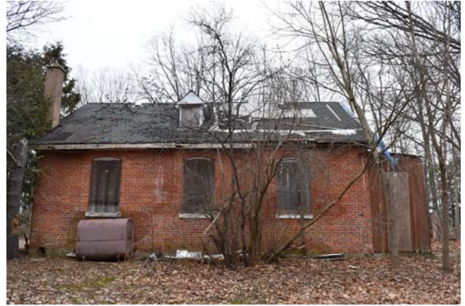
West elevation. [Staff photo 2020]
