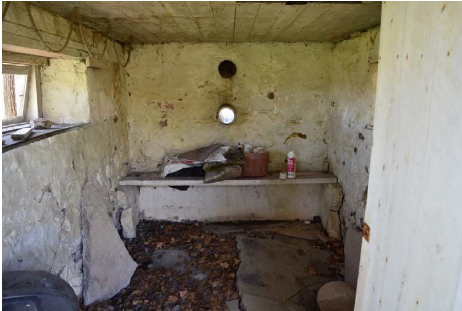
Figure 18: Interior of the butter dairy looking westward (to Tremaine), showing the flue for the brick chimney and light coming through the lower terra cotta pipe through which cooling water was delivered to the trough (Town of Oakville staff, May 2017).
