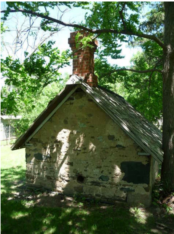
Figure 19: Rear elevation of the butter dairy showing the terra cotta pipe that provides access to the interior. Note that the chimney flue is not visible, unlike with the interior (E. Tumak, June 2018).
