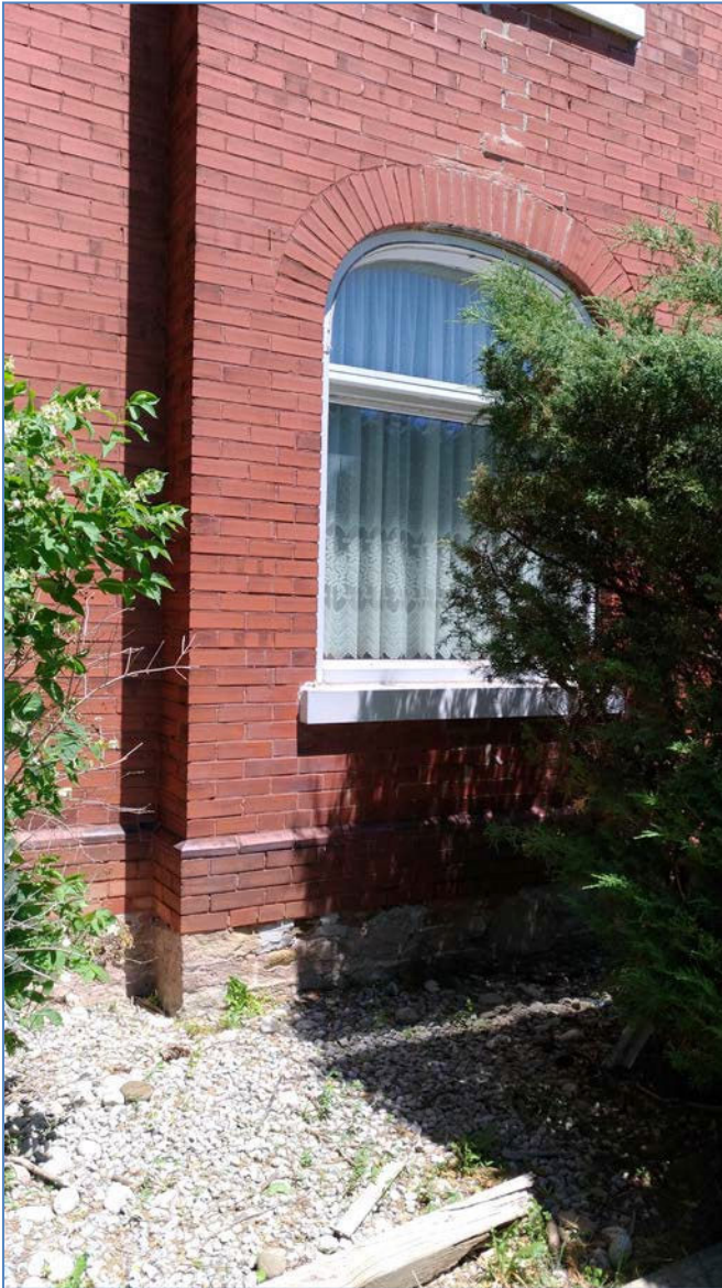
Figure 13: Main level section of 2.5 storey gable bay, showing the basket-handle arch and the angled brick protective drip line for the foundation (E. Tumak, 2018).
