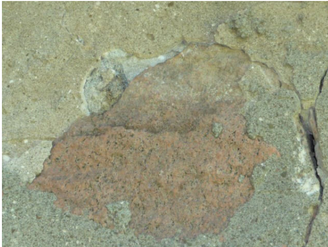
Figure 17: Detail of rough rubble stone construction showing the overlay of a later parge (E. Tumak, 2018).
