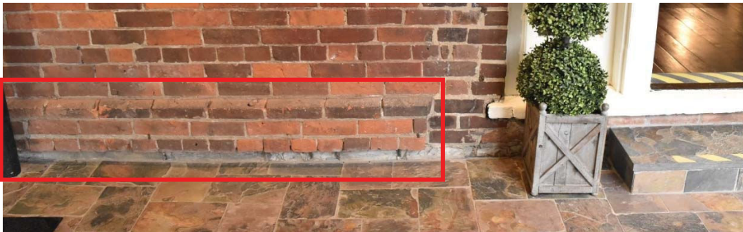
Figure 23: Projecting brick and mismatched brick colours as possible evidence of extent of 1858 residential addition. Erchless , east façade in Museum vestibule entryway.
