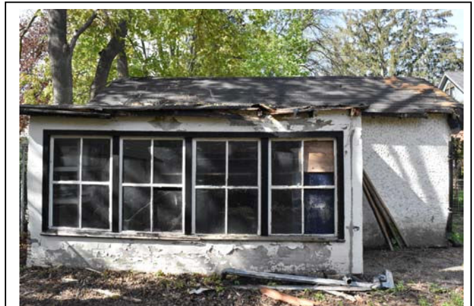
East elevation of garage.
