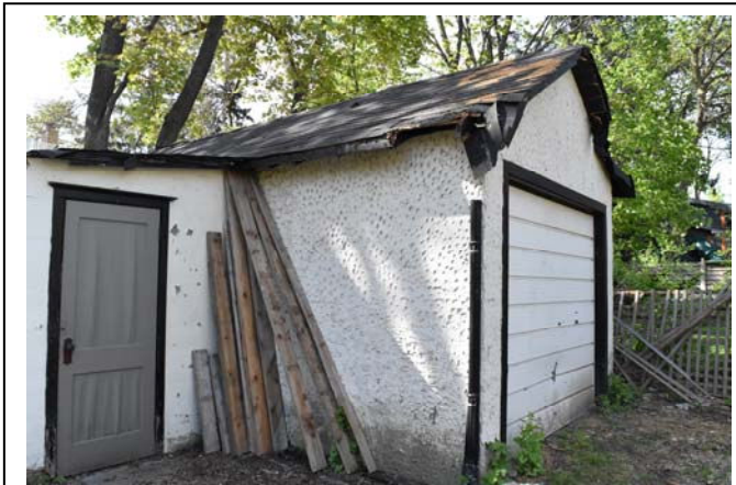
North and east elevations of garage.
