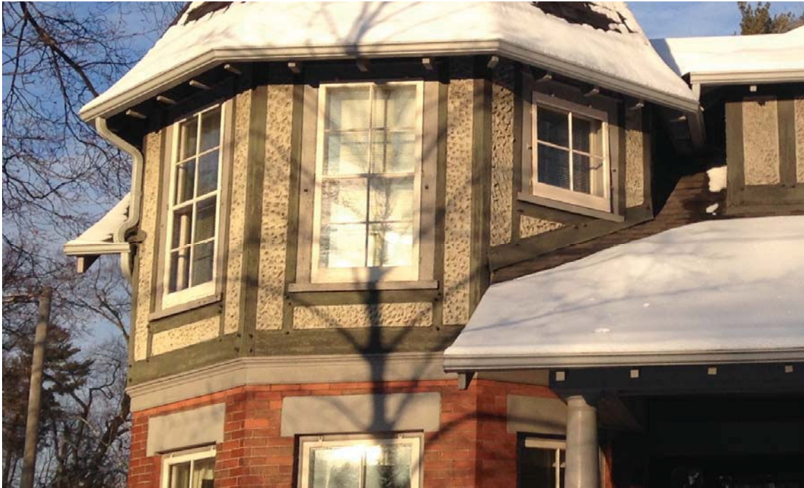
2.16 #359 Douglas Ave., Oakville. Another example of Tudor Revival with stucco in panels. In this beautiful example the “half timbers” are actually pegged in place with protruding oak trenails. The stucco has light texture with small triangular indentations made with the trowel, circa 1910. Stucco was not painted but left exposed to weather along with the stone lintels, sills & freize board painted a colour similar to that of the limestone lintels. The eavestroughs are modern and cover the rafters.
