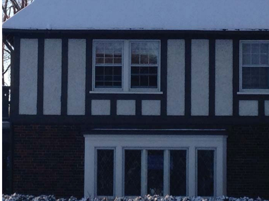
2.20 # 429 MacDonald Ave. This is another example of an early 20 th . C. “Tudor Revival” house, with a subtle mix of brick textures at the ground floor and center gable, “half timber and stucco” at the second floor flanking the center gable, and a heavy timber portico at the entry. The timbers are raised away from the pebbly stucco and protect it from weather. The proportions of timber to stucco are similar to that of medieval wattle and daub infill. The absence of diagonal braces makes this design slightly monotonous and formulaic.
