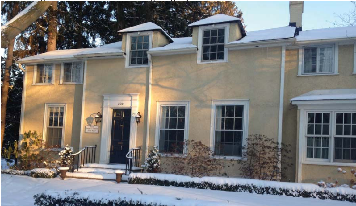
2.21 #320 George Street. Much modified house circa 1859, with additions in early 20 th . C. The stucco is slightly rough but without rusticated embellishment and sweeps. Many houses in the center of town have a consistent texture & workmanship, often painted as here to conceal several stages of repair and addition. This is vernacular rather than Arts and Crafts.
