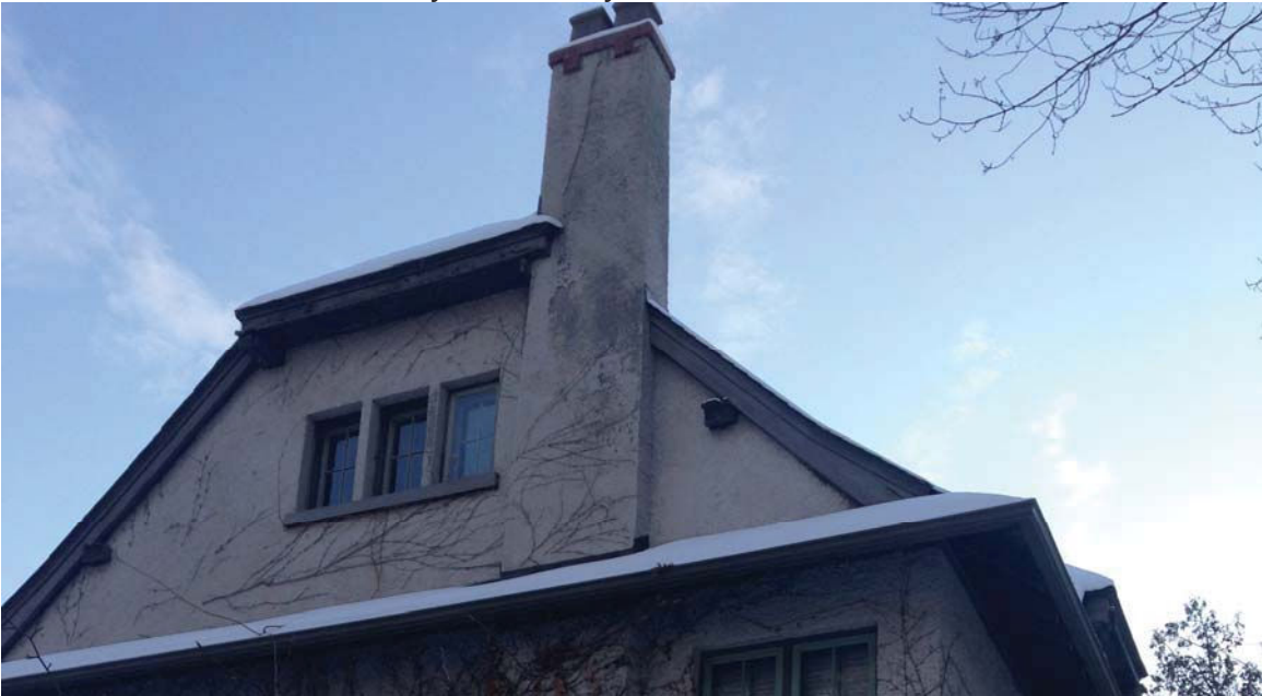
2.19 Another example of smooth Arts & Crafts stucco circa 1910, 335 Watson Ave. The small brackets are integrated with fascias & mouldings projecting eaves with exposed rafter tails multiple "ganged" windows, and emphasized chimneys with ornamental caps & flues. The effect is subtle & carefully planned. No "half timbering" was used but brick details were added to punctuate the stucco at sills and corners. This sophisticated example with hipped gables is more German or Baltic than British though the window arrangements are similar to those of C.F.A. Voysey, an exemplary Arts and Crafts Architect.
