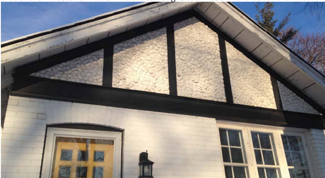
2.17 # 379 Douglas . A timid sort of “half timber” with small boards at wide spacing. The panels are not stucco but painted cobble infill, convex in form. concave. The moderate (4”) size cobbles create the most dramatic texture found in similar age houses. The poor quality of the soffit is quite different from the previous example. This example of another ill conceived builder’s special, had brick walls and arches.
