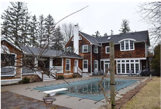
South and west elevations of the house with rear two-storey addition and side one-storey addition.
