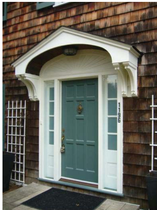
View of central entranceway, portico, sidelights and blind fanlight
