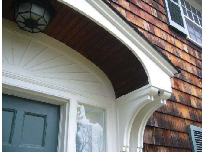
View of detail of central entranceway, portico, sidelights, blind fanlight, paired brackets and curved underside
