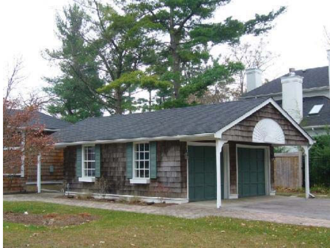
View from Linbrook Road looking southwest showing garage
