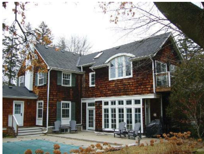
View of rear façade looking northeast.
