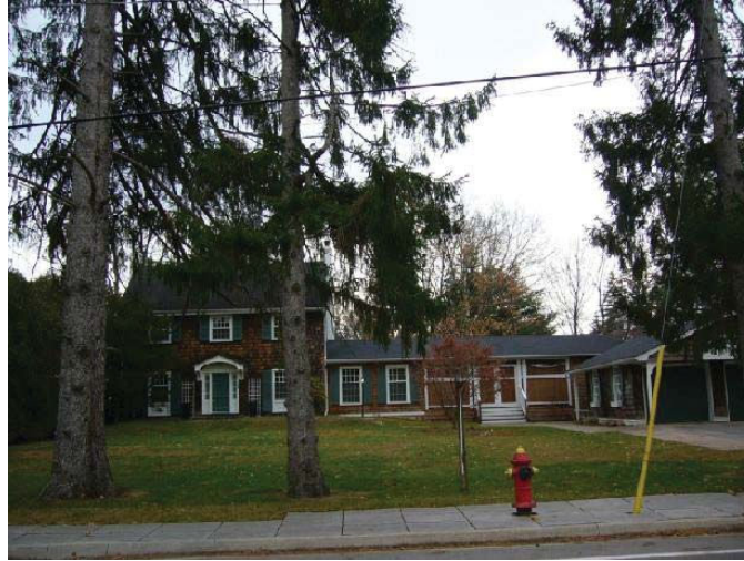
View from Linbrook Road looking south showing main house, additions and garage
