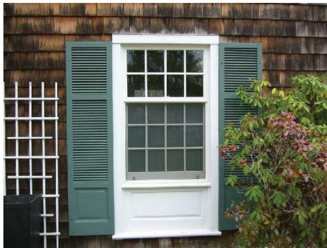
View of sash window with eight (8) over twelve (12) lights or panes flanked by faux shutters with exterior wall of wood shingles
