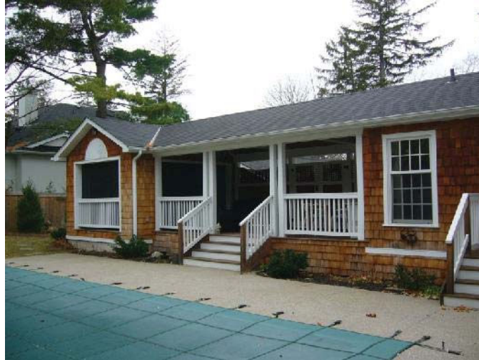
View of rear façade looking northwest showing one-storey additions.
