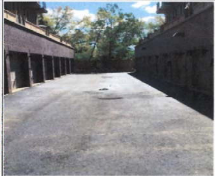
Pic 16 -Parking Garages of Four storey town homes on Royalton Common and Lillykin streets by Dunpar - Narrow parking driveways opposite to each other and no Green area
