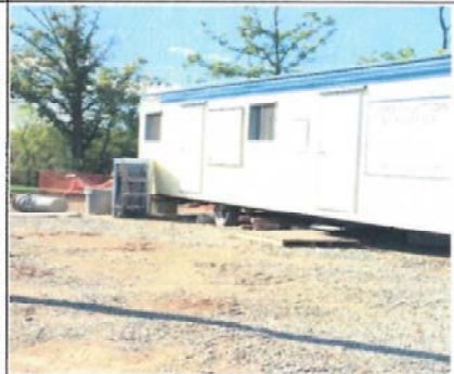
Pic 30 Biddington stacked town homes site Trailer
