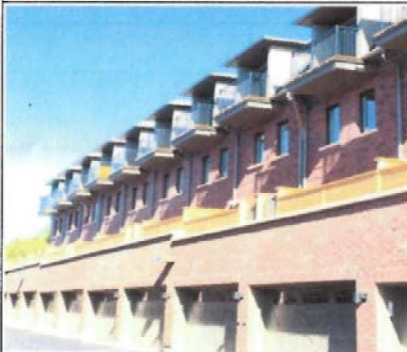
Pic 21 - DUNPAR Four-storey Town homes- Inside view.
