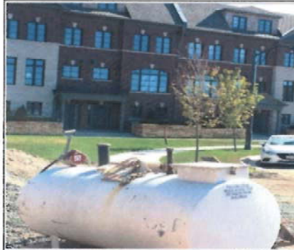
Pic 35- Biddington stacked town homes site entry & exit in front of existing town homes.
