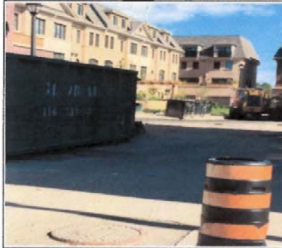
Pic 17 - DUNPAR Four-storey Town homes
