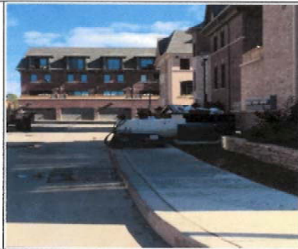
Pic 18 - DUNPAR Four-storey Town homes
