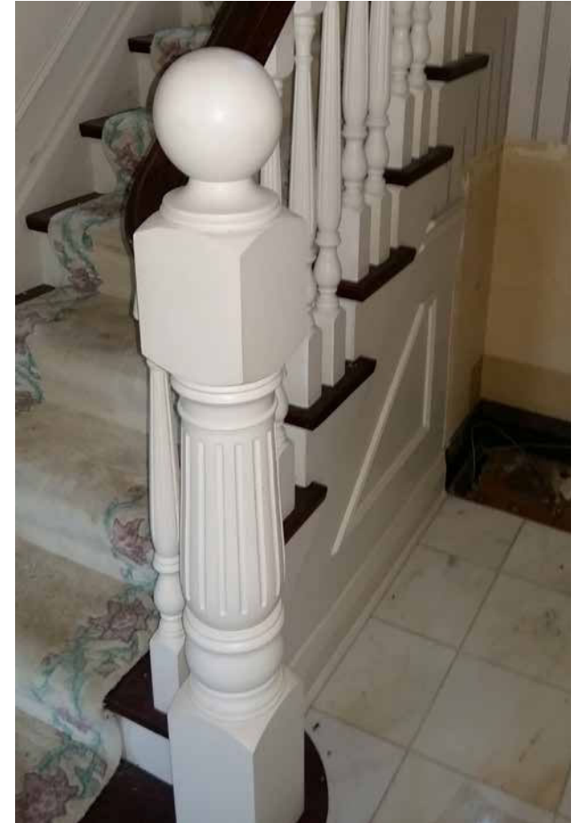
Wood newel post, balusters and railing.
