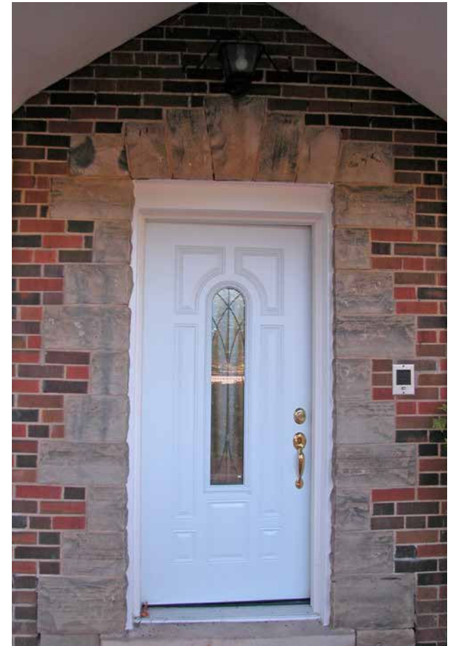
Stone quoins around the main entrance door of the original house.
