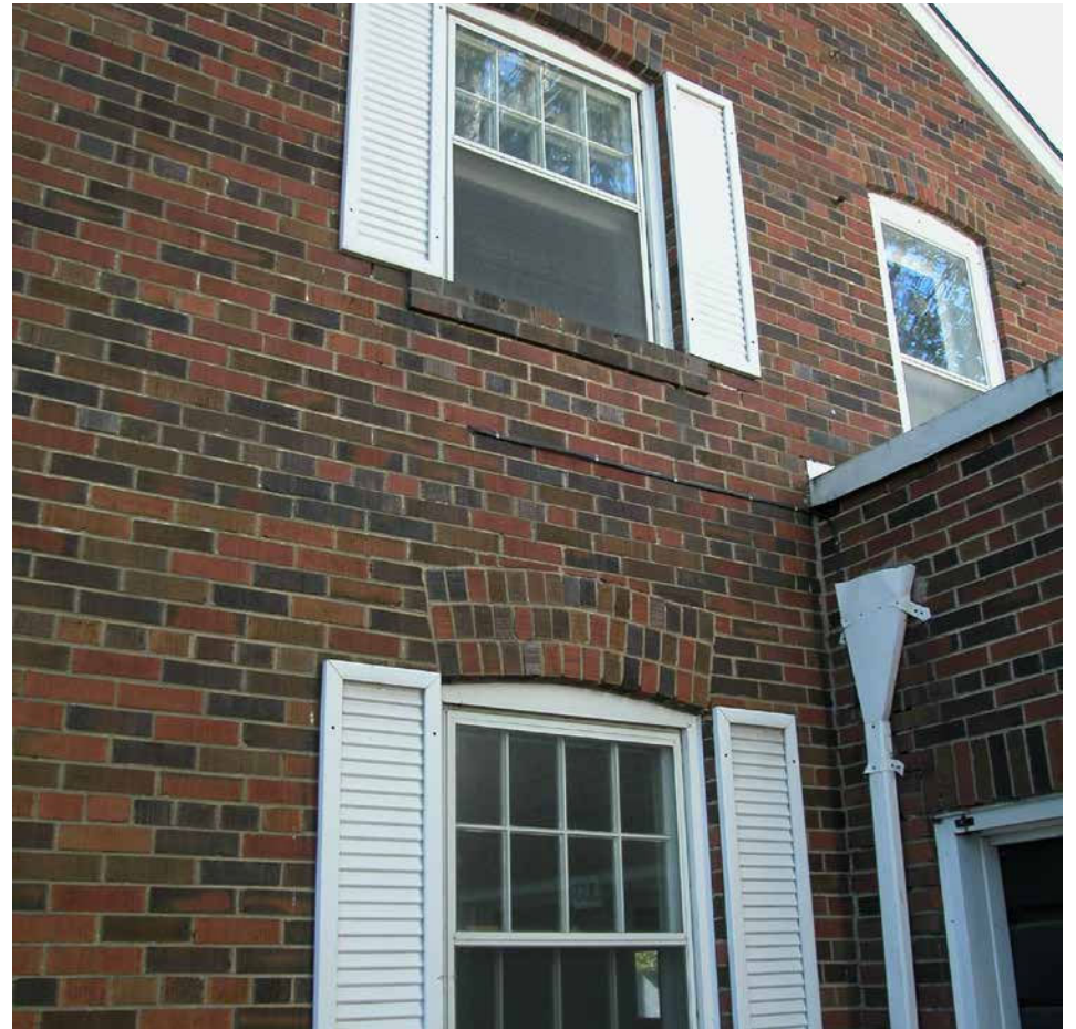
Curved brick arches are used on the original house on its east and north façades while on the south façade soldier course brick lintels are used.
