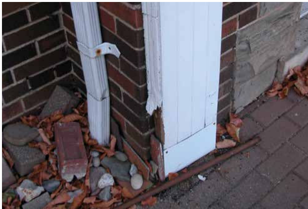
Wood trim attached to brick around the portico at the entrance.
