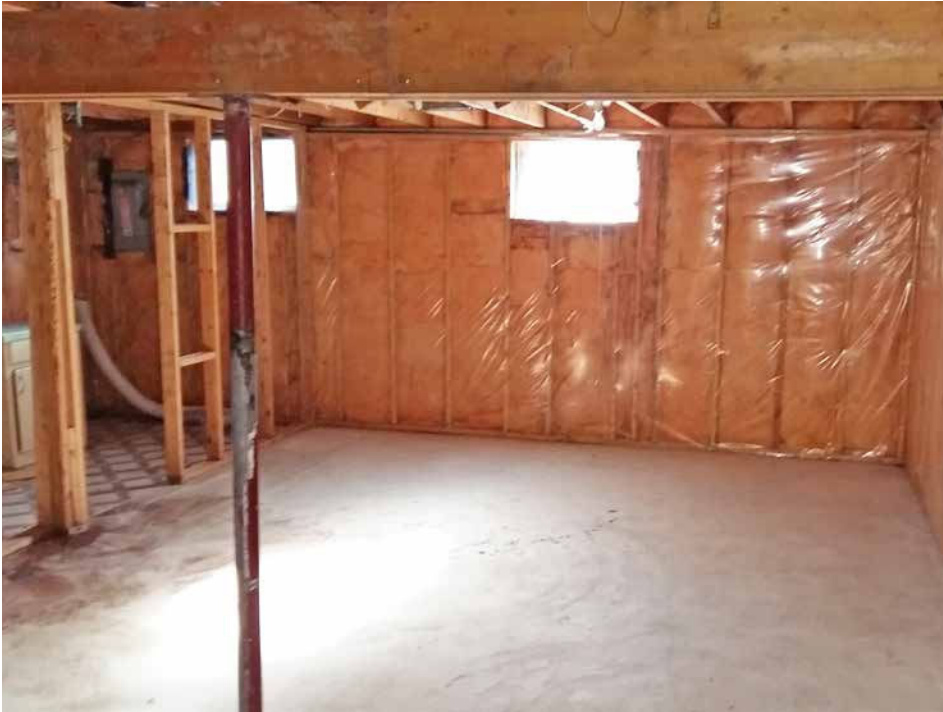
Basement of the addition is unfinished though framing and insulation are in place.
