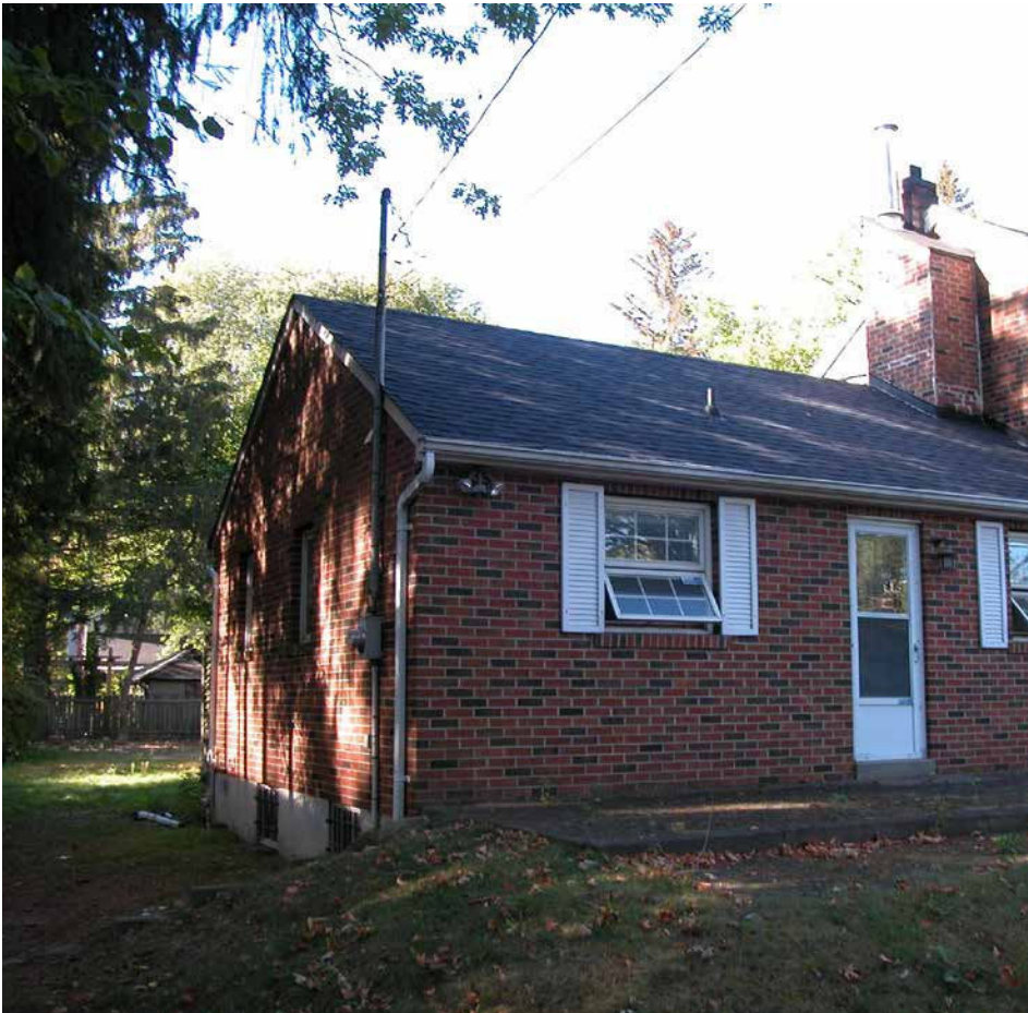
Southwest corner of the addition. Contemporary awning windows used on additions south façade.
