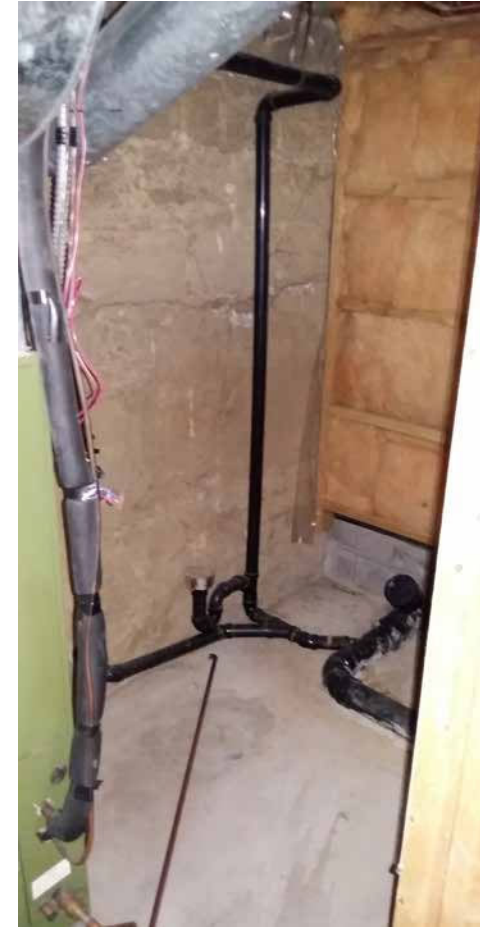
Original foundation wall between addition and original building constructed from concrete block masonry.
