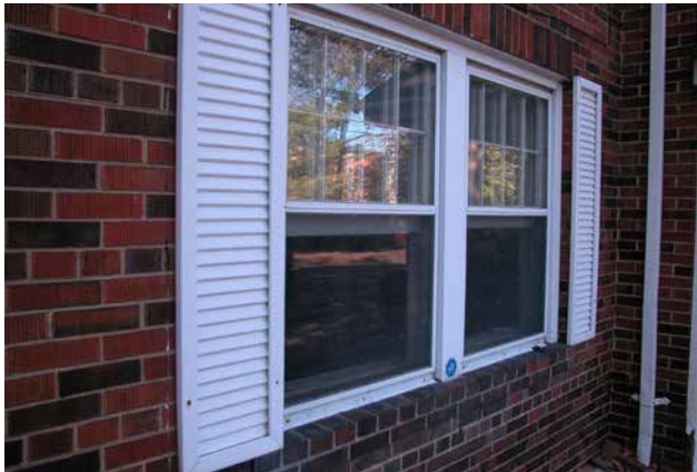
Faux shutters and aluminum storms are installed over the windows.
