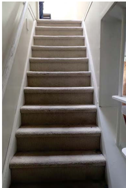
83. Good condition of stairs in 1860s section of the house.
