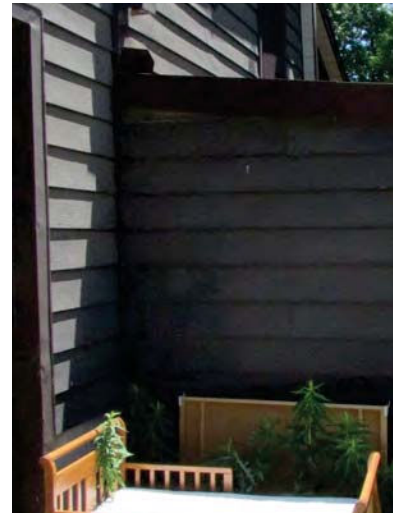
95. General condition of metal cladding (North, and West elevation)
