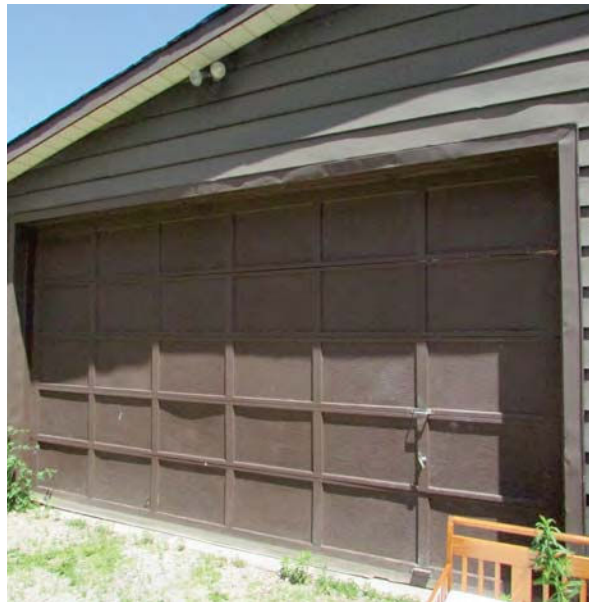
104. Garage style door (West elevation)
