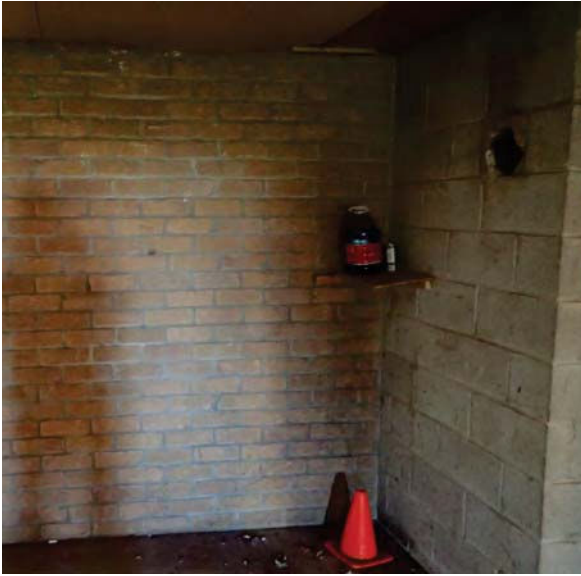
111. Fair condition of concrete blockwork, and bricks at Western extension.
