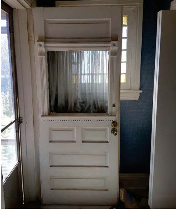
55. Good condition of entrance door.
