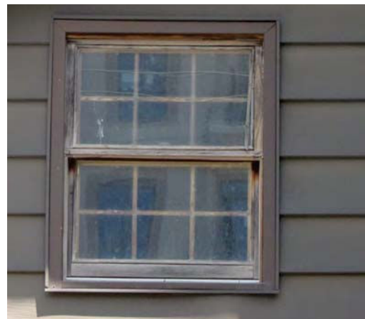
100. Weathered timber window (West elevation)
