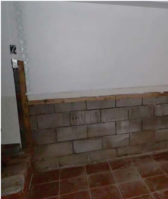
86. Removed drywall revealing concrete blockwork in 1980s basement.
