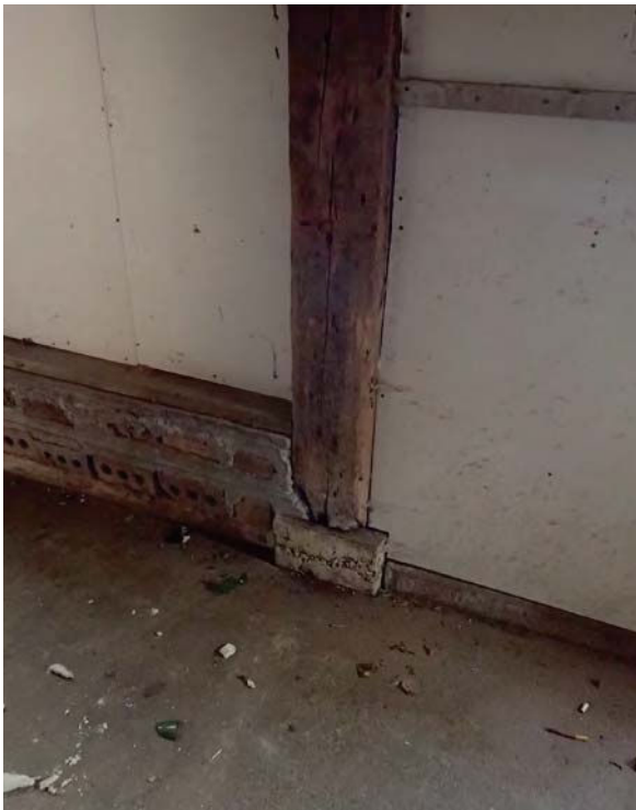
117. Base of timber post with concrete foundation.
