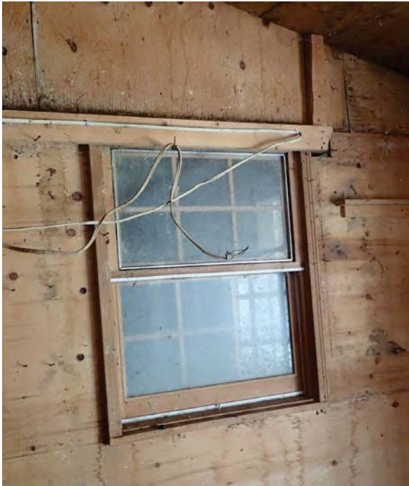
123. Fair condition of internal window.
