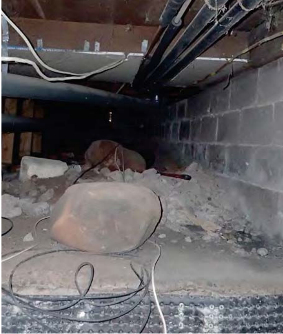
92. Crawl space underneath part of 1860s section of house.
