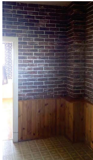
50. Good condition of faux brick effect wall covering and wood panelling.
