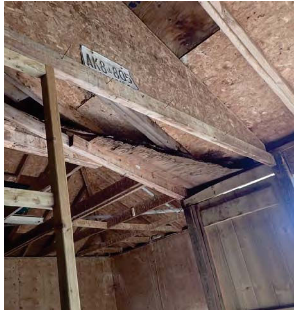
116. Fair condition of framing in Southern extension.
