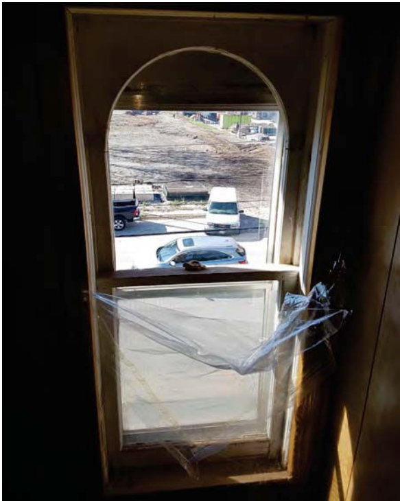
57. Fair condition of sash window in attic of 1911 section of house.
