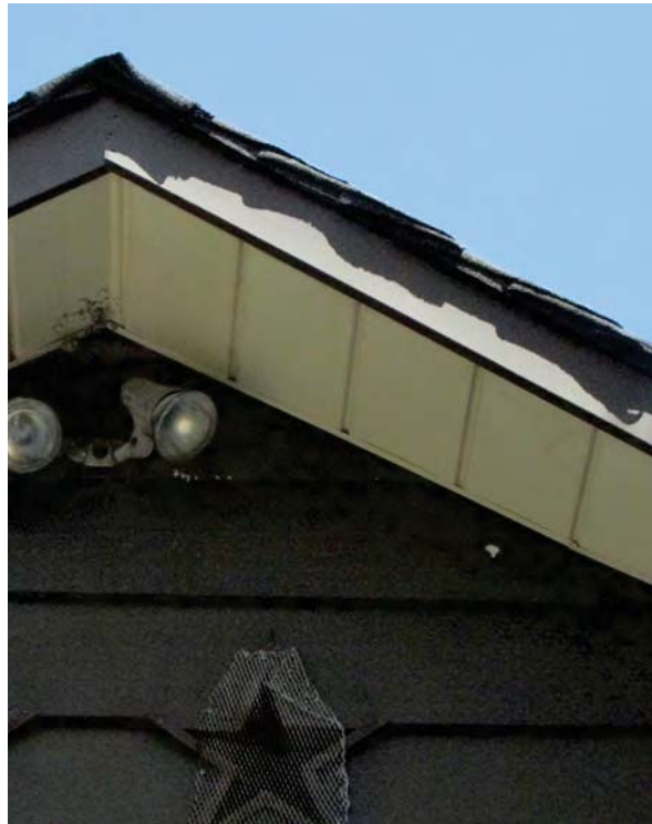
108. General condition of fascia and soffit (West elevation)
