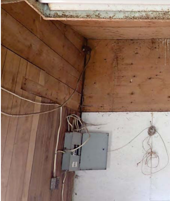
119. Fair condition of wall coverings in area labelled as 'the office'.
