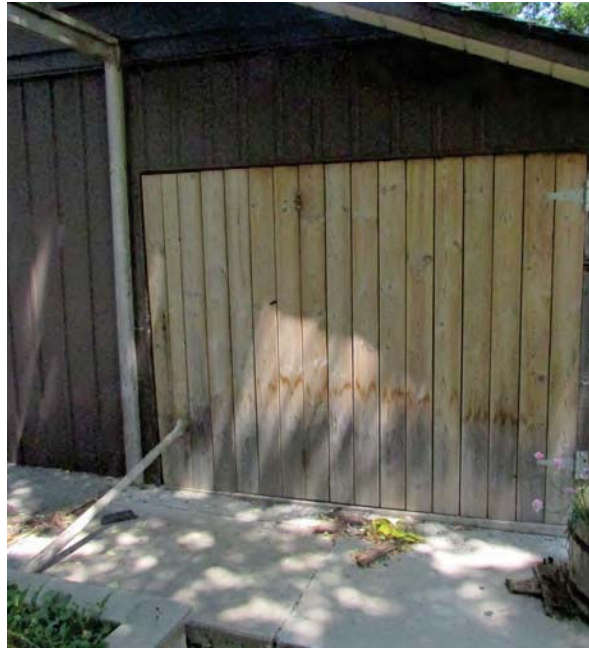
102. Unfinished door. Note stick used to keep door shut (West elevation)
