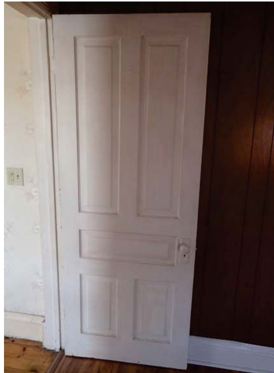
54. Good condition of door in 1911 section of house.
