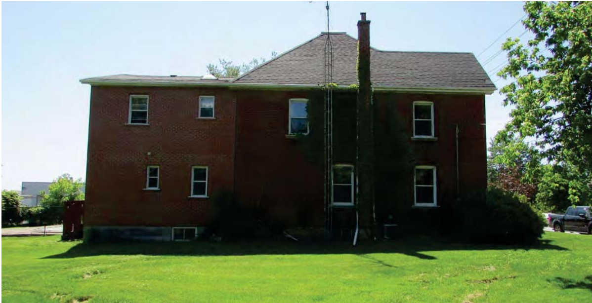
3. The north elevation of 2467 Old Bronte Road, 2017 (Source: ERA Architects)
