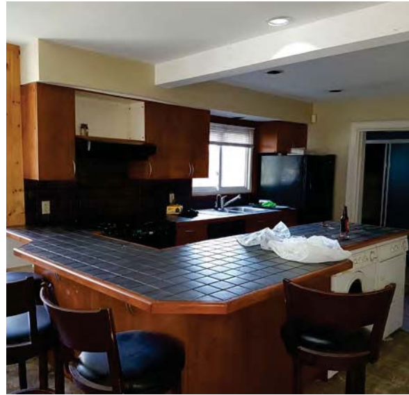
77. Fair condition of kitchen in 1860s section of the house.
