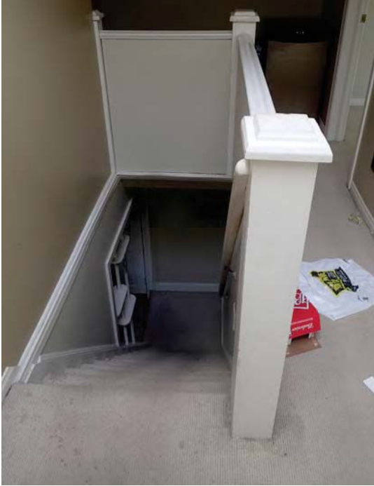
84. Good condition of stairs in 1860s section of the house.
