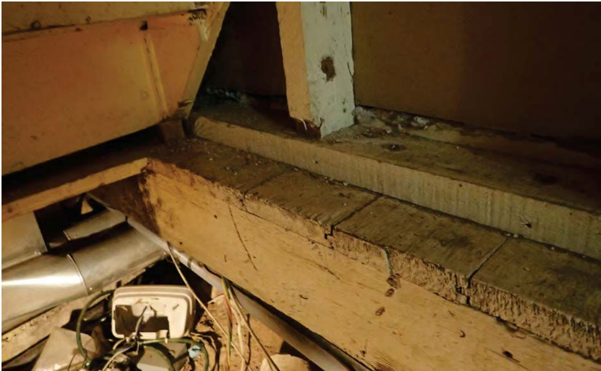
94. Joist and floorboards to 1860s house.
