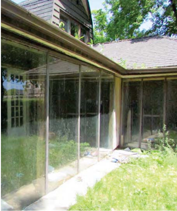
101. Full height windows (South and West elevation)
