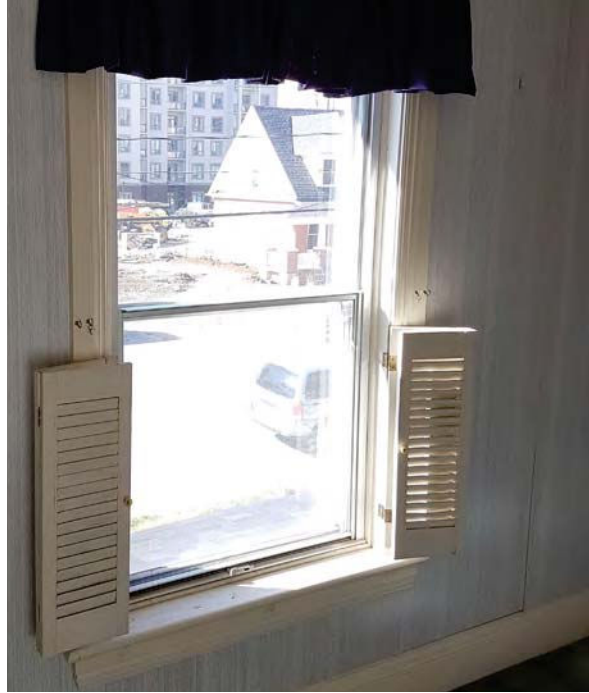
56. Good condition of window frame in 1911 section of house.
