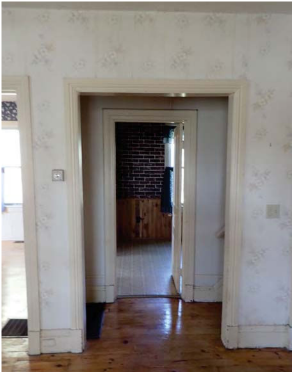
53. Good condition of door frames in 1911 section of house.
