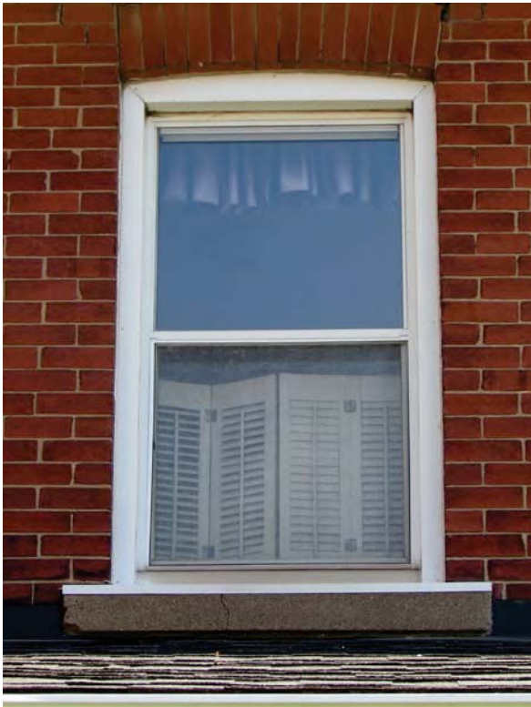
41. Example of condition of metal framed window (West elevation)
