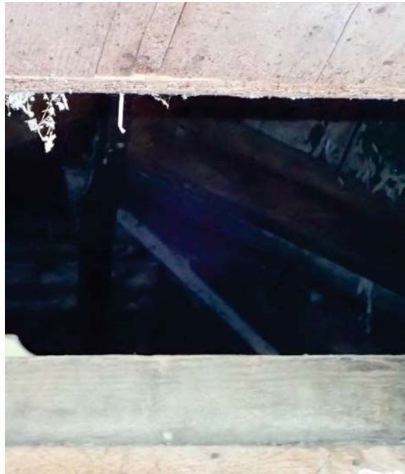
130. Partial view of roof space through open loft hatch.
