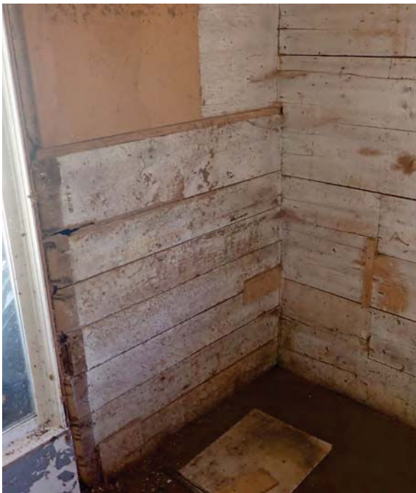
121. White washed planks in area labelled as 'the office'.
