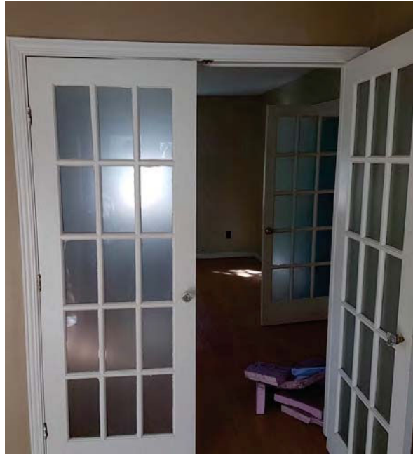
81. Good condition of possible early 20th century doors and door frame.
