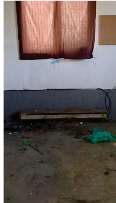
109. Fair to poor condition of walls and flooring in Northern extension.
