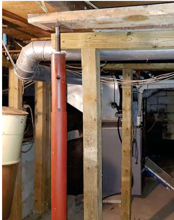
91. Supports to flooring in basement underneath 1860s section of the house.
