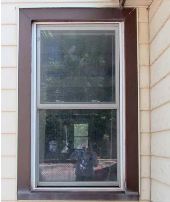
69. Example of metal framed window.
