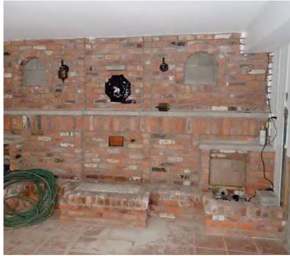
85. Fair condition of 1980s basement.
