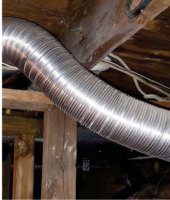
93. Floor joist and flooring to 1860s house.
