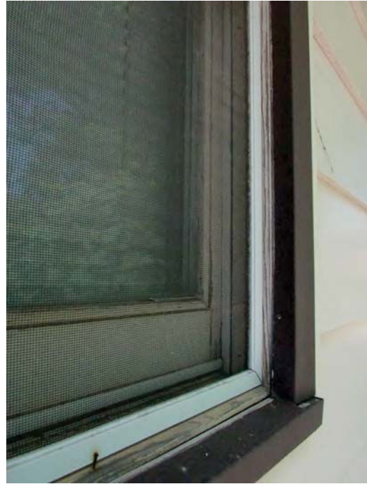
70. Timber sash with storm window.
