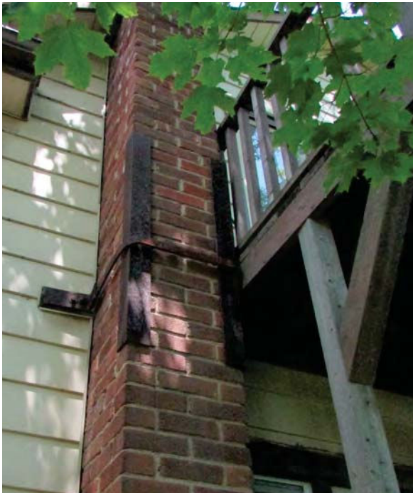
67. Bracing support for chimney
