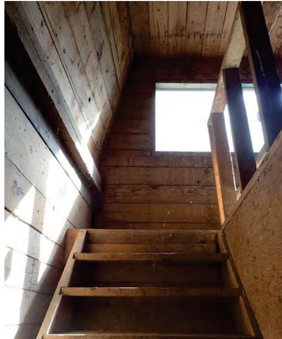
124. Fair condition of stairs to second floor.
