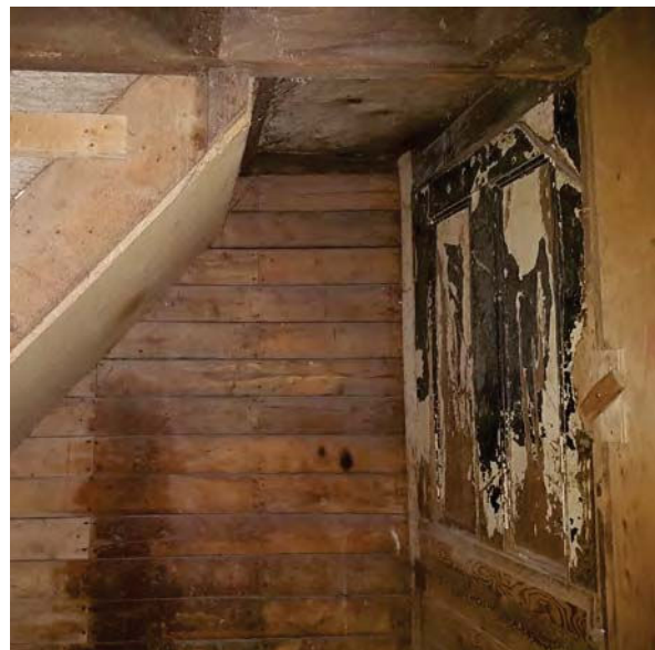
118. Timber planks as panelling underneath stairs.
