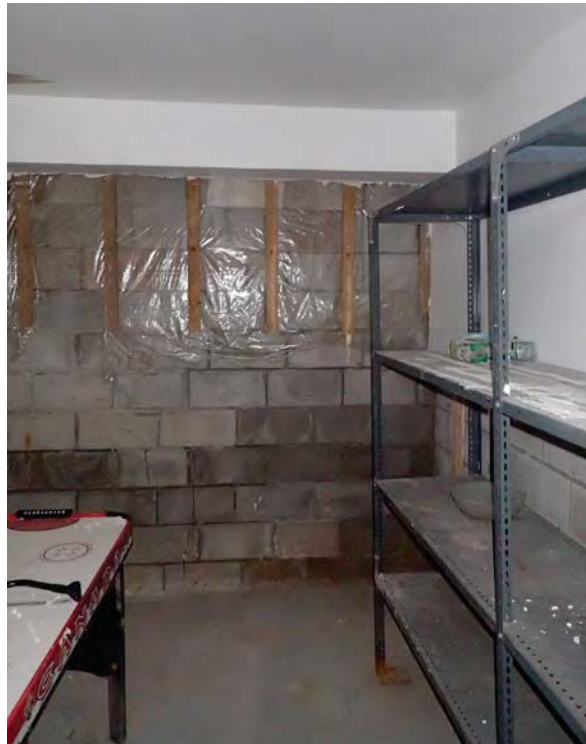
87. Concrete blockwork in 1980s basement.
