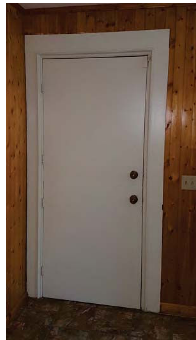
75. Good condition of door and frame on first floor.
