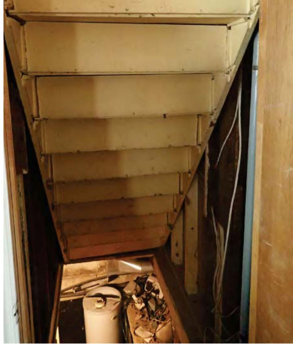
89. Stairs down to basement underneath 1860s section of the house.
