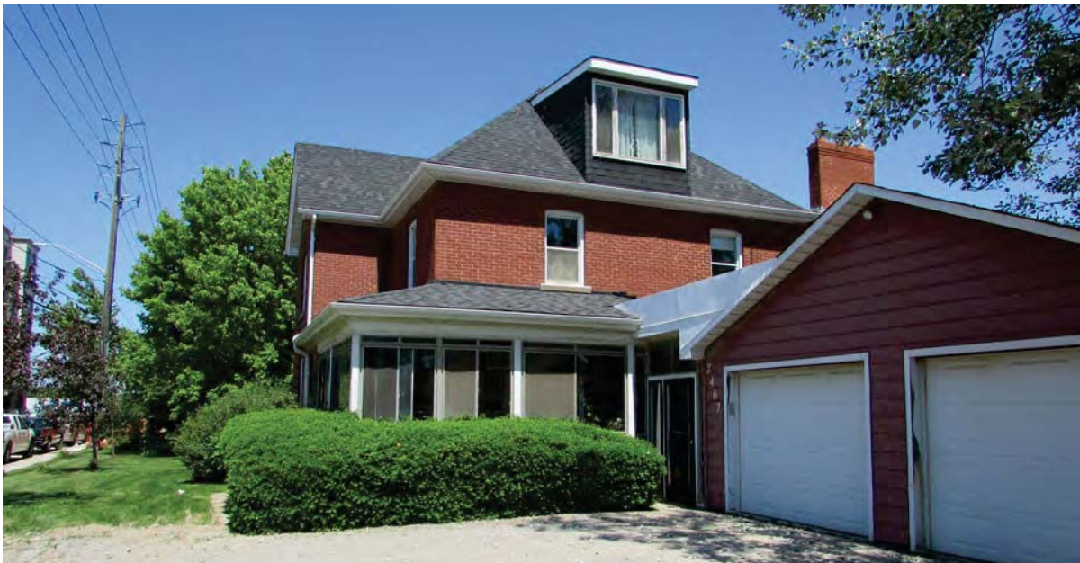
5. The south elevation of 2467 Old Bronte Road, 2017 (Source: ERA Architects)
