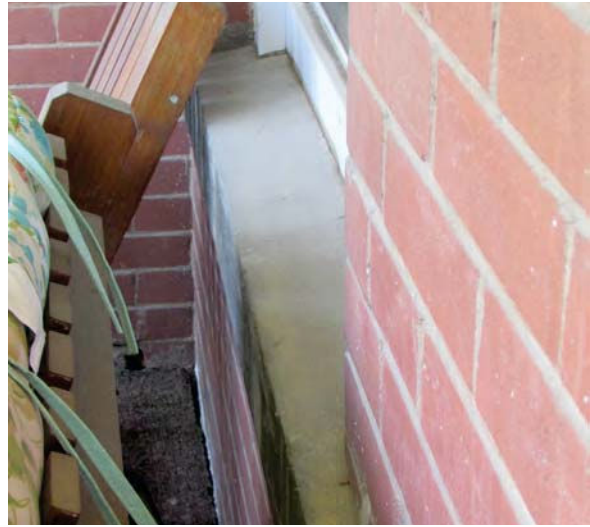
44. Good condition of stone sill (West elevation).
