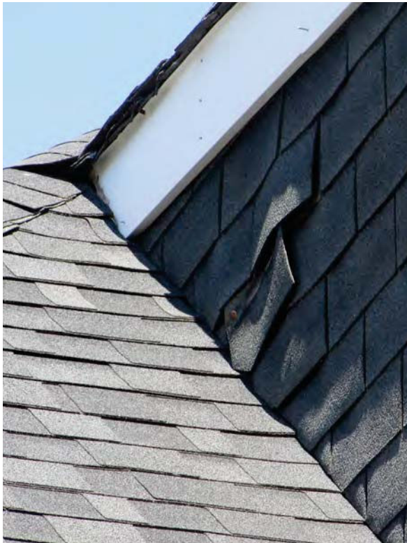
45. Lifting shingles on dormer extension.
