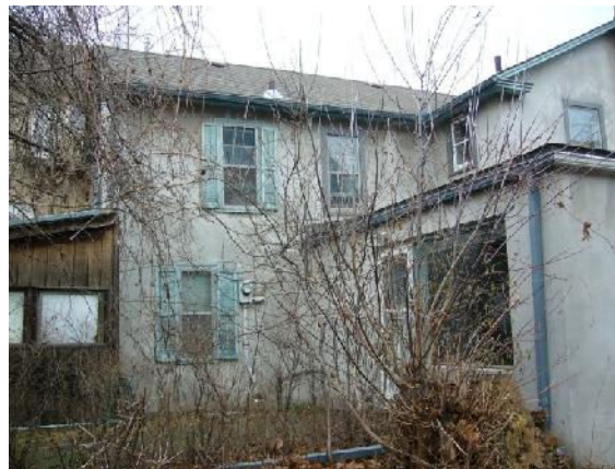
Rear façades of main building and addition (foreground), January 18, 2017.
