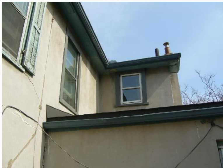
Upper floor (south) façade
