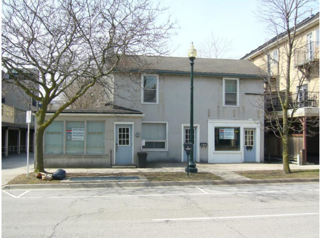
Front (east) facade of 132-136 Dunn Street (April 10, 2017)
