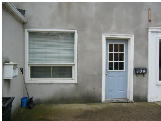
Window and door alterations (134 Dunn Street), January 18, 2017.
