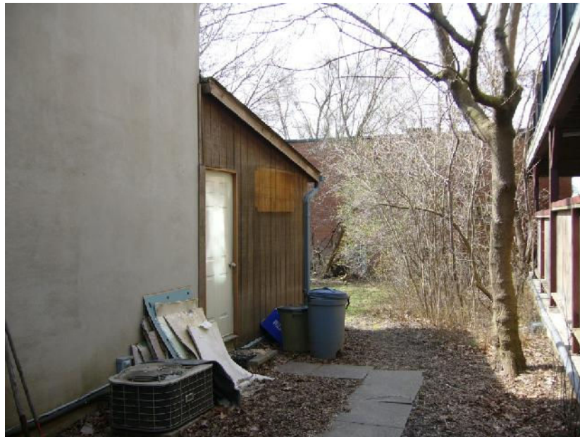
Side (north) facade
