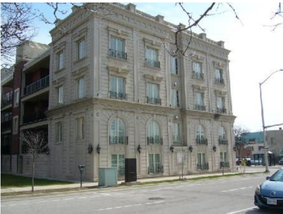
Rear of 253 Church Street (April 10, 2017)
