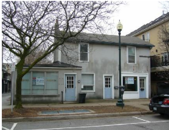
Front (east) façade with cementitious render, synthetic doors and windows, January 18, 2017.
