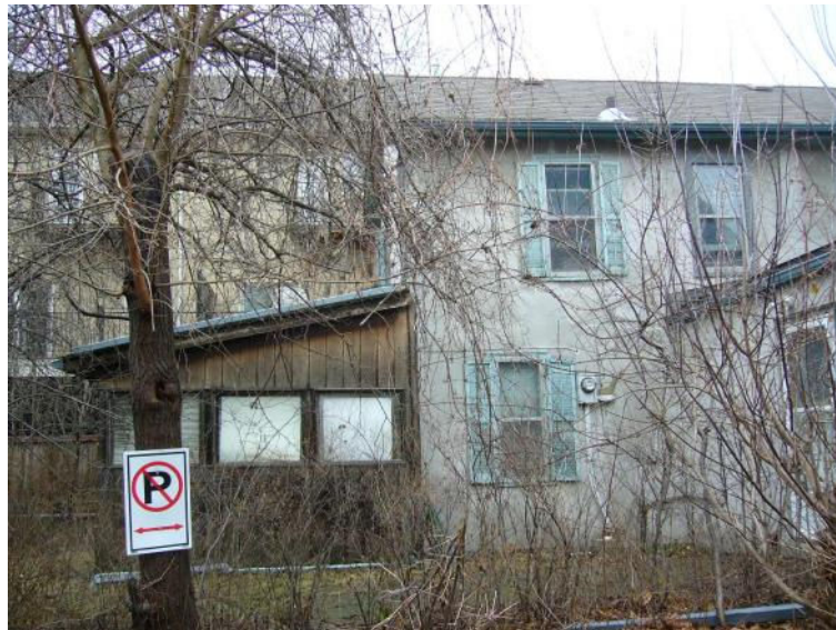
The rear (west) addition and side (south) facade
