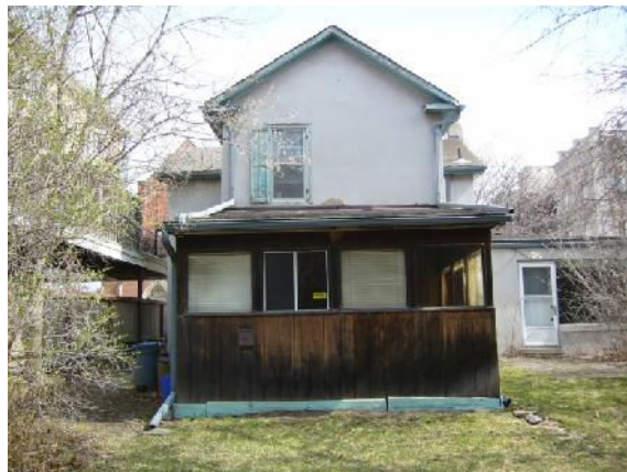
West façade with timber clad, rear lean-to addition, April 10, 2017
