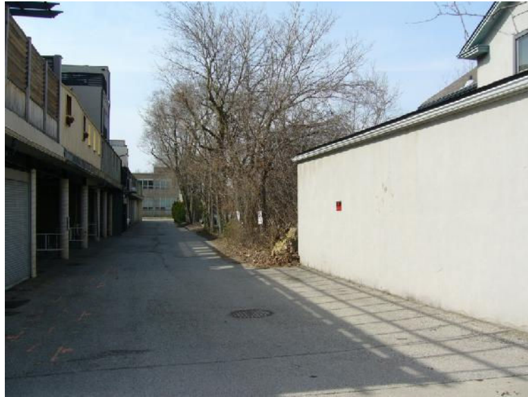
Ground floor side (south) façade
