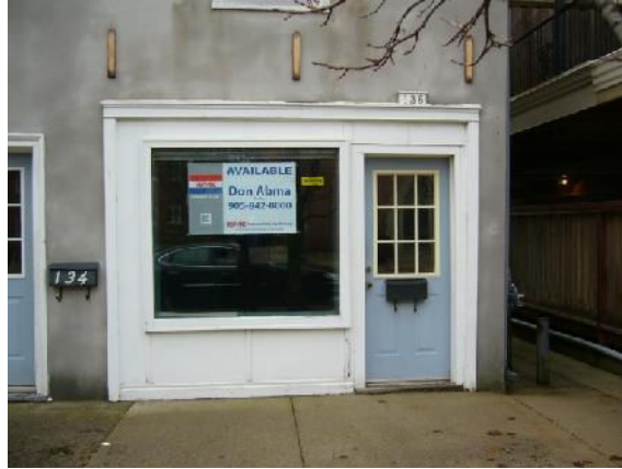
Shopfront and door alterations (136 Dunn Street) January 18, 2017.
