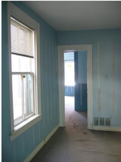
Interior at north side looking east to front façade of 136 Dunn Street, April 10, 2017
