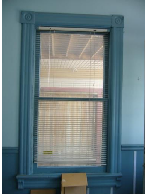
Interior window on north façade of 136 Dunn Street, April 10, 2017
