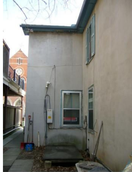
Side (north) facade
