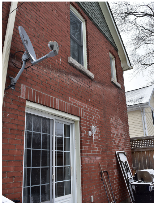
Rear elevation with ghost lines and brick repairs.
