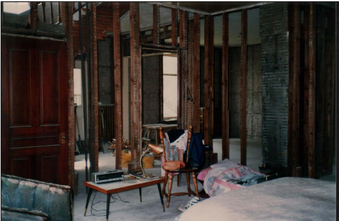
Figure 46: Interior renovation of the main level showing the exposed lath and plaster (C. Schulz, 2016).
