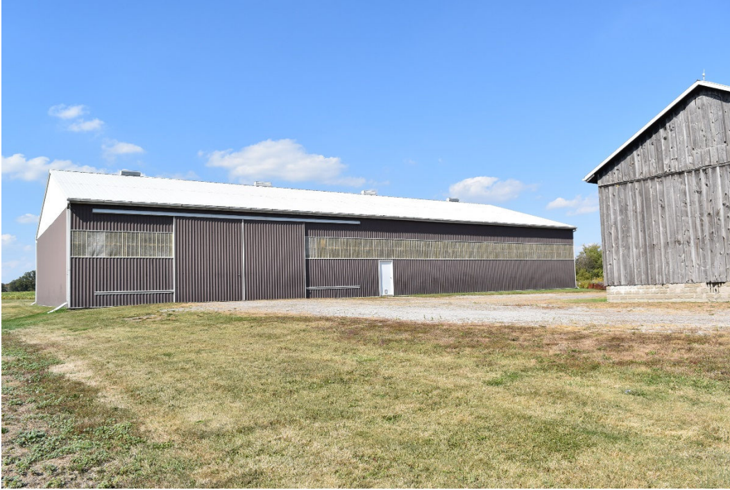
1984 drive shed, south façade
