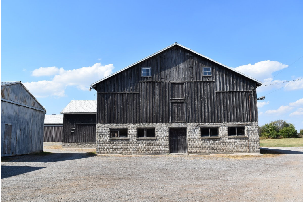
Connected barn front (south) façade
