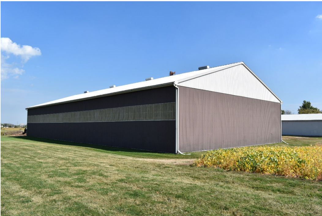
1984 drive shed, northwest corner
