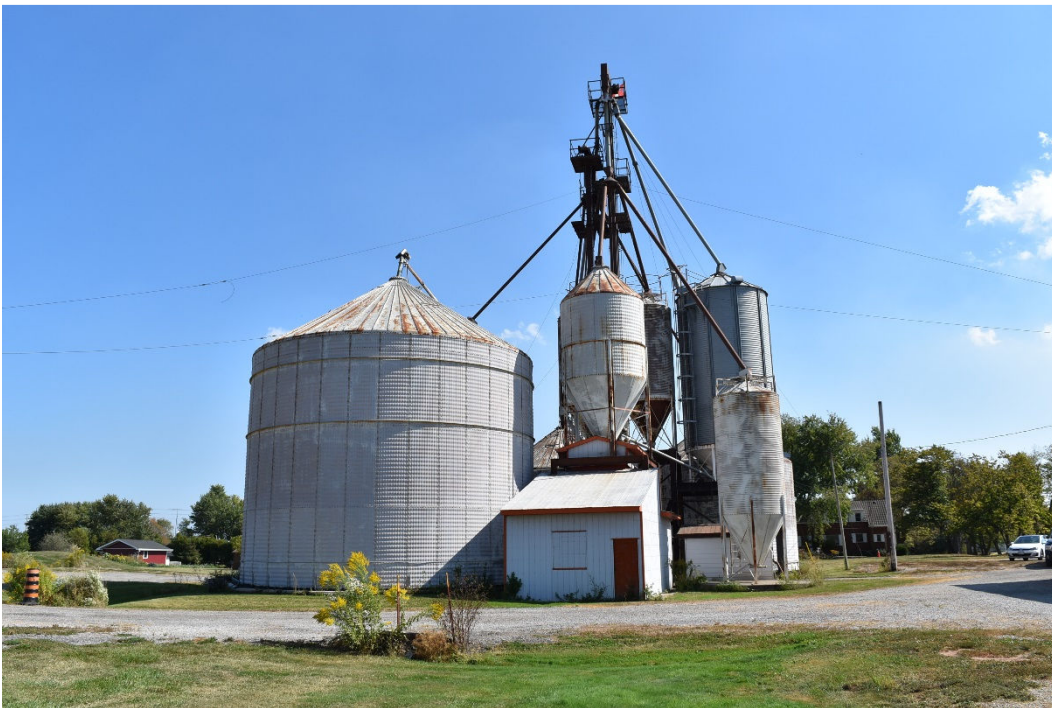
Silos, north facade
