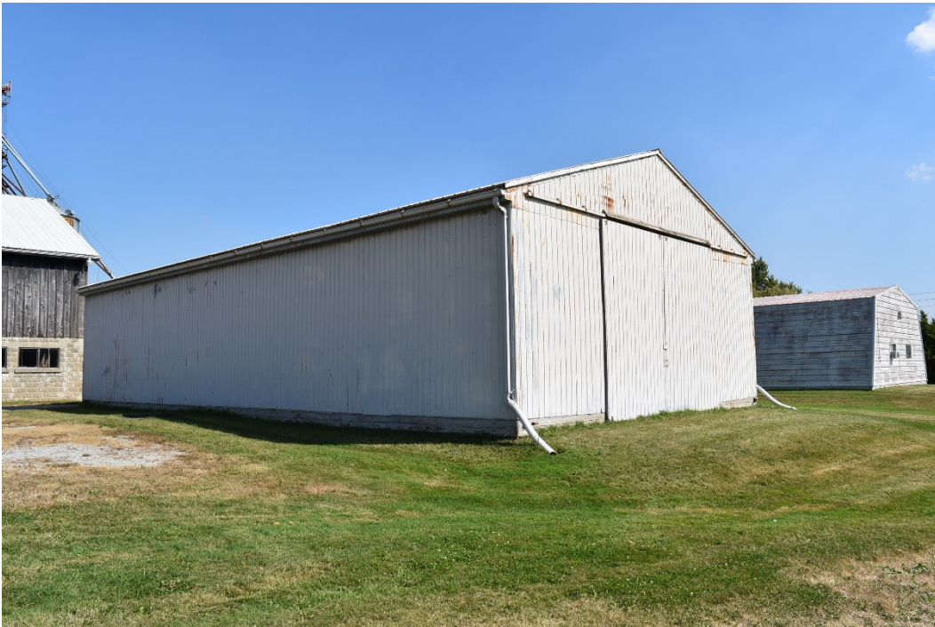
1960s sheds, northwest corners
