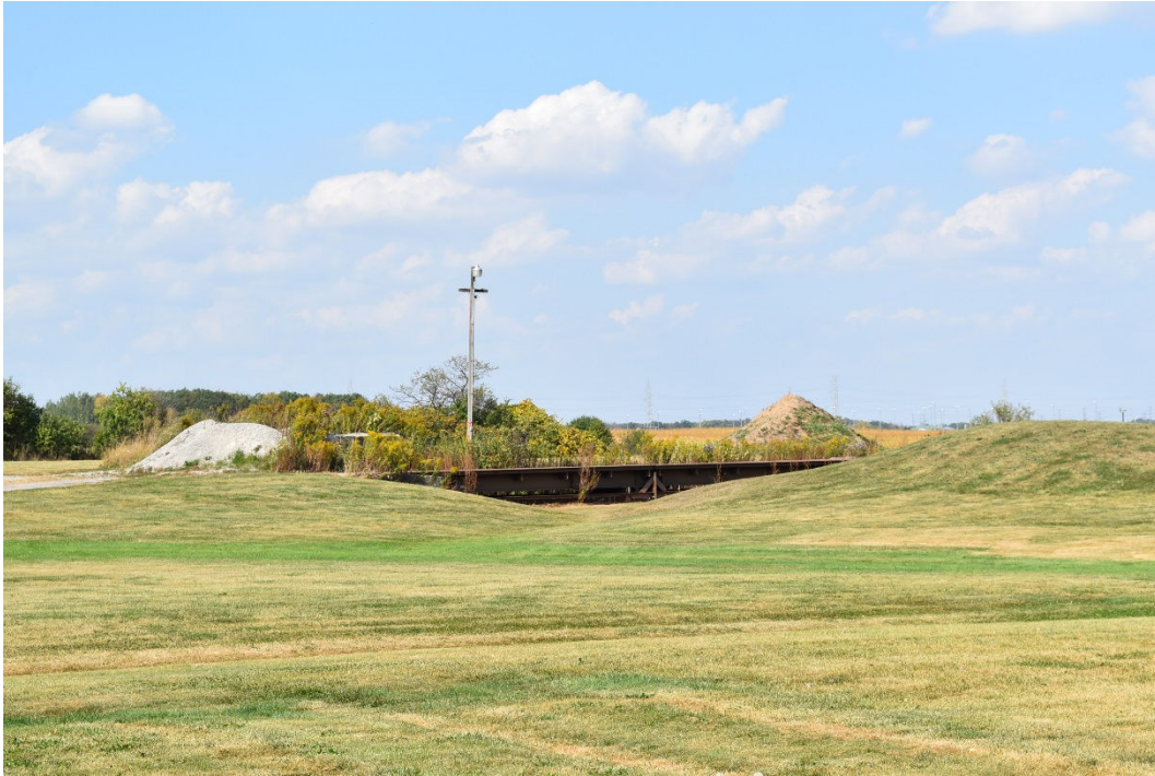
Grain truck weighing platform south facade
