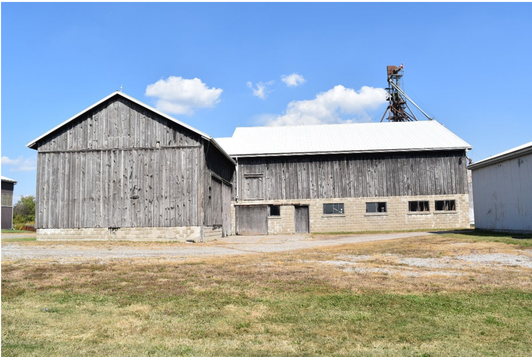
Connected barn west façade
