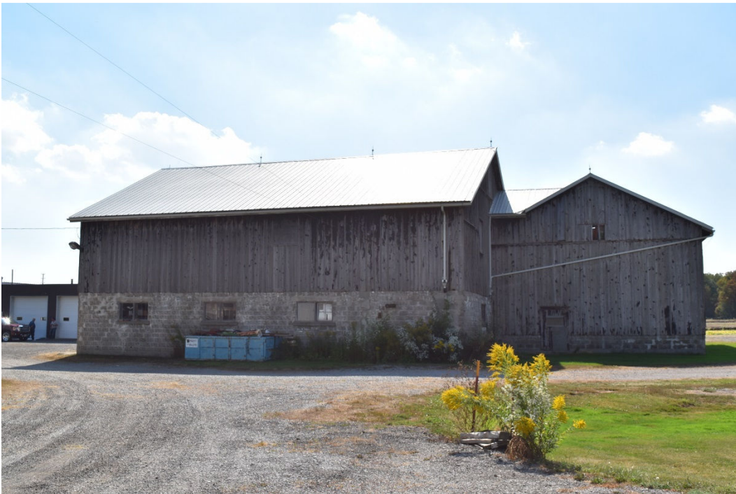
Connected barn east façade
