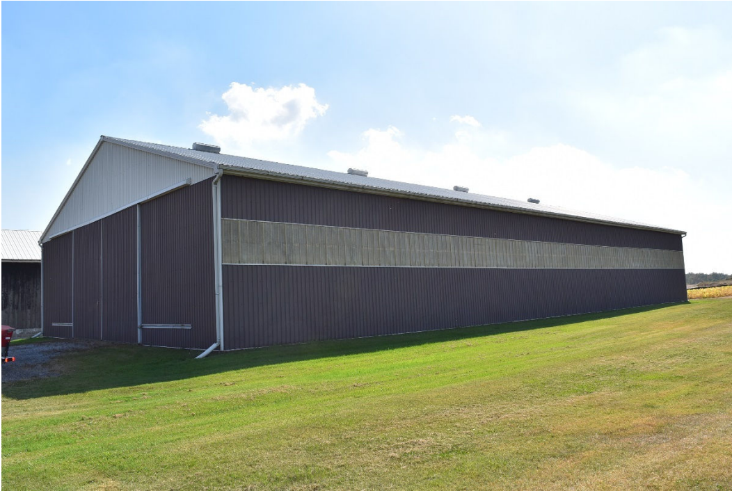
1984 drive shed, northeast corner
