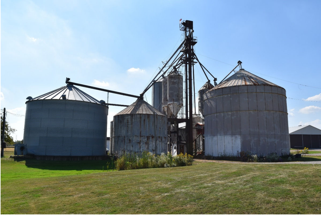
Silos, east facade
