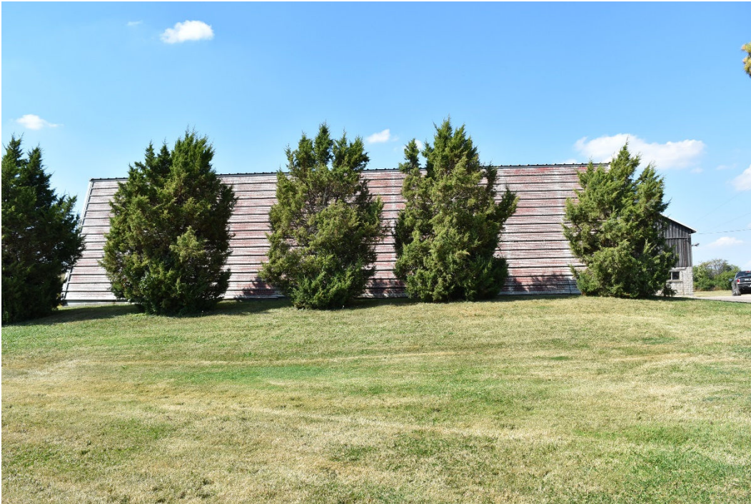
South most shed, south façade
