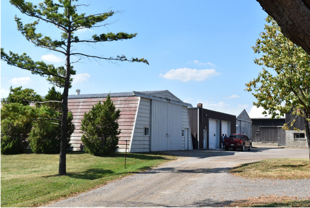
Three 1960s sheds southeast corners
