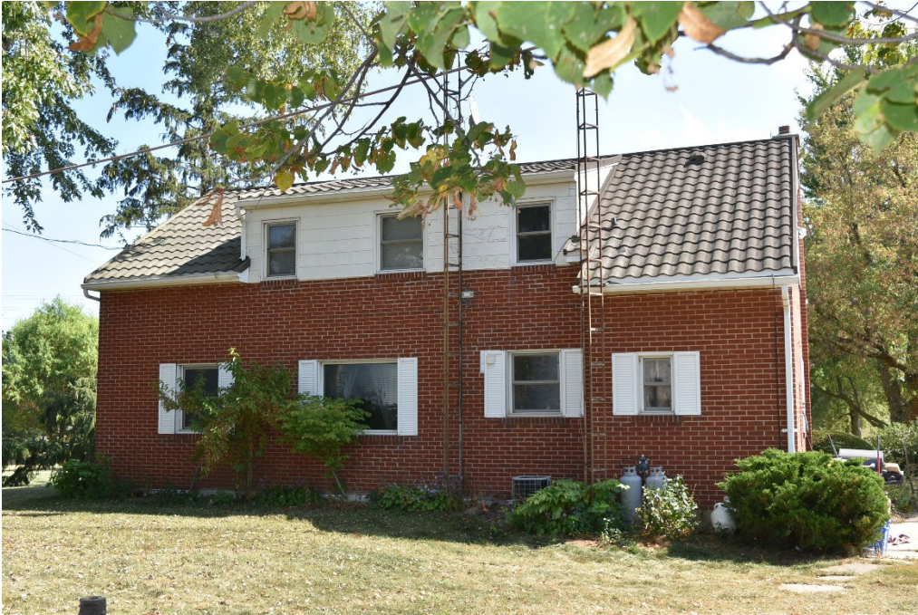
Farmhouse rear (north) facade
