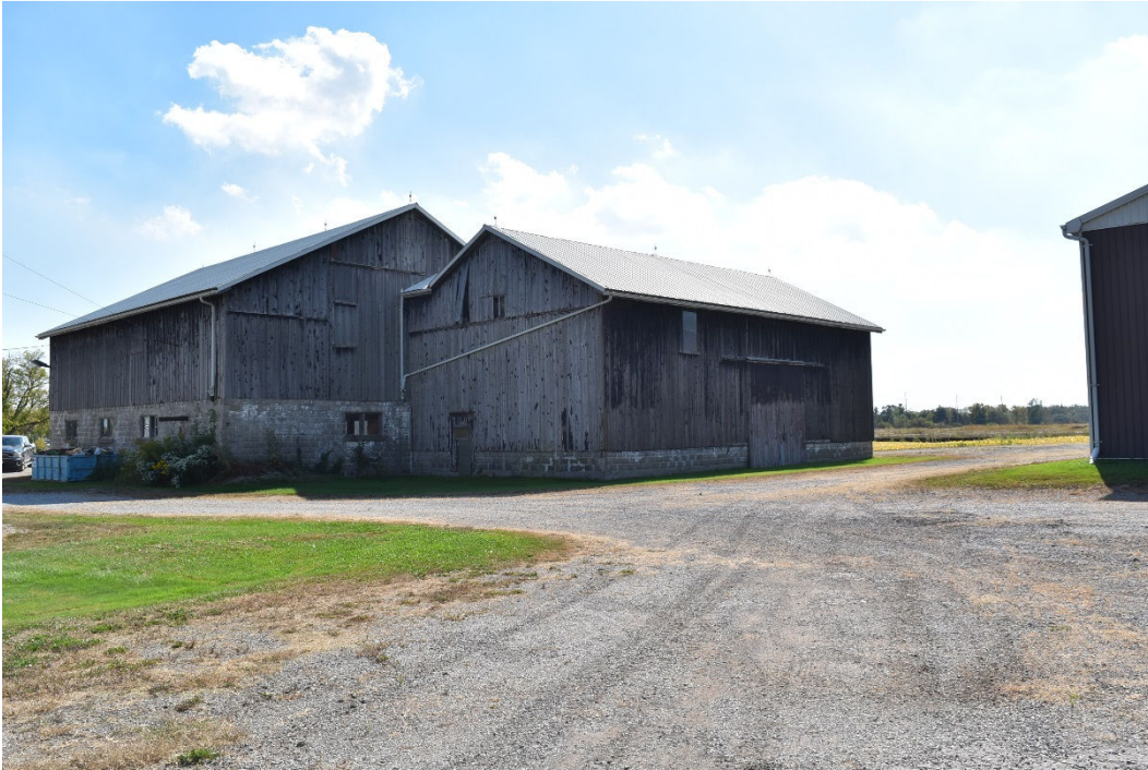
Connected barn northeast corner
