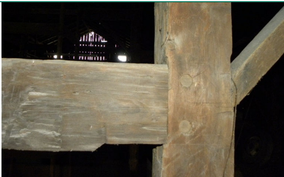
Image 28. Detail of beam joinery in the barn with visible treenails.
