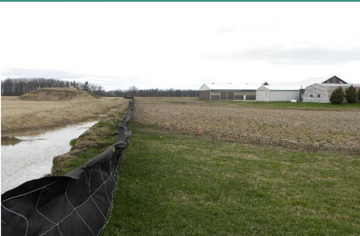
Image 7. Silt fencing along the east edge of the Study Area, view facing northwest.
