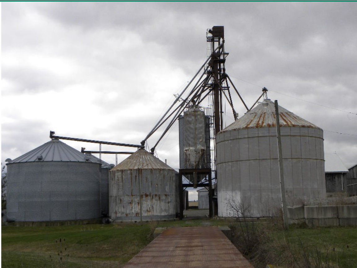
Image 37. Silo complex with two smaller grain bins on the left, three hopper tanks in a line in the centre and the largest grain bin on the right, view southwest.
