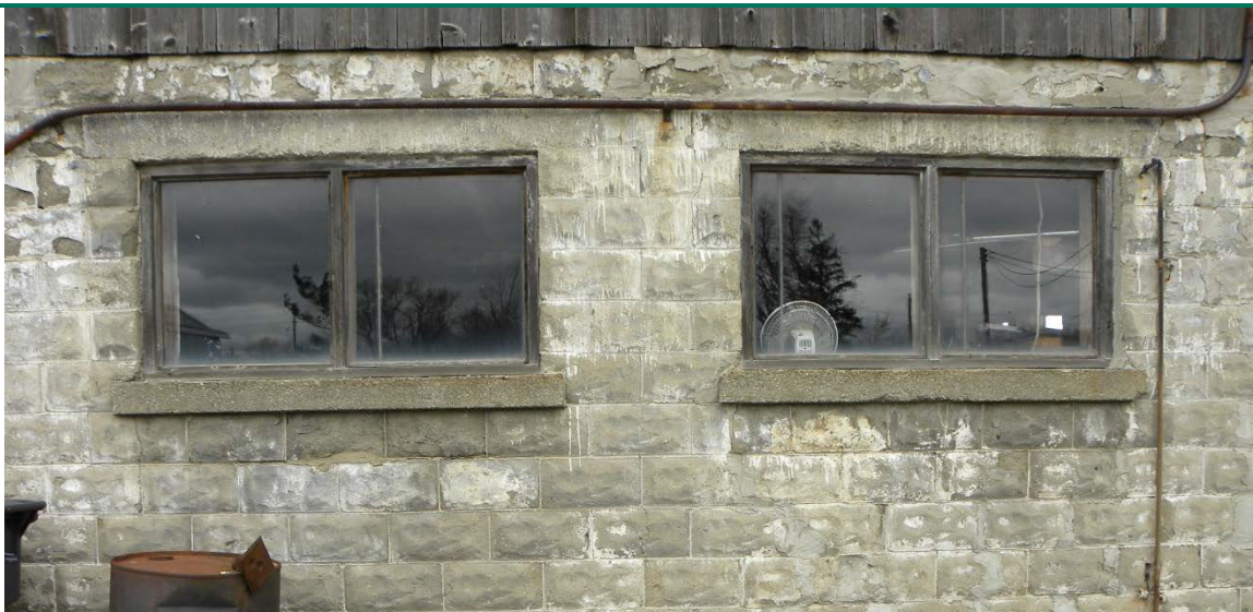
Image 21. Wooden frame windows with concrete sills on southeast elevation of the barn, view northwest.
