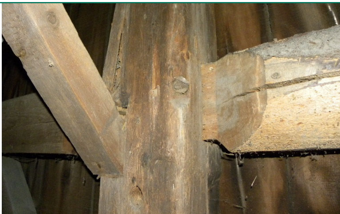
Image 27. Detail of beam joinery in the barn.
