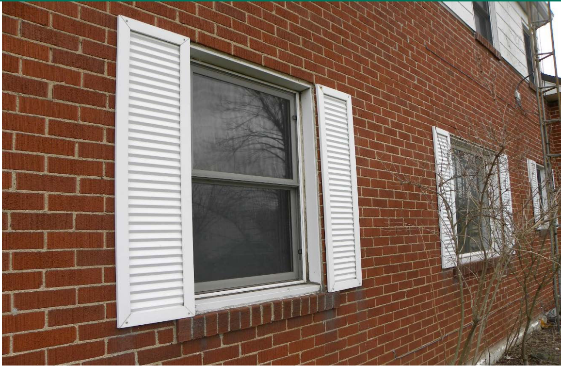
Image 14. Metal double hung windows with rowlock brick sill on the back of the house.
