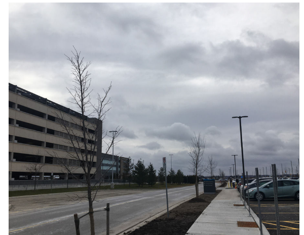
Structured and surface parking, looking west along William Halton Parkway West
