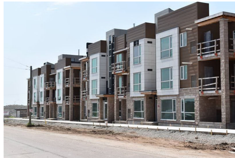
Image: New townhouses under construction on Khalsa Gate
