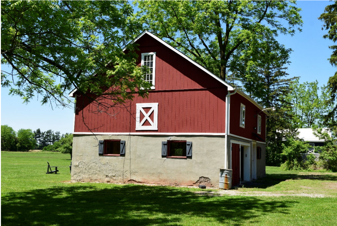
Image 40: South facade of outbuilding, red siding is modern
