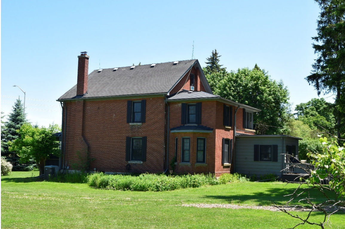
Image 5: Northwest facade, note bay window on c. 1920 addition, facing southeast
