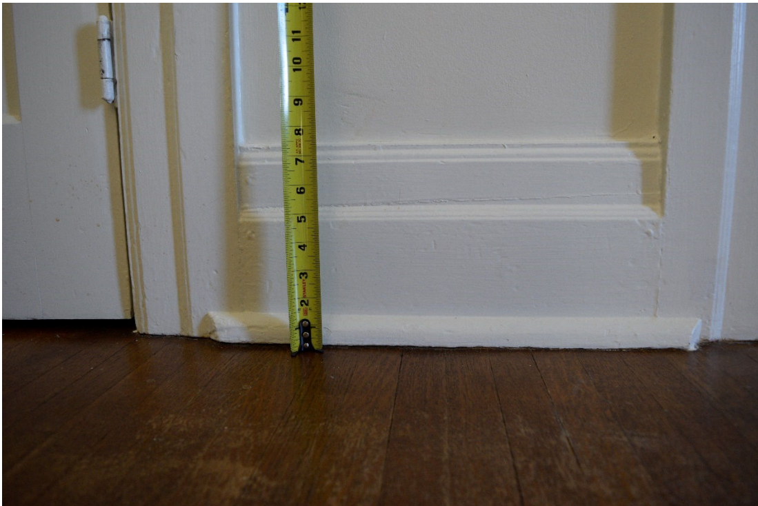
Image 34: Typical door trim and baseboard, original oak floors visible
