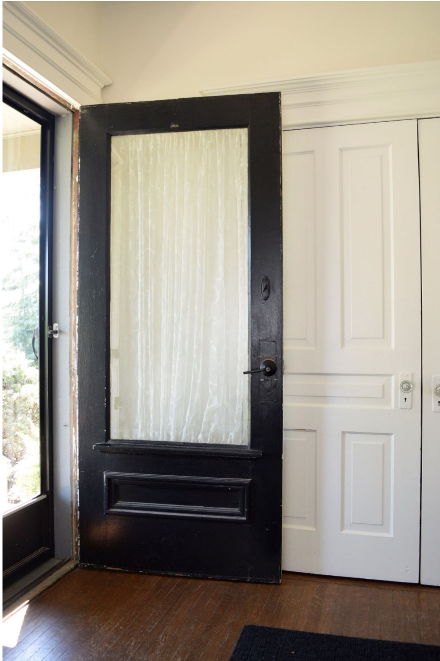
Image 11: Original front door, note original doorbell hardware
