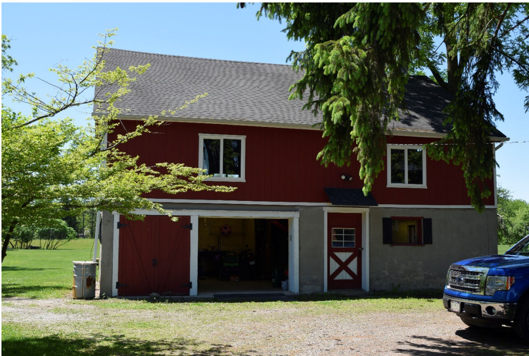
Image 39: East facade of outbuilding, doors and windows are modern, facing west
