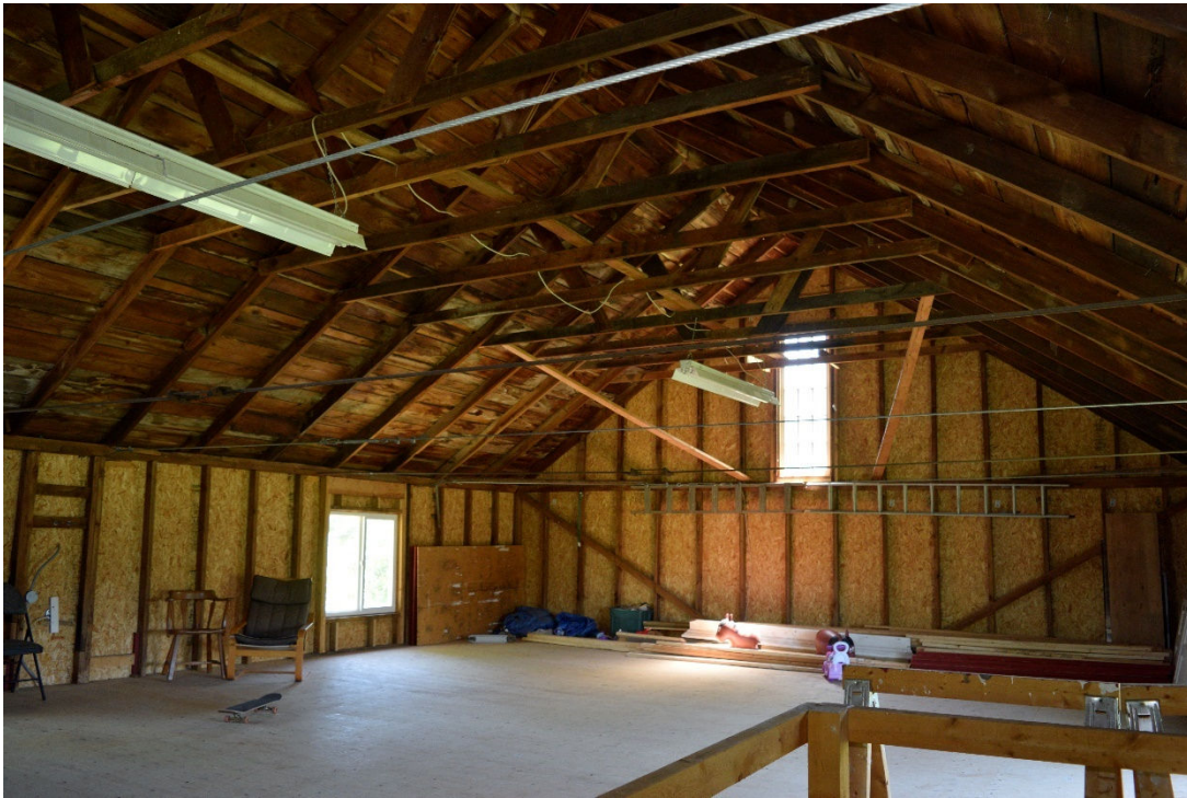
Image 44: Interior of stick framed outbuilding, note use of contemporary particle board
