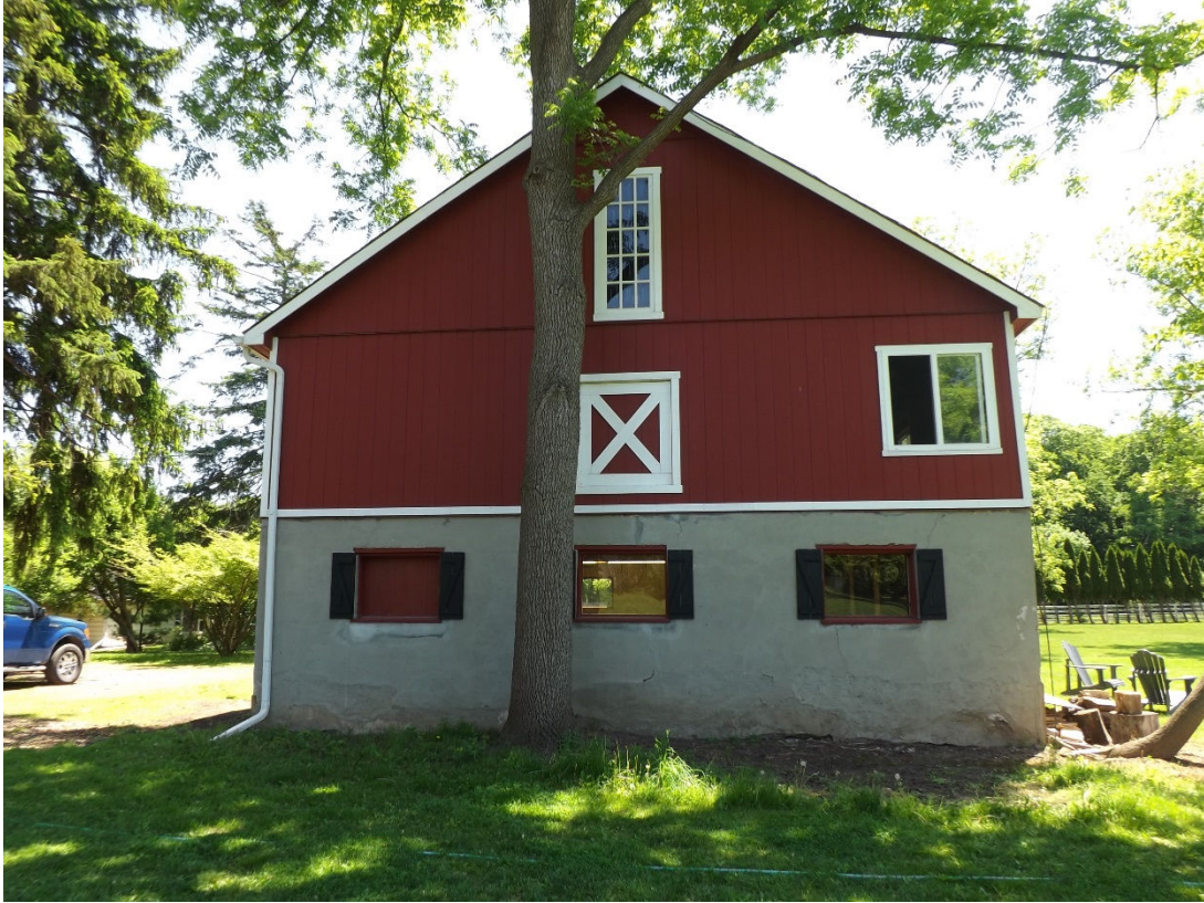
Image 42: North face of outbuilding, facing south
