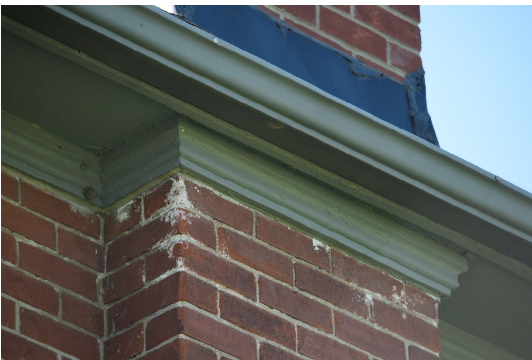
Image 8: Typical moulded freeze under eaves
