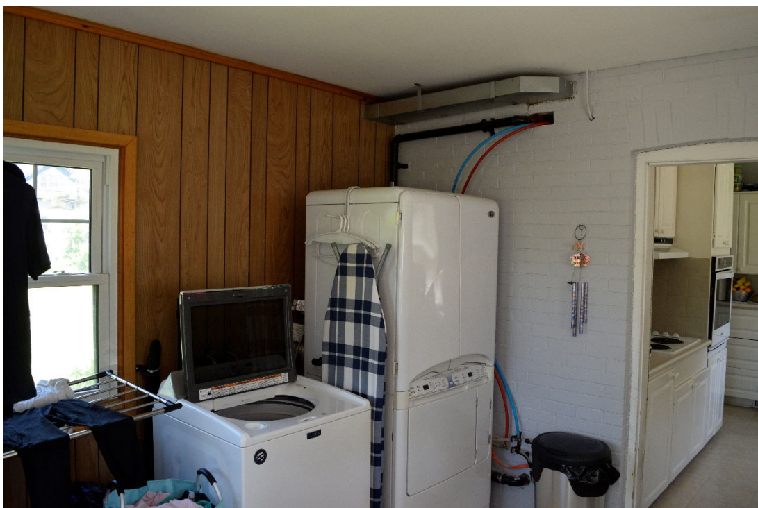
Image 21: Interior of c.1950 addition, note original exterior wall of c.1920 addition
