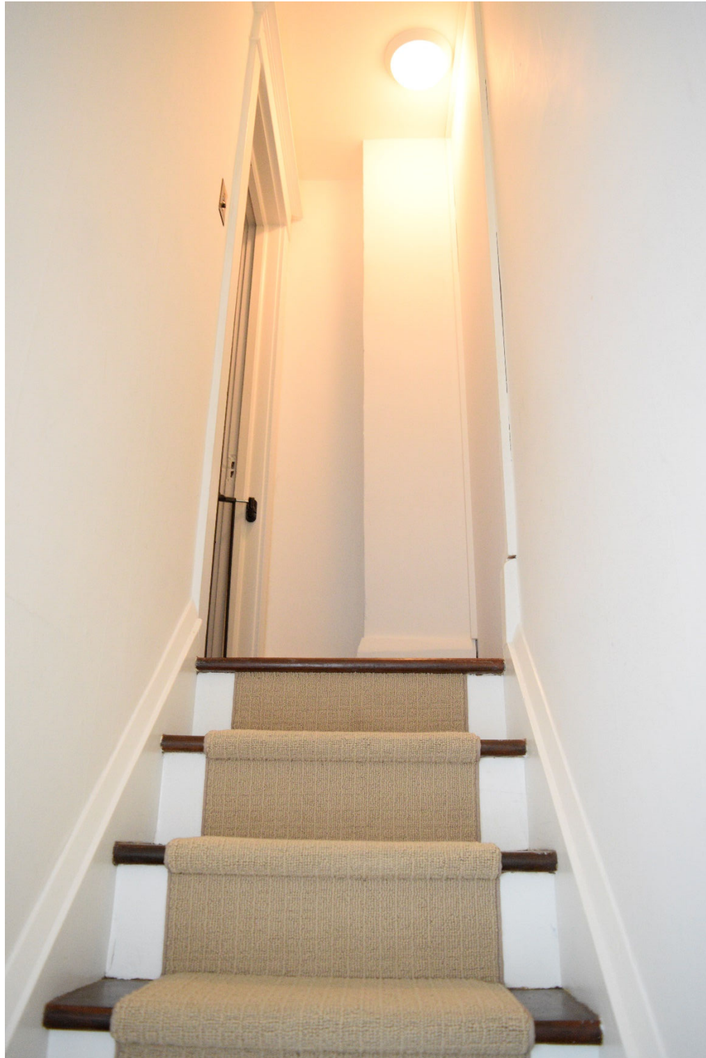
Image 23: Narrow stairs in c.1920 addition
