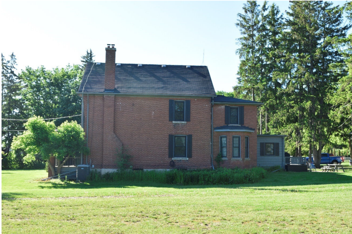
Image 3: North facade of residence, facing south
