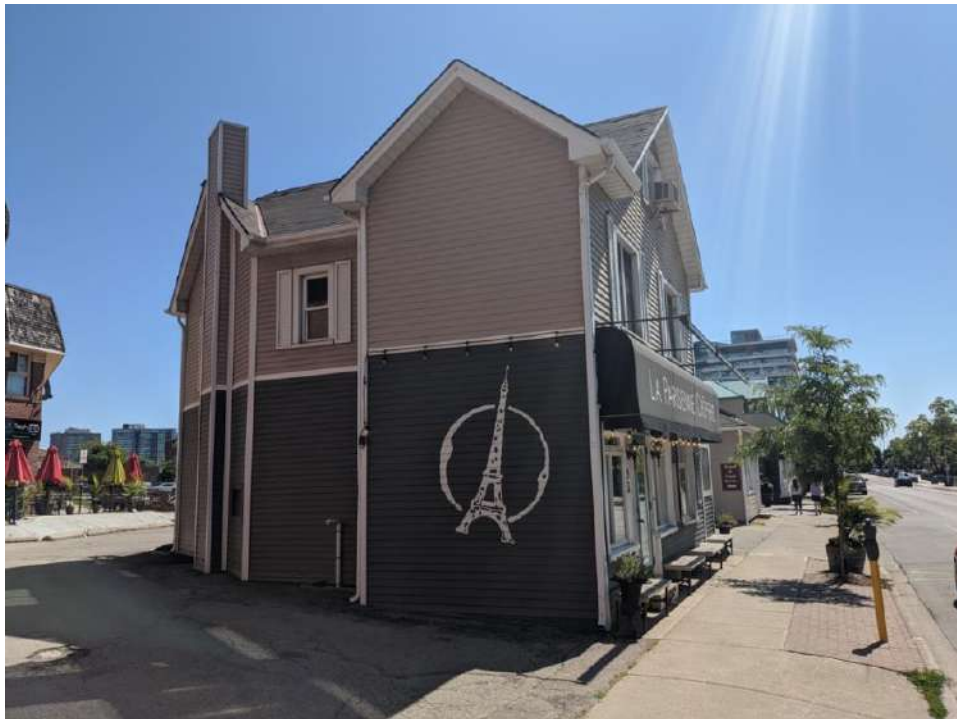
Figure 35: South and west façades of 93 Bronte Road
