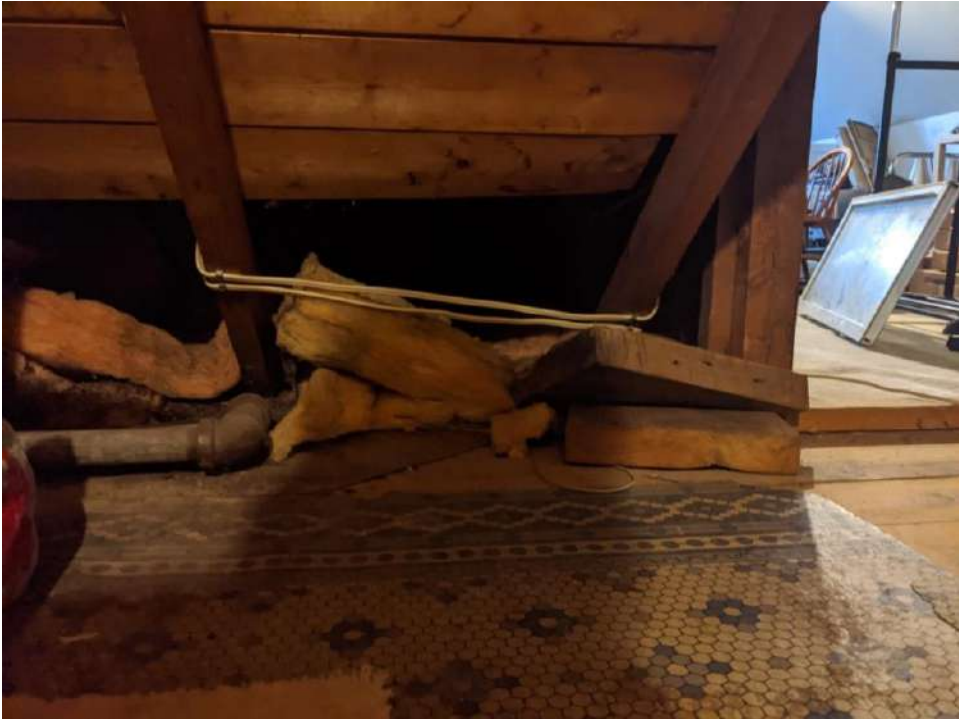
Figure 63: Attic beams supported by bungee cord
