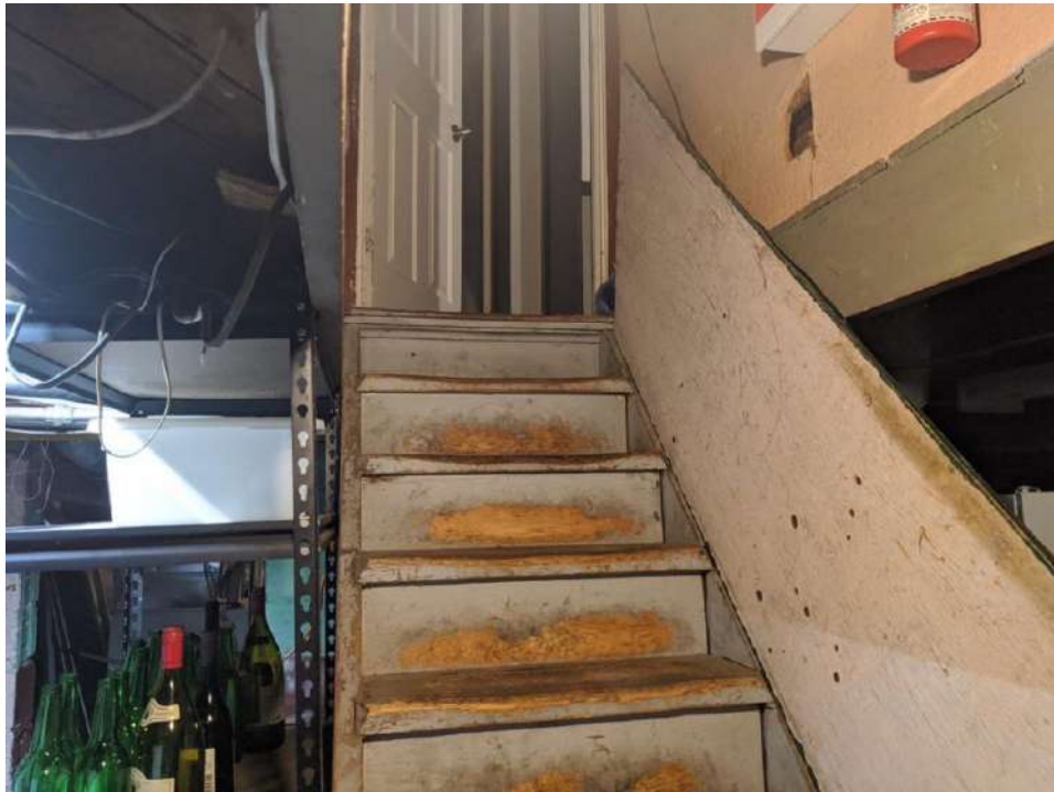
Figure 59: Stairs leading from the main floor to the basement
