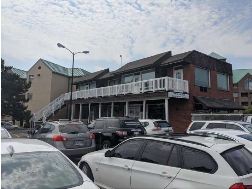
Figure 16: North façade of 77 Bronte Road
