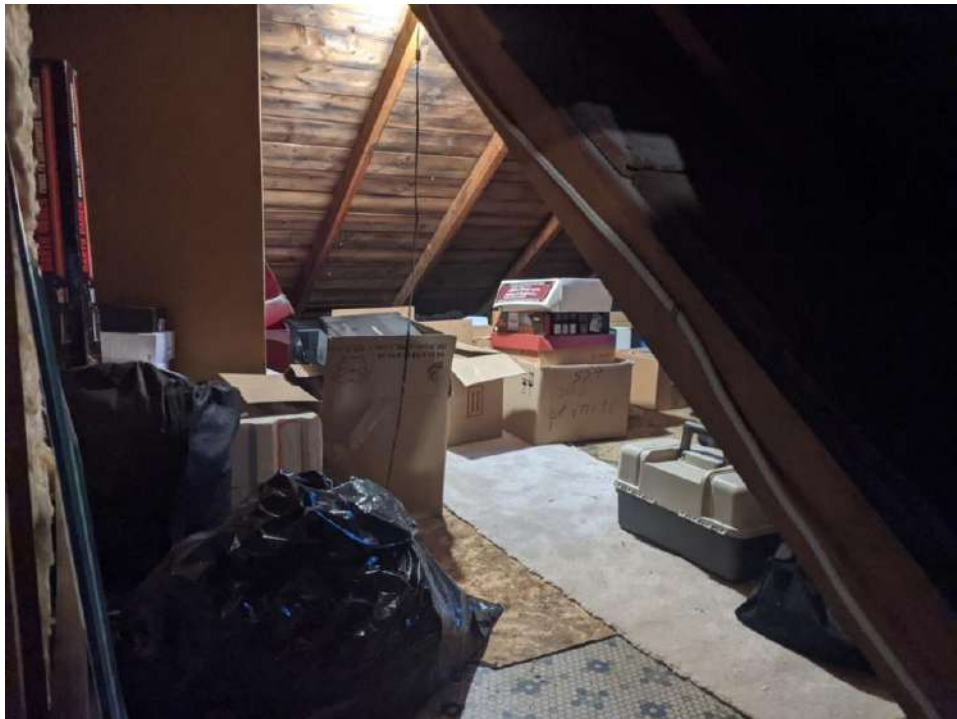
Figure 58: Crawlspace to the north
