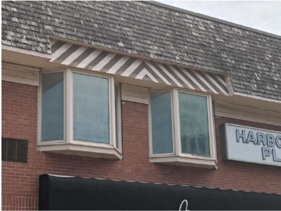
Figure 72: Mansard style roof
