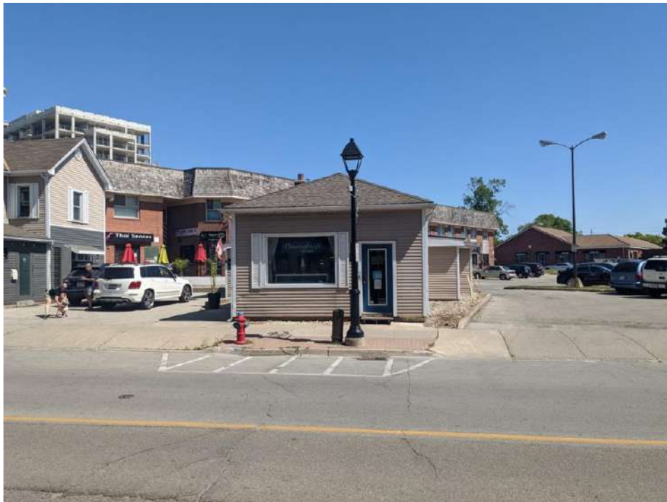
Figure 20: South façade of 87 Bronte Road
