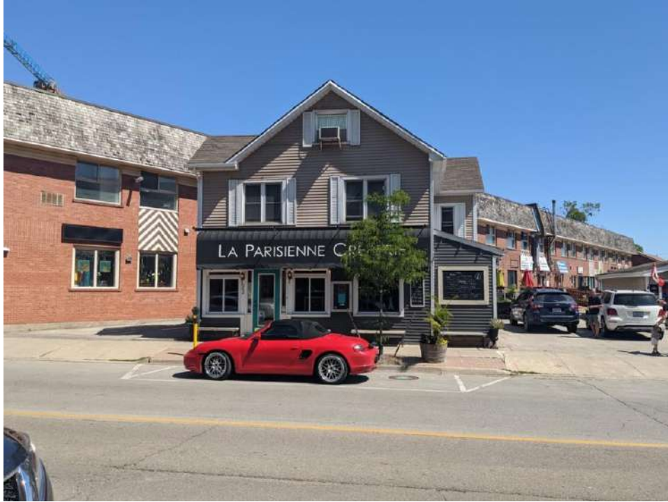
Figure 34: South façade of 93 Bronte Road
