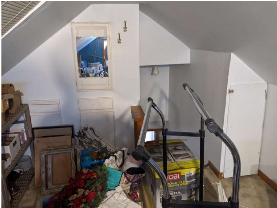
Figure 56: Attic space facing north with crawlspace to the right
