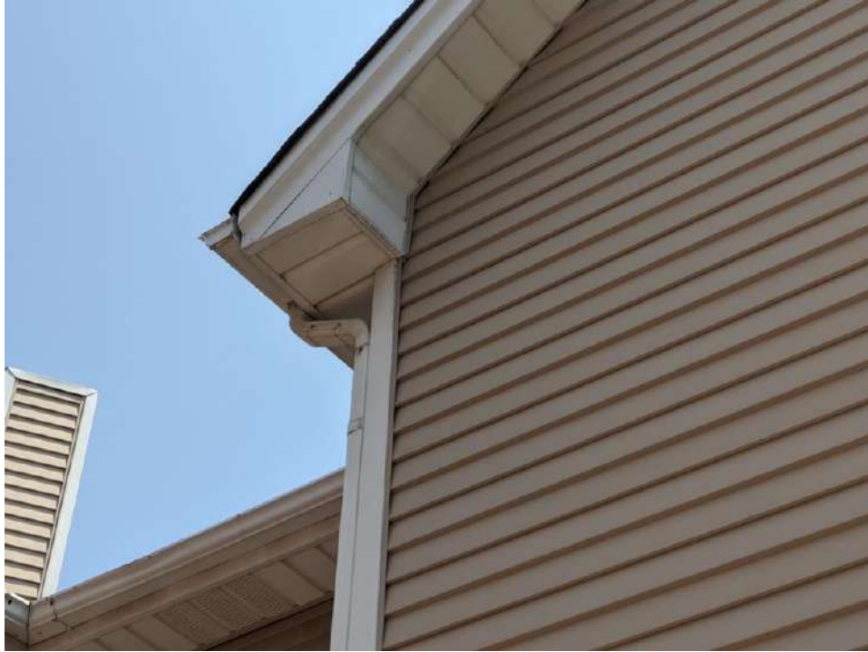
Figure 38: Vinyl soffit and eaves at west façade gable
