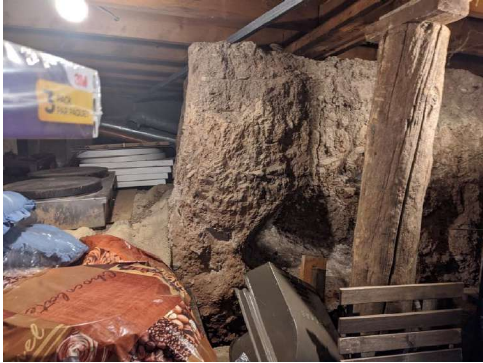
Figure 64: Dirt basement covered in cement based parging
