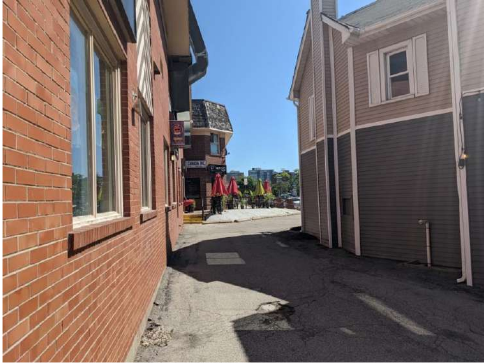
Figure 13: Paved alleyway between 2432-2452 Lakeshore Road West and 93 Bronte Road
