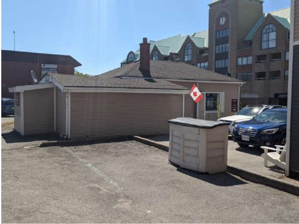
Figure 21: West façade of 87 Bronte Road
