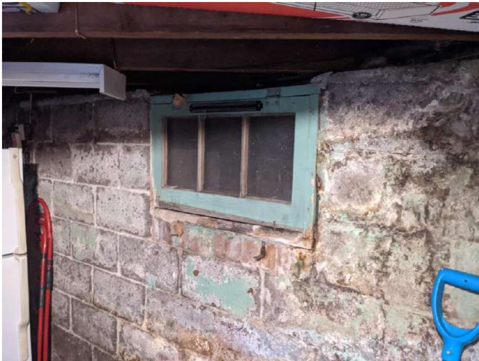
Figure 61: Basement window facing northwest
