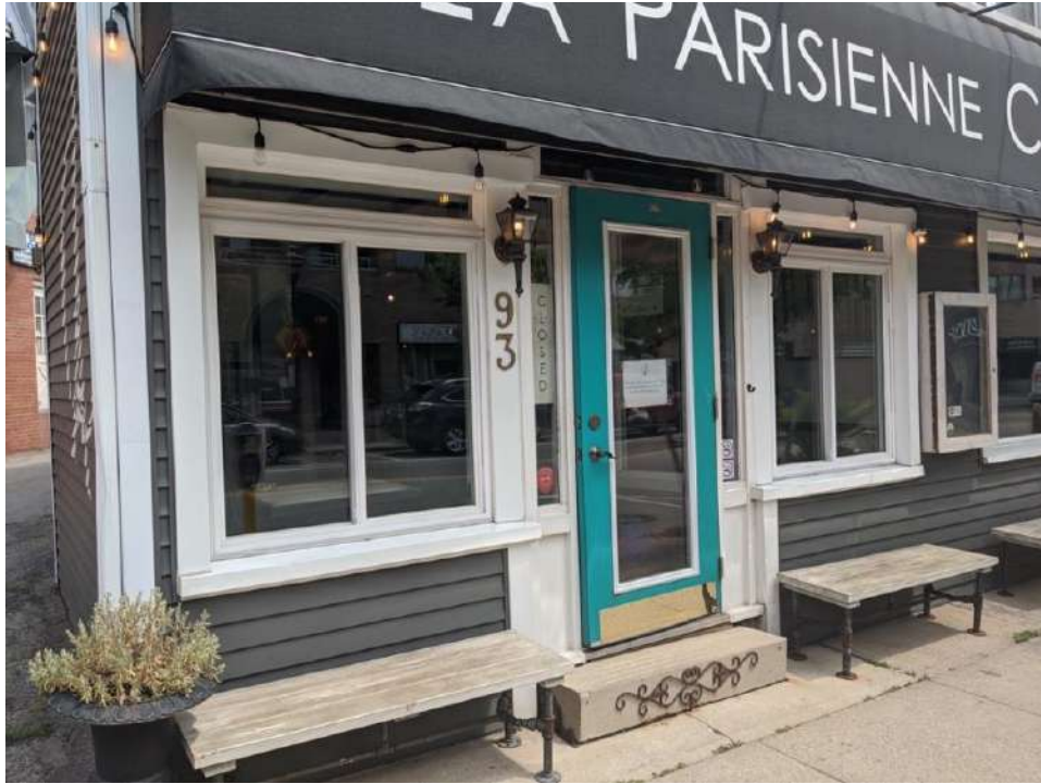
Figure 40: South façade main entrance
