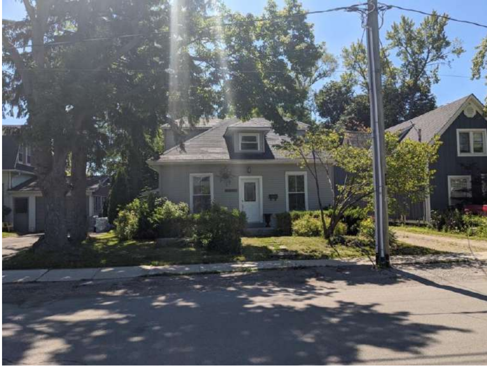
Figure 65: Listed vernacular property at 2370 Sovereign Street
