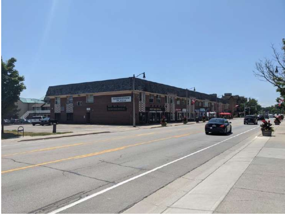
Figure 68: North and west façades of 2432-2452 Lakeshore Road West
