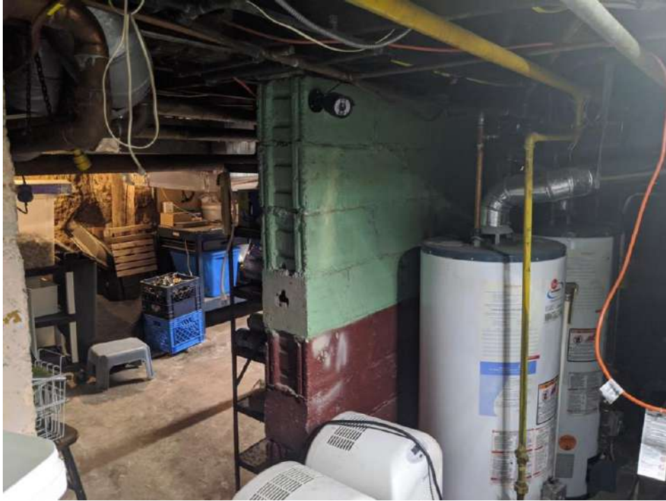
Figure 60: Basement facing southwest
