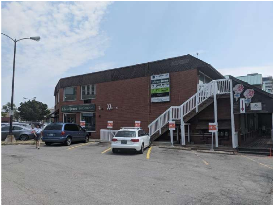
Figure 15: West façade of 77 Bronte Road
