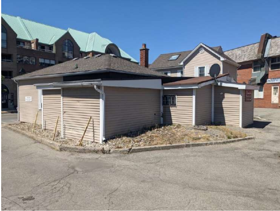
Figure 23: East façade of 87 Bronte Road, showing all four rear additions
