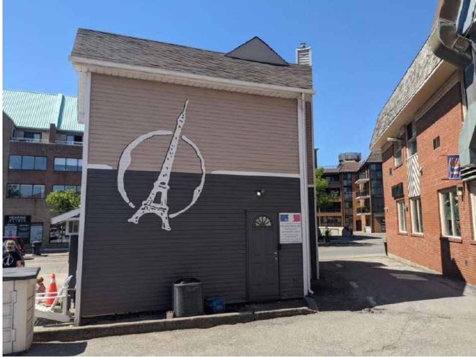
Figure 36: North façade of 93 Bronte Road
