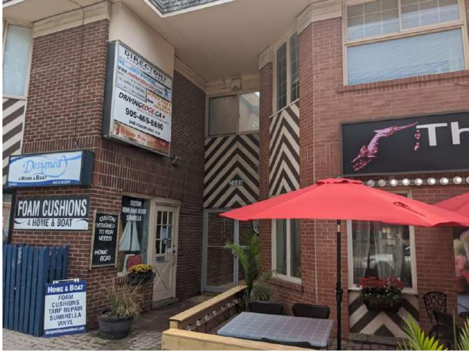
Figure 74: West façade entrance
