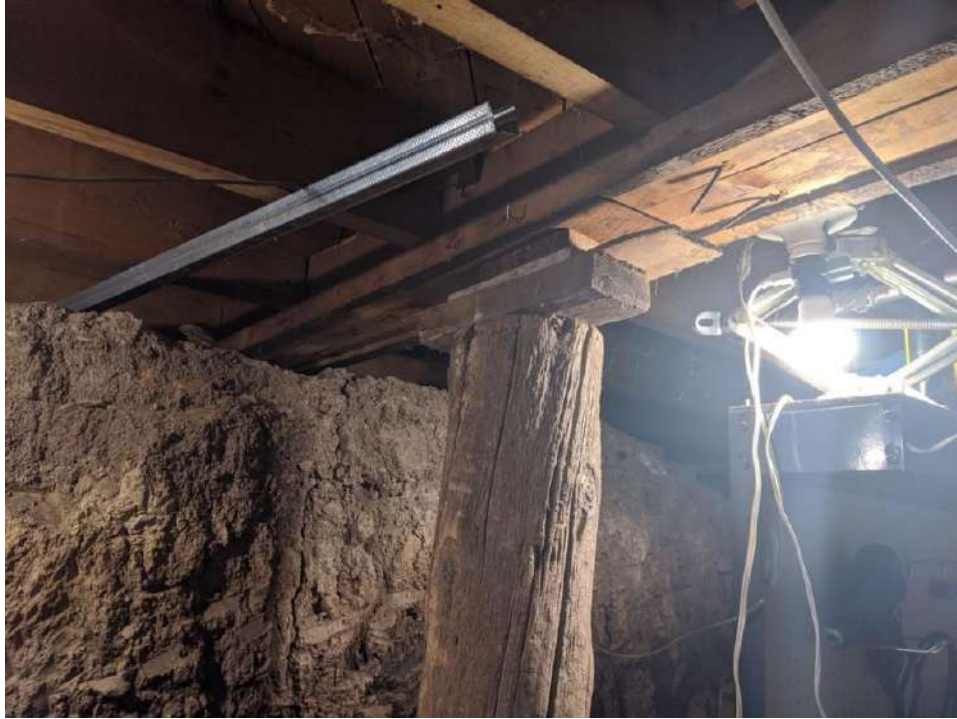
Figure 62: Wood support column in basement
