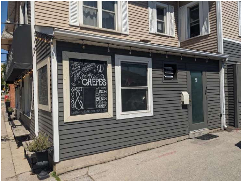
Figure 41: Entrance on the east façade of 93 Bronte Road
