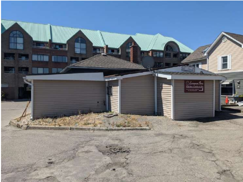
Figure 22: North façade of 87 Bronte Road
