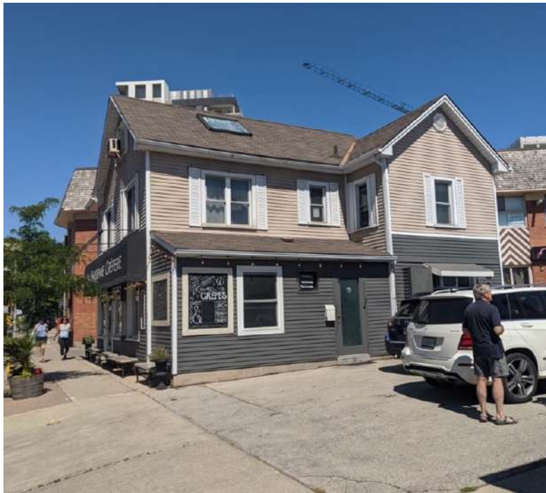
Figure 37: North and east façades of 93 Bronte Road
