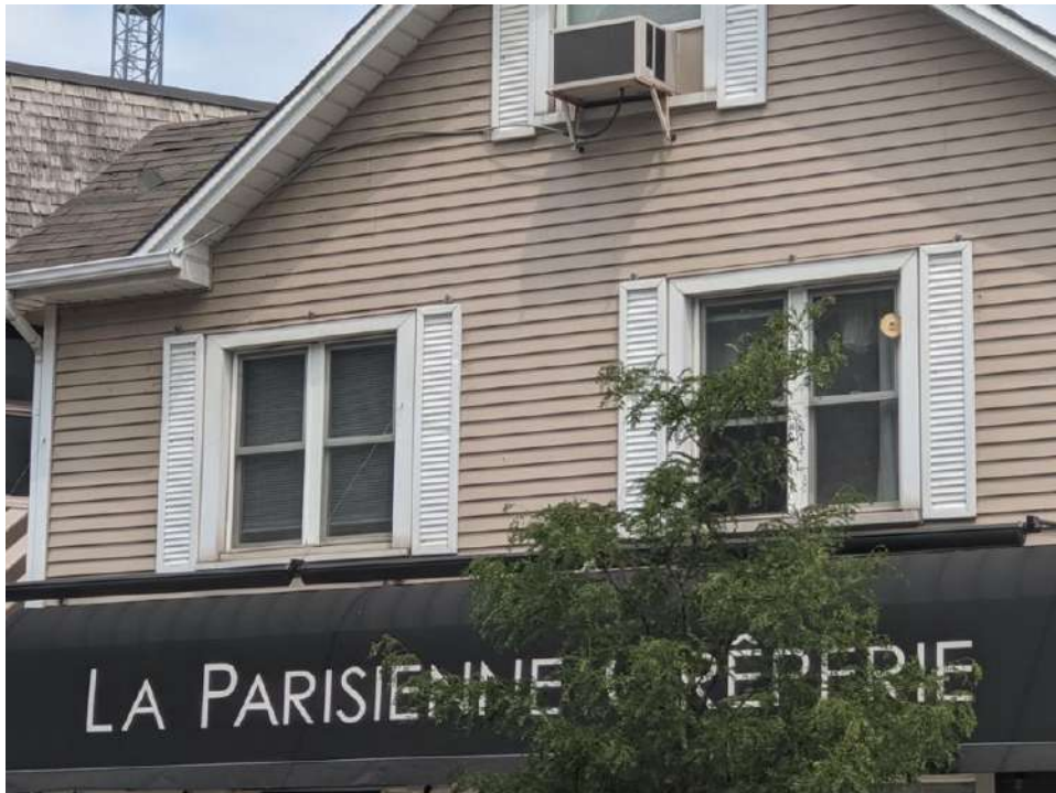
Figure 39: South façade one-over-one vinyl windows
