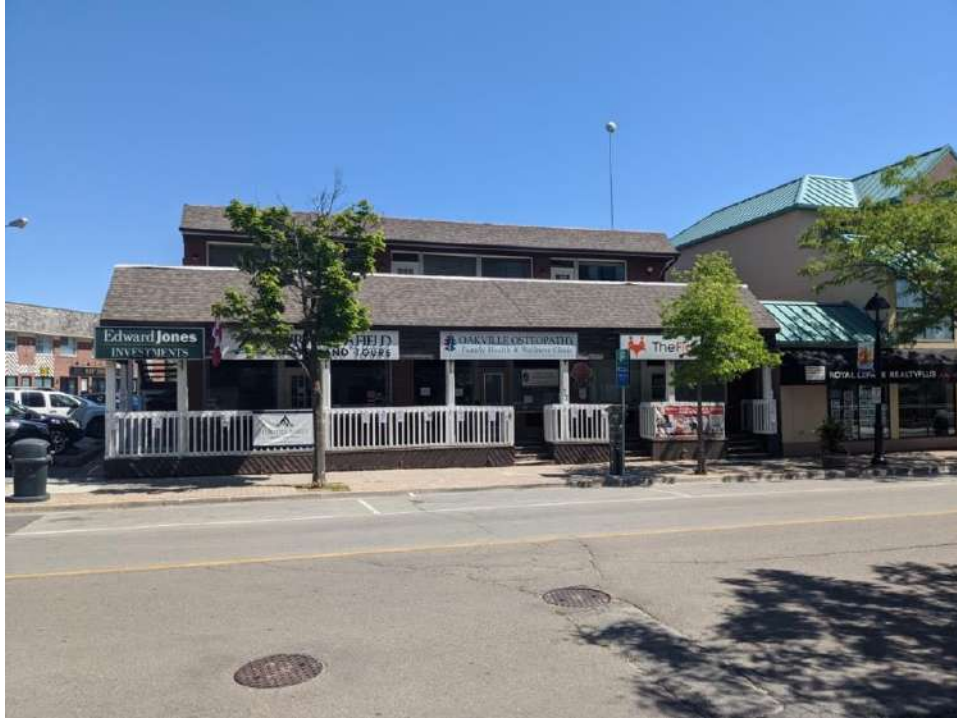
Figure 14: South façade of 77 Bronte Road
