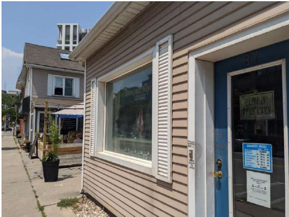
Figure 26: South façade entrance and shopfront window
