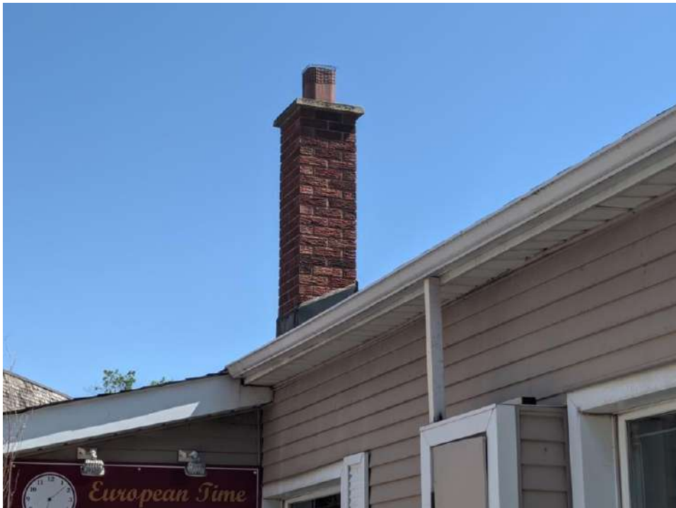
Figure 24: Single brick chimney at 87 Bronte Road
