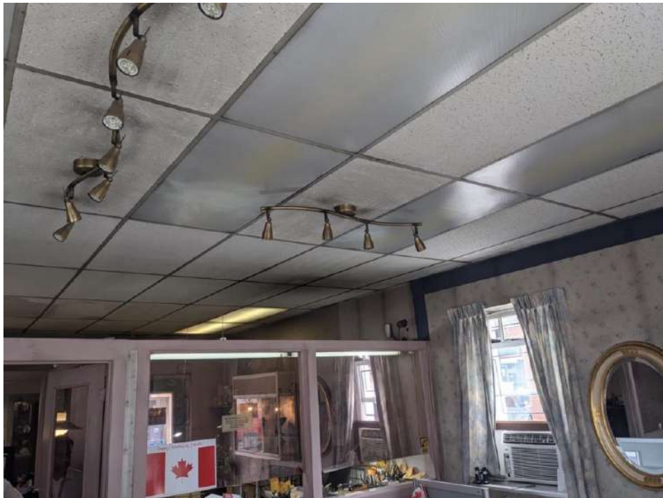
Figure 29: Drop tile ceiling and fluorescent lighting in the jewelry shop
