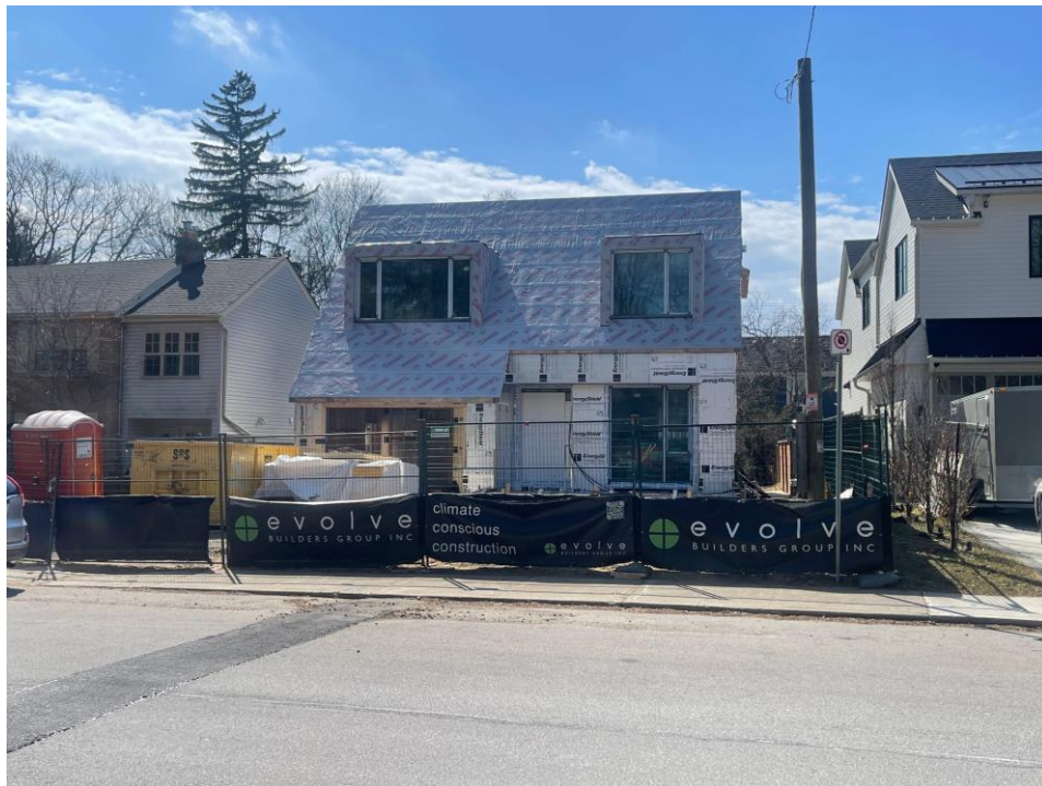
Figure 13 – 302 Douglas Avenue (under construction)
