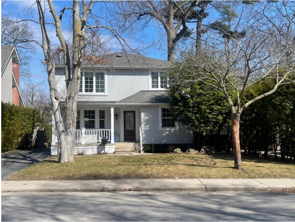
Figure 6 – Street View of Adjacent Property to North (347 Douglas Avenue)
