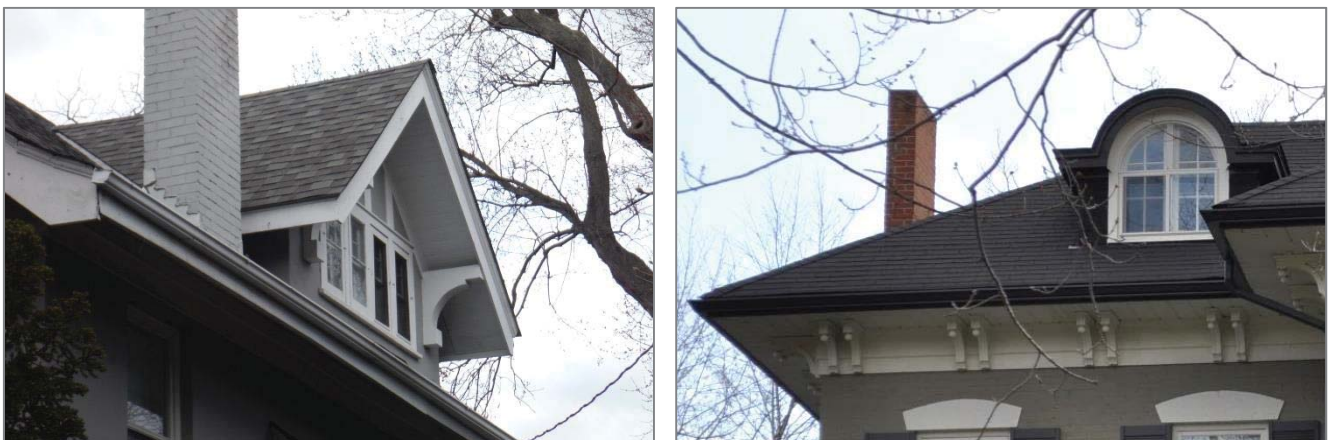
Figure 4: Dormers on 80 Second St. (left), and 72 First St. (right).
