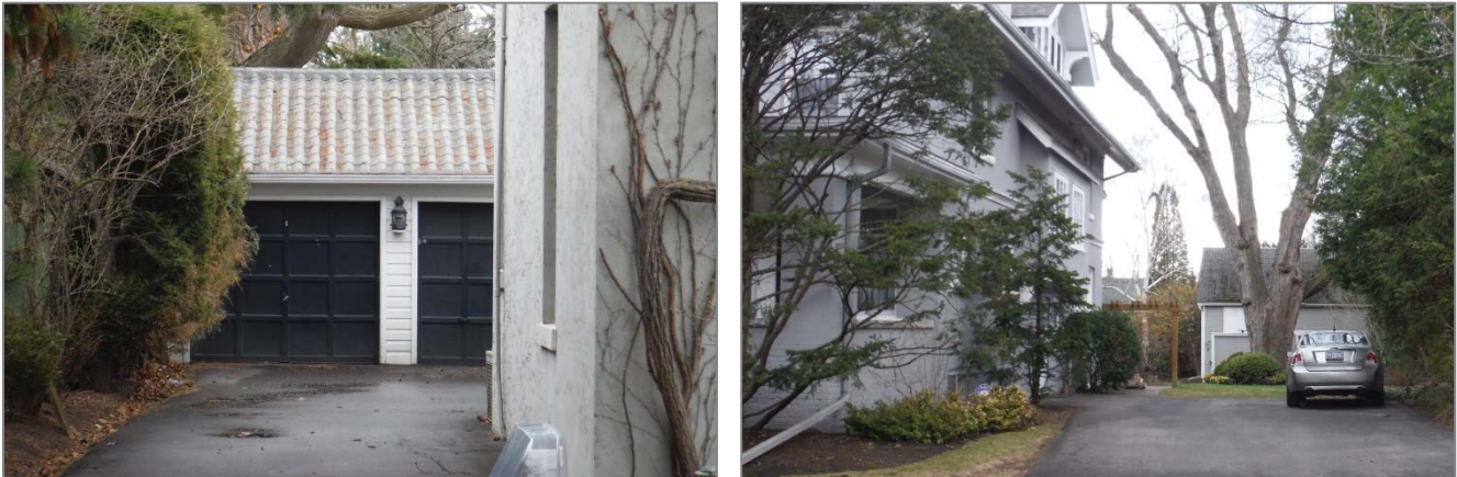
Figure 11: Historic garages at 75 Second St. (left); and 80 Second St. (right).
