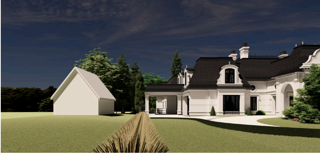
Rendering of proposed open structure carport from Balsam Drive in relation to the neighbouring two-storey garage
