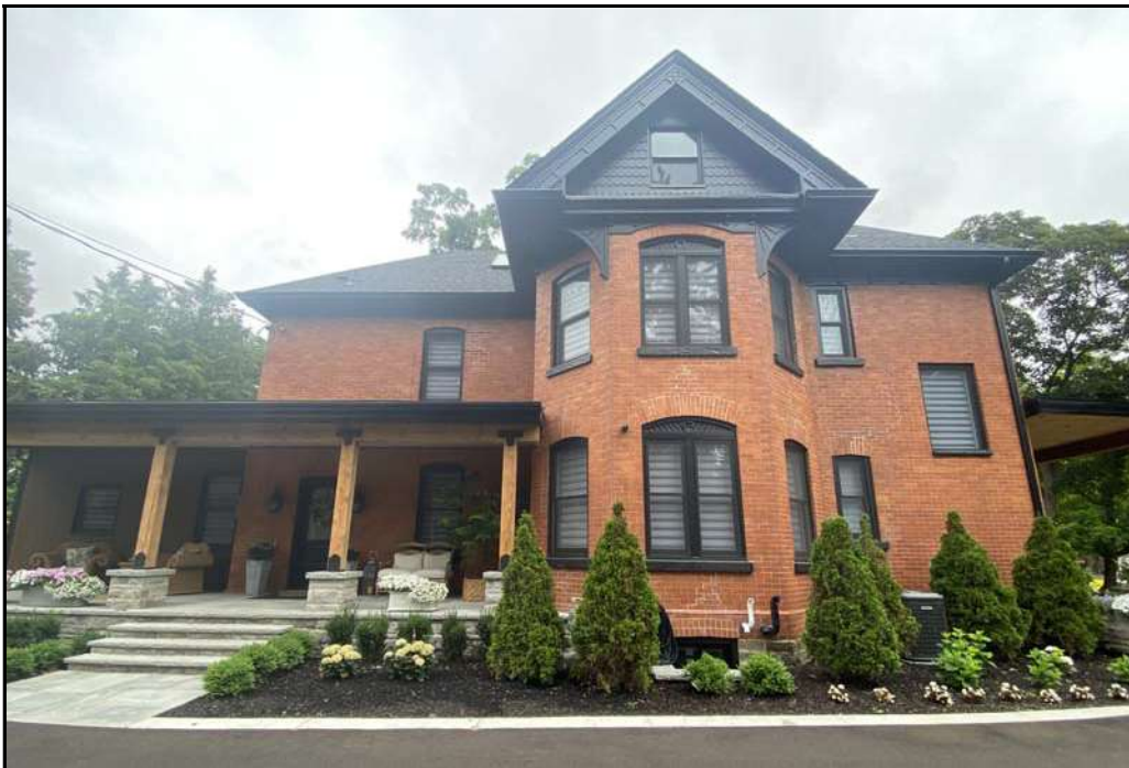
South elevation view showing the new side porch, which extends farther to the west, 2025. Source: Planning Services staff.
