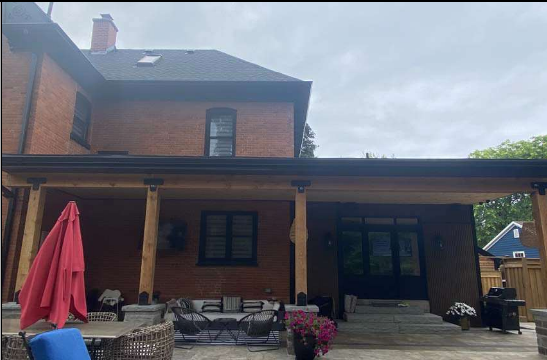
North elevation view showing the new rear covered porch, 2025. Source: Planning Services staff.
