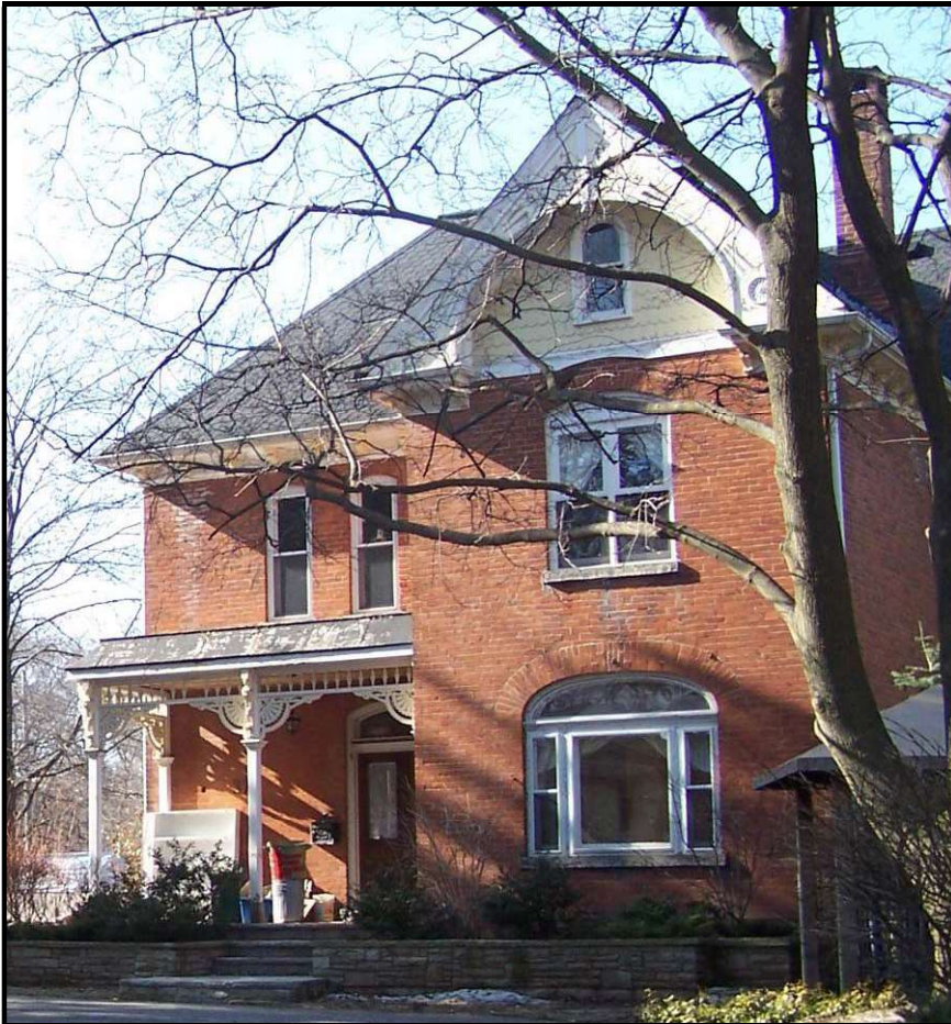
East elevation view showing the front of the house, 2009. Source: Planning Services staff.
