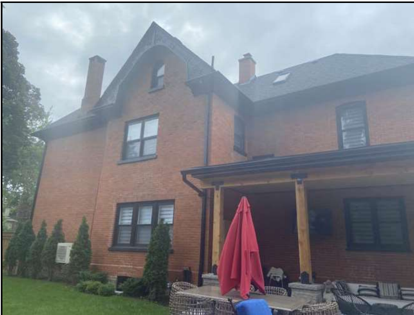
North elevation view showing updates to the original windows, 2025. Source: Planning Services staff.
