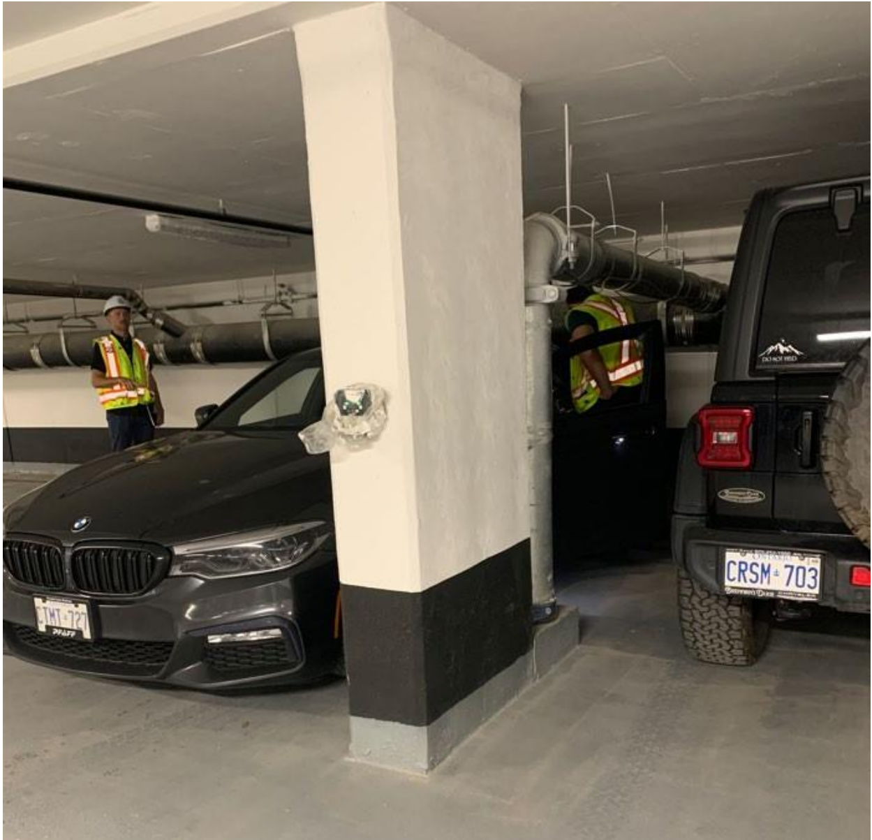
Parking Level A – Space 48 and 49 Vehicle backed into Space 48 with driver side door open to side with pipe obstruction
