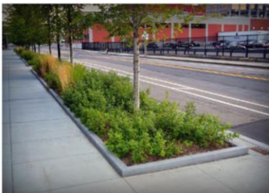
Trees in Open Planter Planter areas to be delineated by 100mm - 150mm concrete curb
