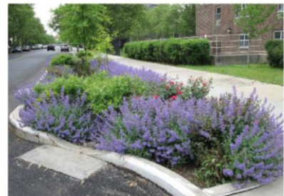
Curb Bump-out Bump-out areas will extend approximately 2.5 metres (the depth of the lay-by parking zone) from the existing curb, at the ends of block.
