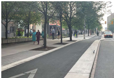
Examples of a raised cycle track between the curb and layby parking
