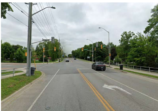
Lakeshore Road West looking east at Dorval Drive
