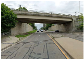
Speers Road looking west at Sheppard Road underpass
