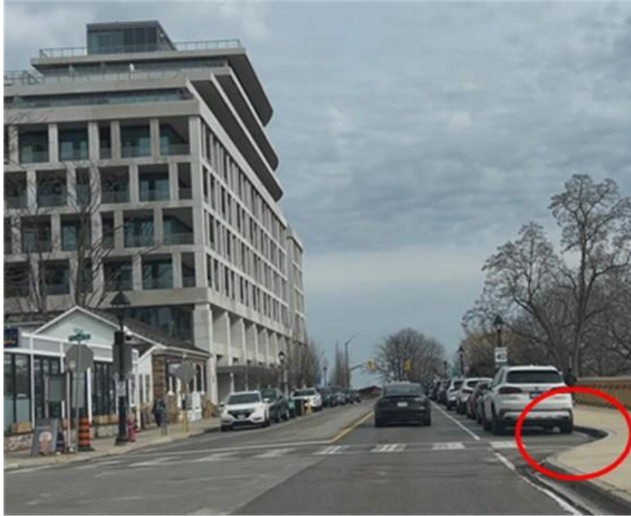
Figure 30: Crosswalk with curb ramp missing
