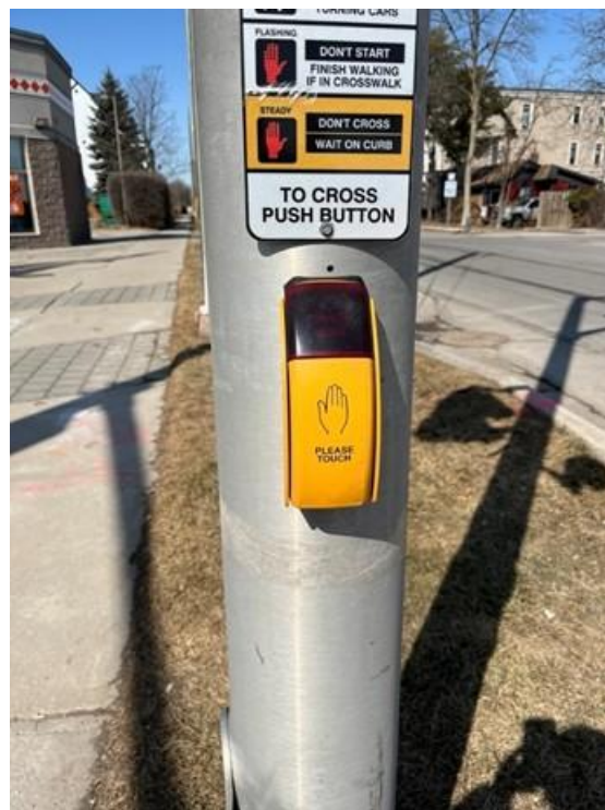
Figure 29: Pushbutton Missing Tactile Directional Arrow
