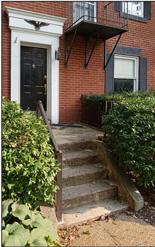
3.2.20: front door and stairs
