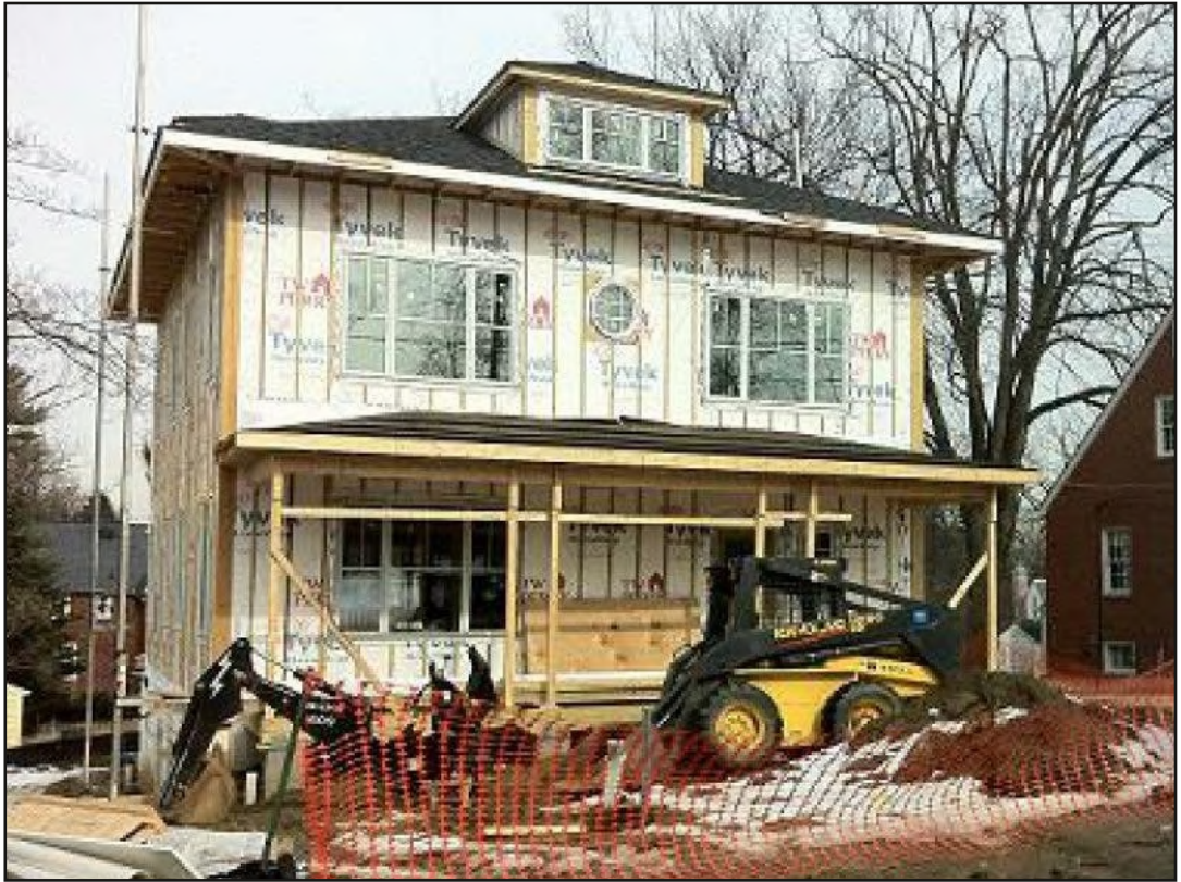
5.2.7a: Bethesda Passive House, under construction (2011)
