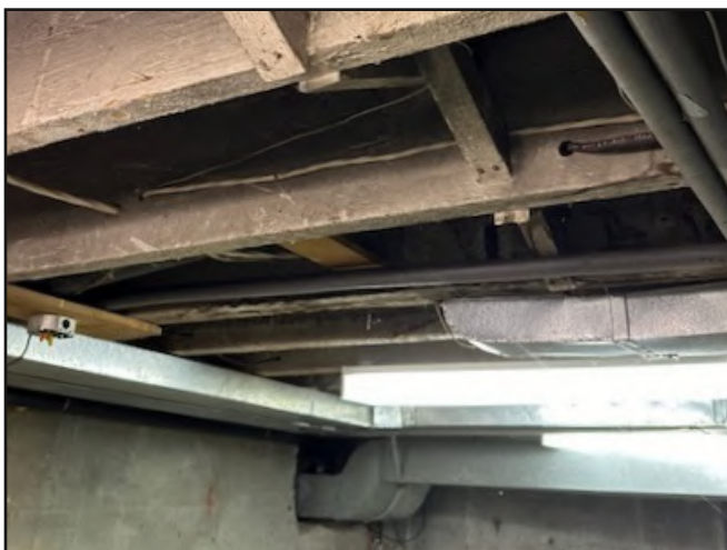
3.2.3d: basement ceiling
