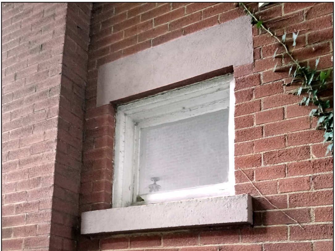
3.2.2l: window with large lintel and apron, west elevation
