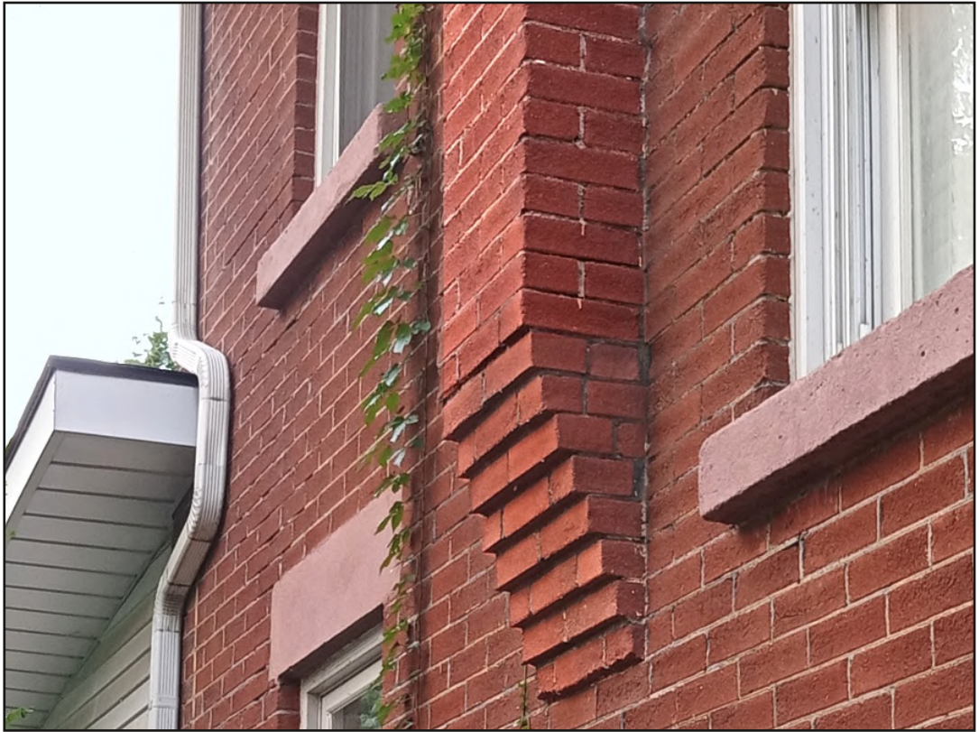
3.2.2i: chimney, east elevation
