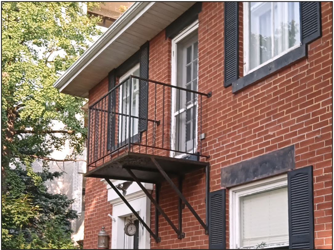
3.2.2m: second-floor balcony, north elevation
