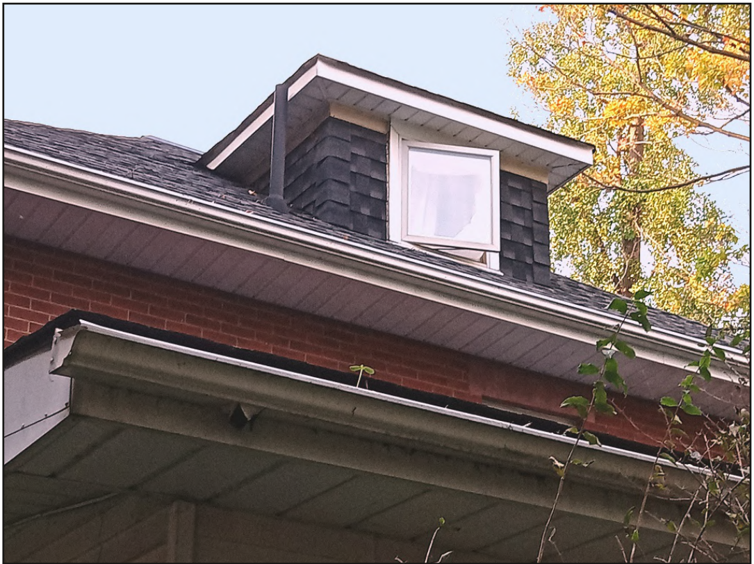
3.2.2n: attic dormer, south elevation
