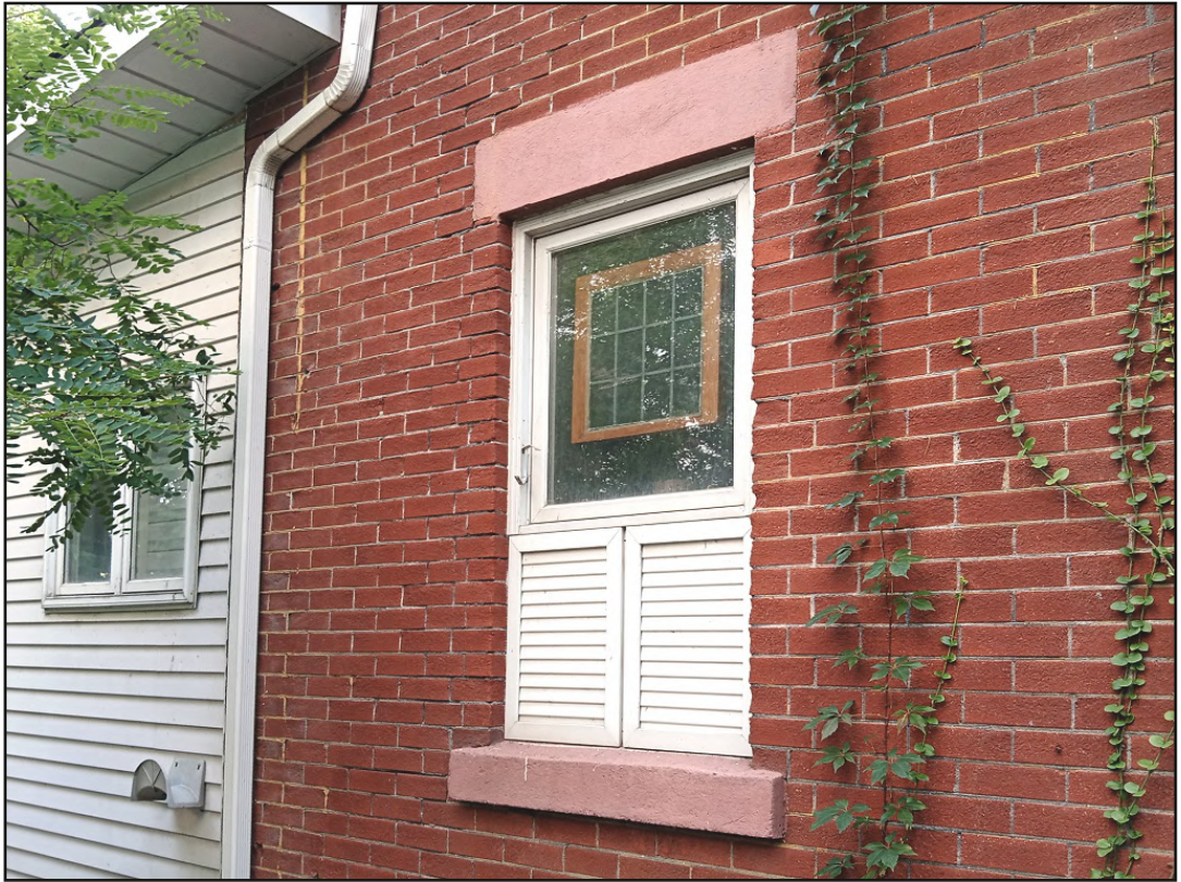
3.2.2g: ground floor window, east elevation
