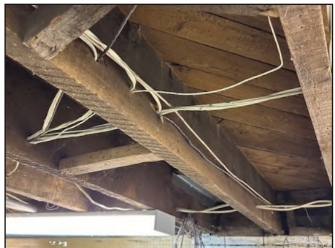
3.2.3e: basement ceiling
