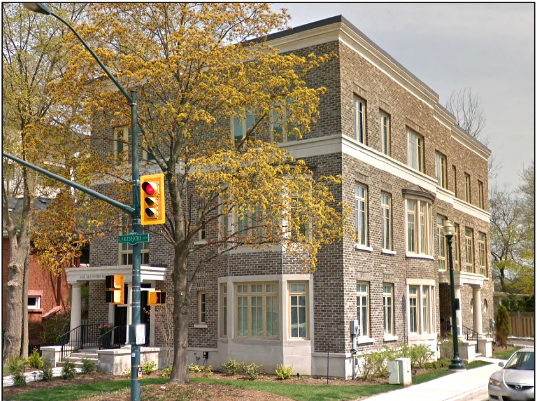
3.2.4b: 360 Lakeshore Road East / 97 Allan Street
