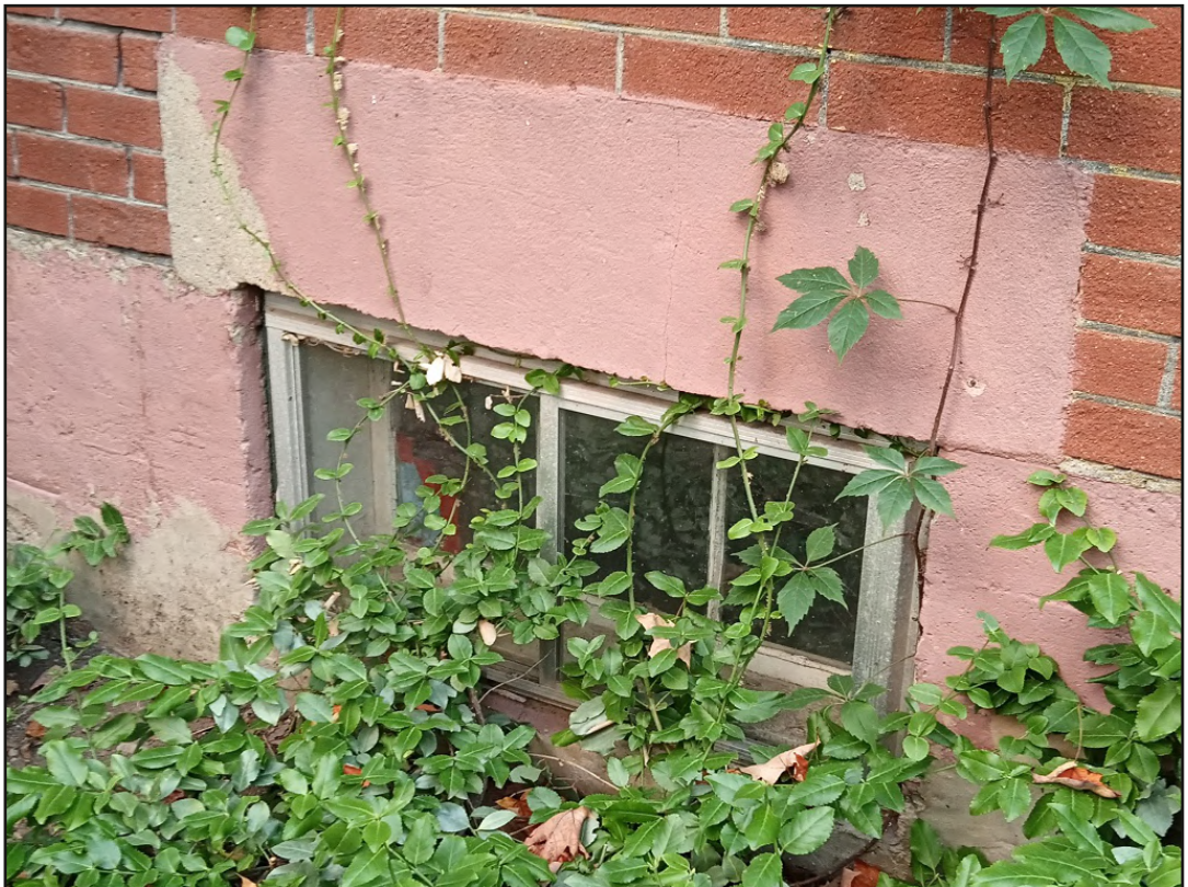
3.2.2h: basement window, east elevation
