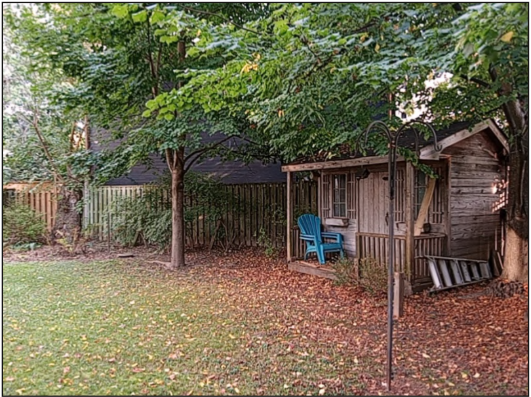
3.2.2e: back yard - looking south east
