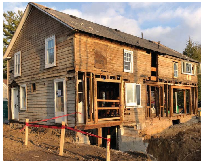
The rear wall of the house after the stucco and rear additions were removed.
