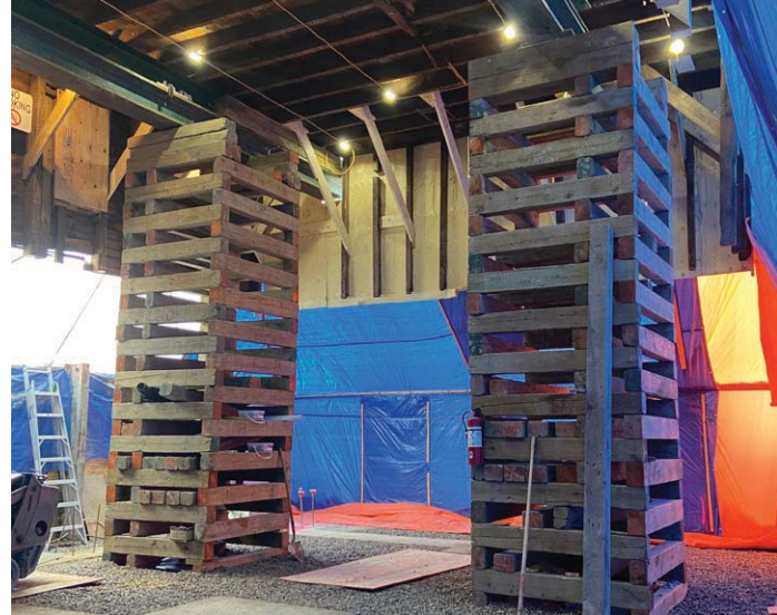
A view underneath the house when it was up on cribs to build a new foundation.
