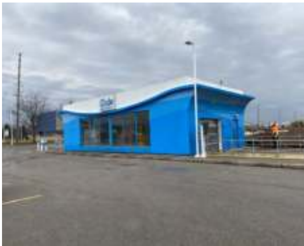
Photo 7 Comments: Entrance and Exit of car wash station. Looking northeast.
