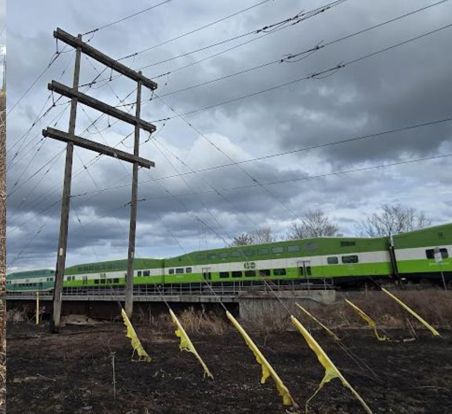
Damage to poles and H-Frame structure at the Bronte Creek Crossing
