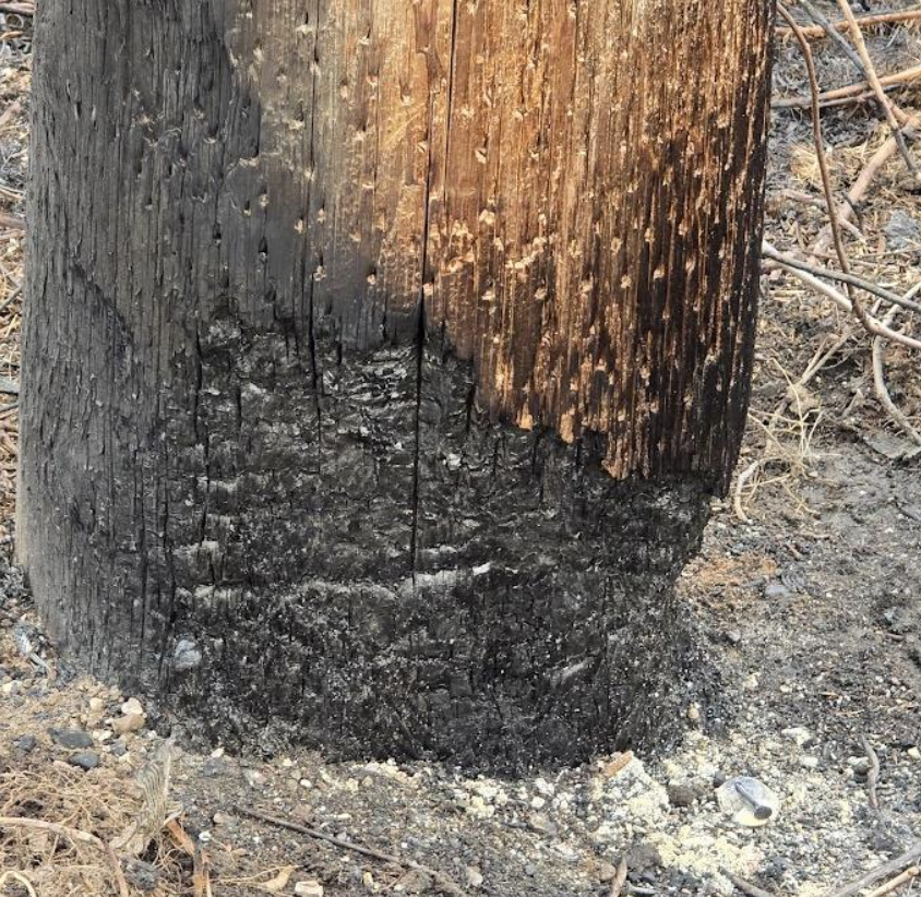
Damage to poles and H-Frame structure at the Bronte Creek Crossing
