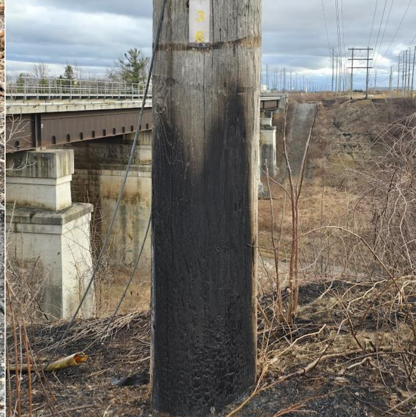
Damage to poles and H-Frame structure at the Bronte Creek Crossing
