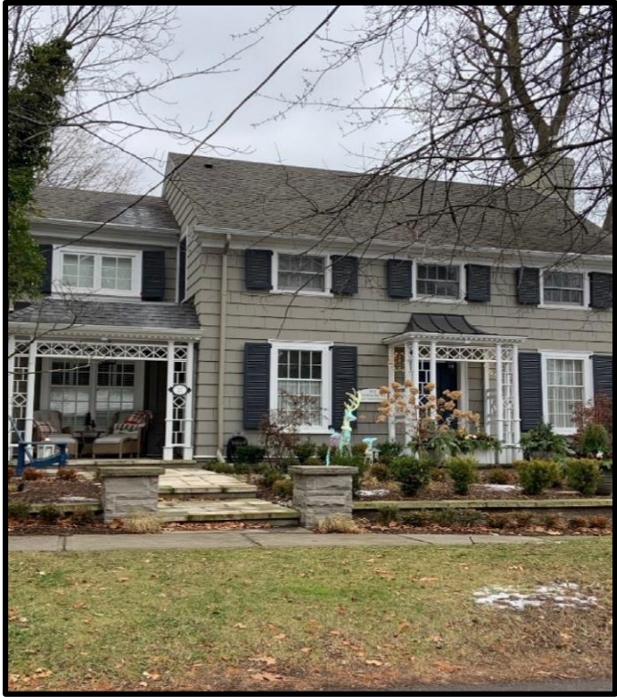
Figure 14: 27 Reynolds Street – Asphalt gable roof with shake cladding
