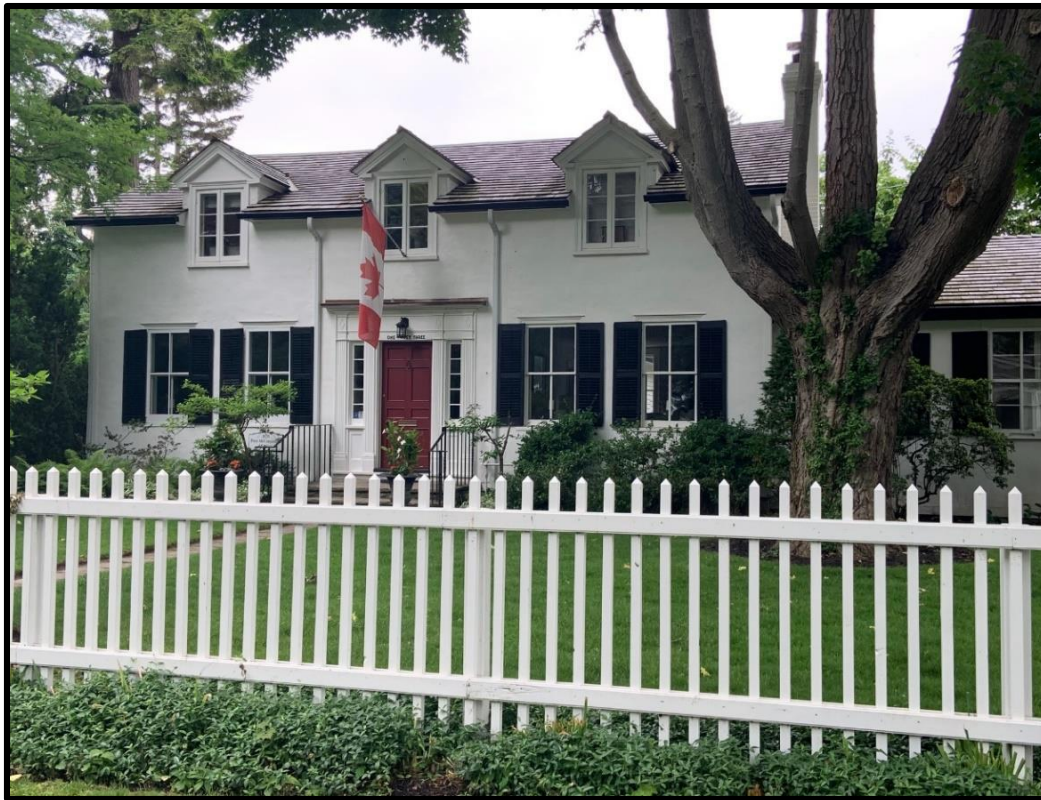
Figure 7: 143 Front Street – Cedar shake gable roof with dormers and stucco cladding
