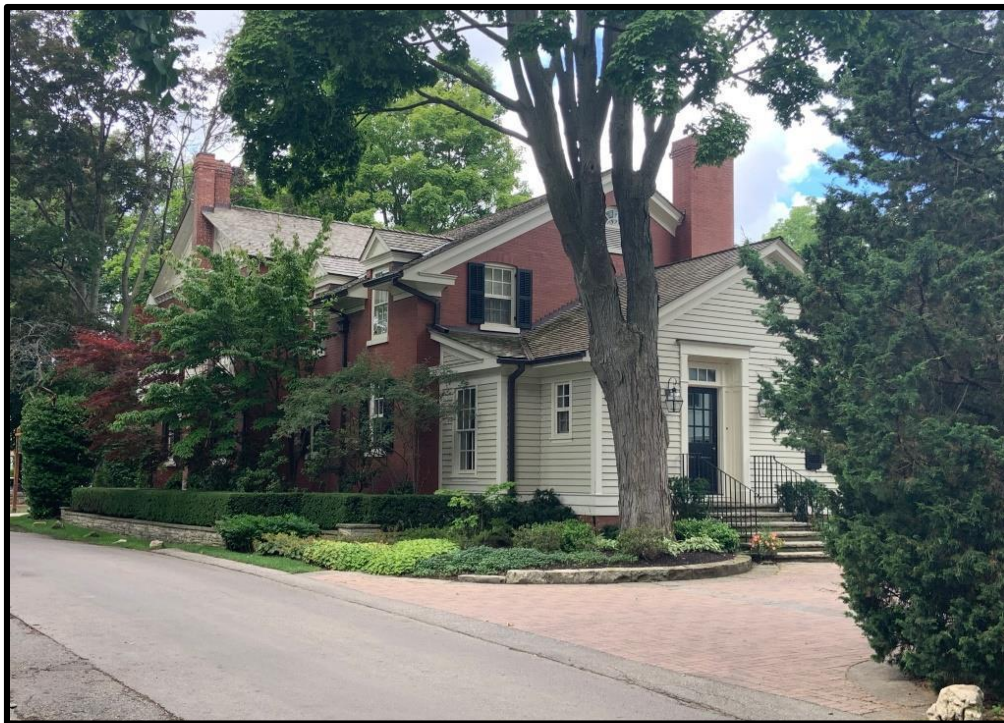
Figure 57: 19 Navy Street – addition to rear and visible from side street; height of addition steps down; consistency in roof form and style of windows/doors and trim; complementary use of materials including brick and horizontal wood cladding
