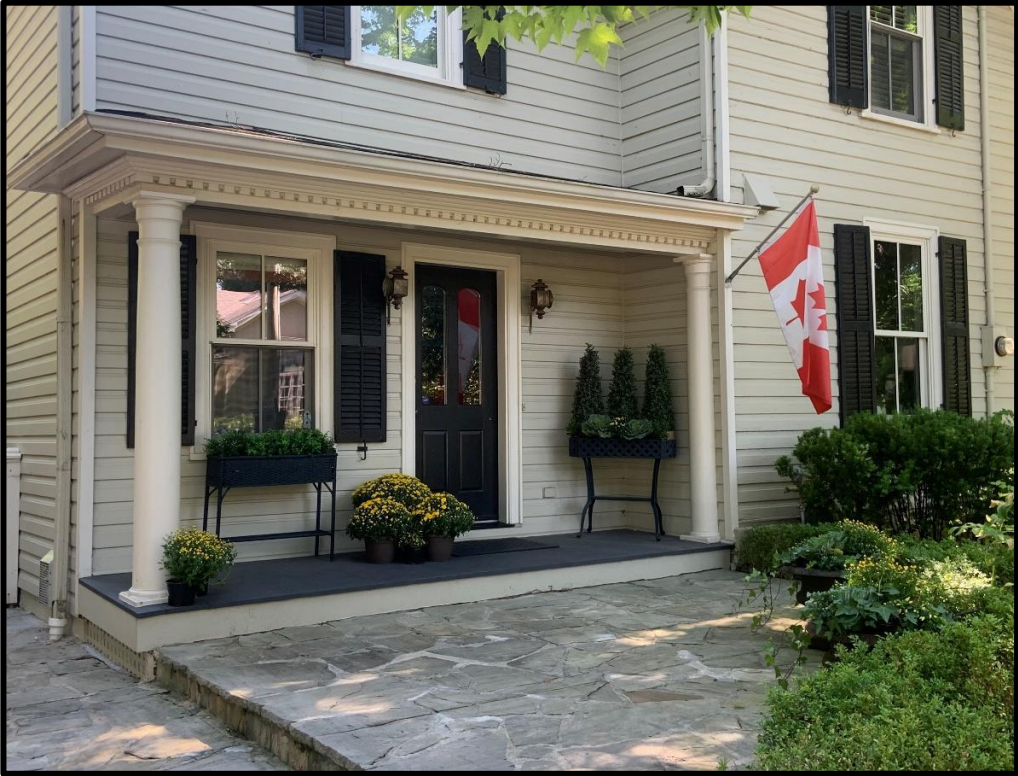
Figure 45: 53 Dunn Street – Example of horizontal wood cladding
