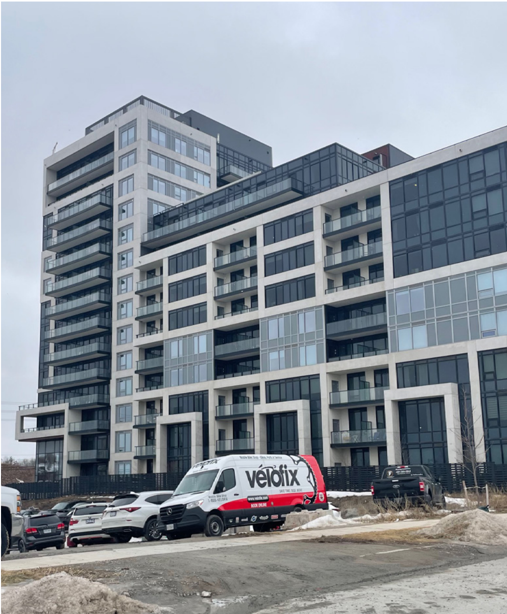
Threshing Mill Blvd 14 Storey
