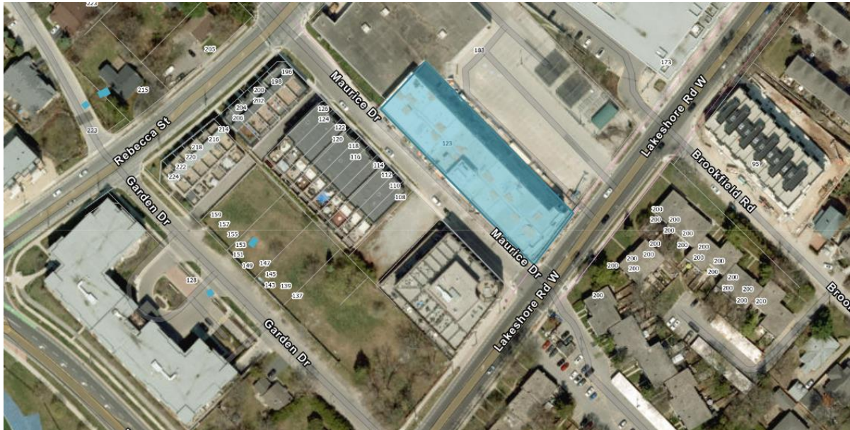
Figure 4 – Aerial view of 123 Maurice Drive
