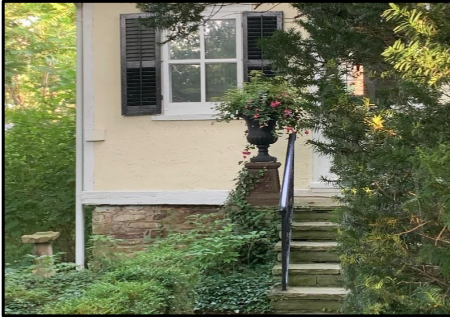
Figure 26: 115 William Street – Lakestone foundation
