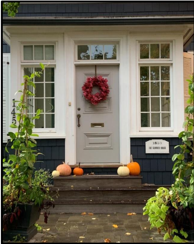
Figure 25: 145 William Street – Main entrance wood door facing street
