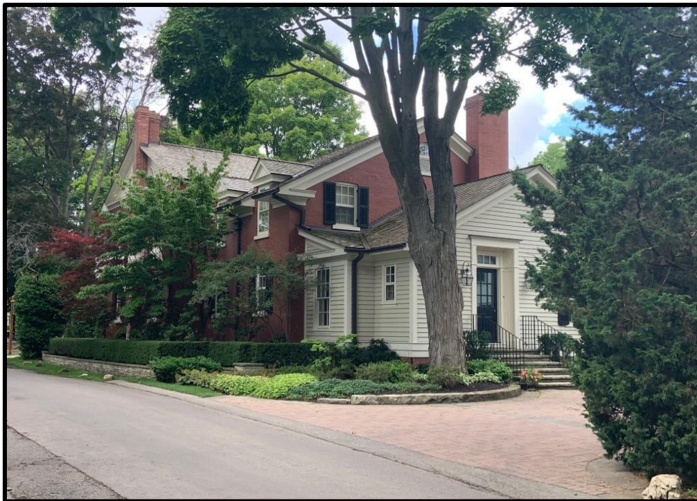
Figure 57: 19 Navy Street – addition to rear and visible from side street; height of addition steps down; consistency in roof form and style of windows/doors and trim; complementary use of materials including brick and horizontal wood cladding
