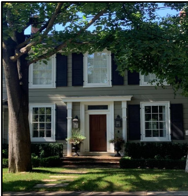
Figure 21: 215 William Street – Wood windows with storm and operating shutters
