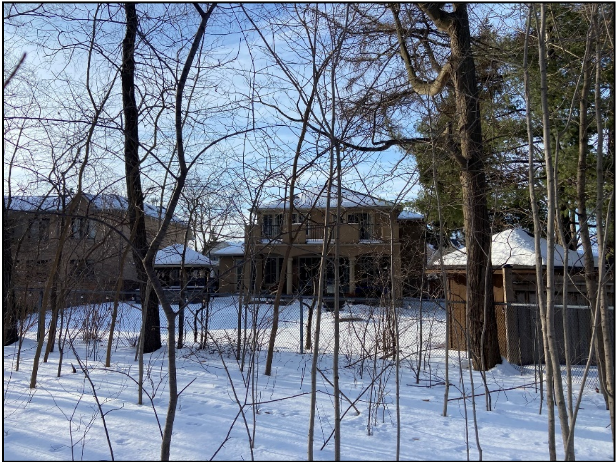
Rear of 1082 Melvin Avenue and existing covered porch taken on February 24, 2025
